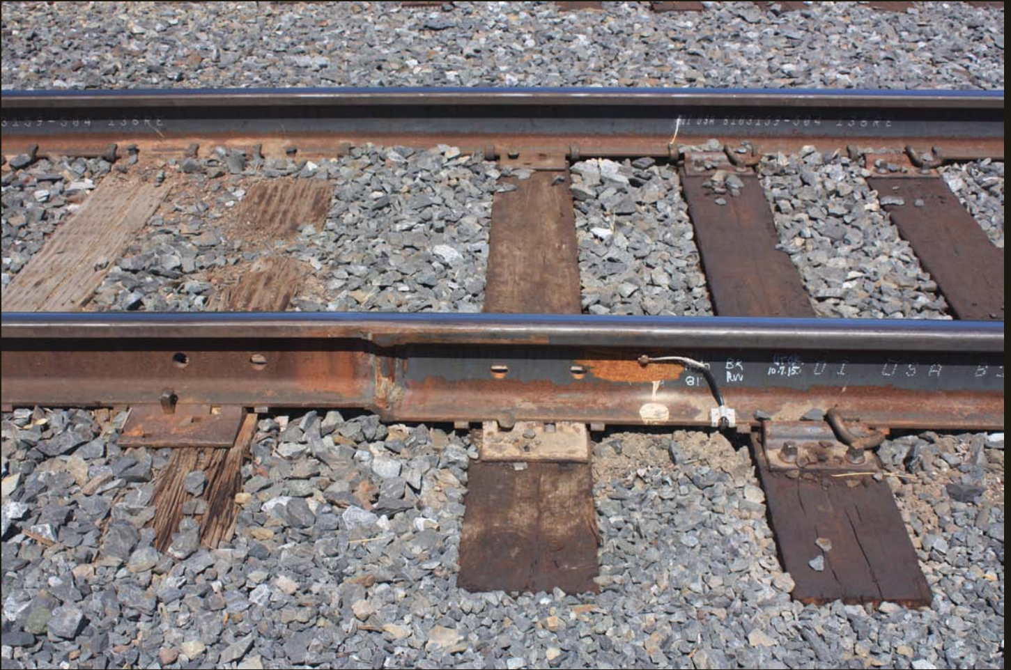
A change in rail weight is welded together at the north end of the Ashland sidings.
