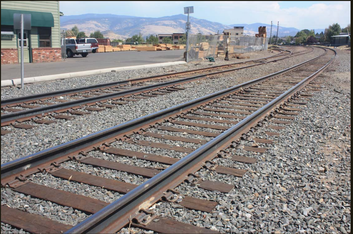
Southward view of the CORP line, one mile northwest of previous location. This is the north end of the Ashland sidings, where four tracks converge to two tracks. The Ashland yard represents the meeting place of the C&O and O&C in 1887, fulfilling the mandate of the 1866 law, so this is the south end of the O&C.
