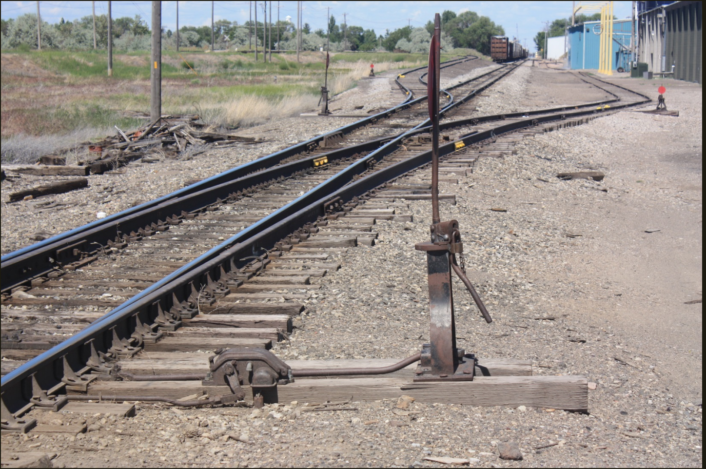
Northeastward view of the M&SW (1905), same location as previous. The first split to the left (northwest) is the south branch of the wye for the OSL Wendell Branch (c1912). That track turns due west (left) in the distance.
