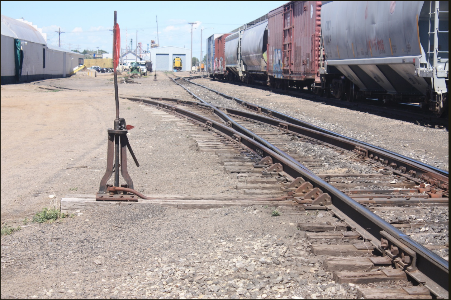
Northeastward view, same location as previous. The bolted track is the north branch of the wye for the OSL Wendell Branch (c1912); the further of the two switches in this view is the crossover from the Wendell Branch wye to the siding with the cars and then the M&SW mainline.
