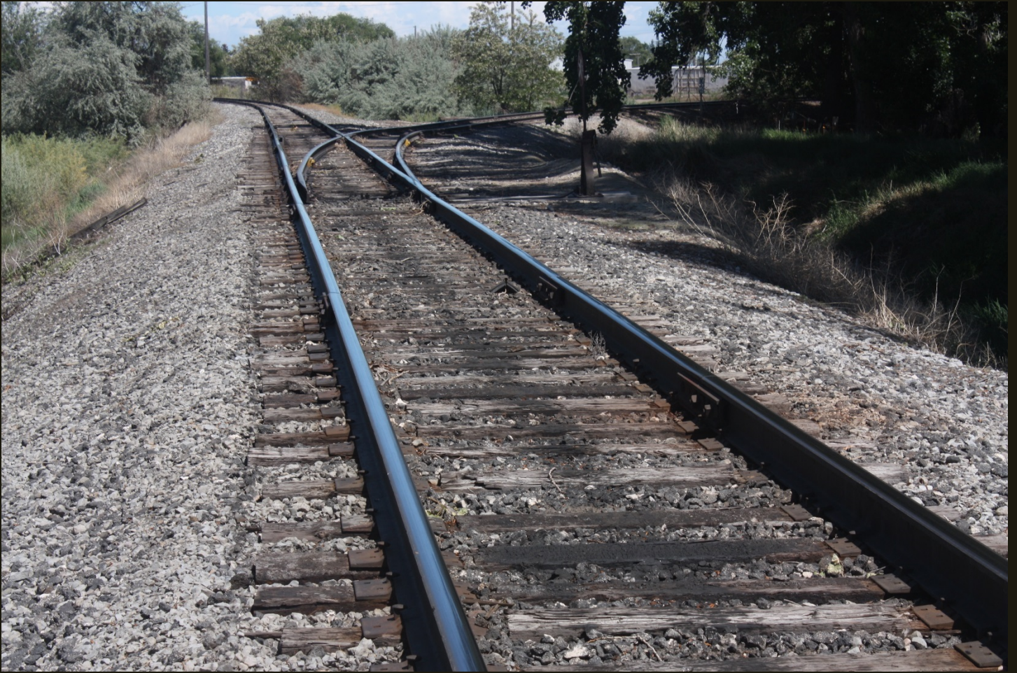
Eastward view of the tip of the wye for the OSL Wendell Branch (c1912). The south branch of the wye is to the right and the north branch is to the left.
