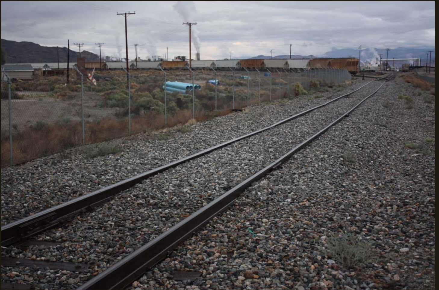
The end of track of the TR is a big loop to turn around trains for the trip back to the start-of-track at Mojave. The switch just to the right of the end of the train splits the track into the two branches of the loop.
