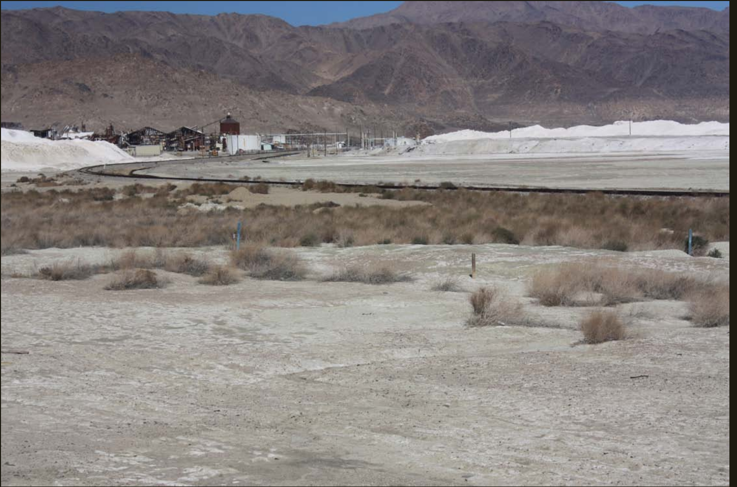
Northward view of the Trona Railway at Westend, the southernmost processing plant, 5 miles south of the end of track at Trona.
