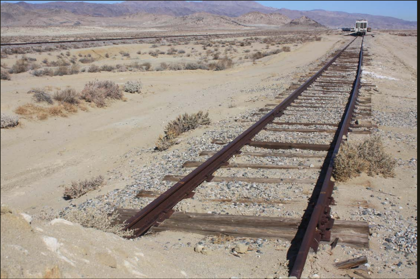
Same hoppers as above, showing the end of the siding and the main line to the left.
