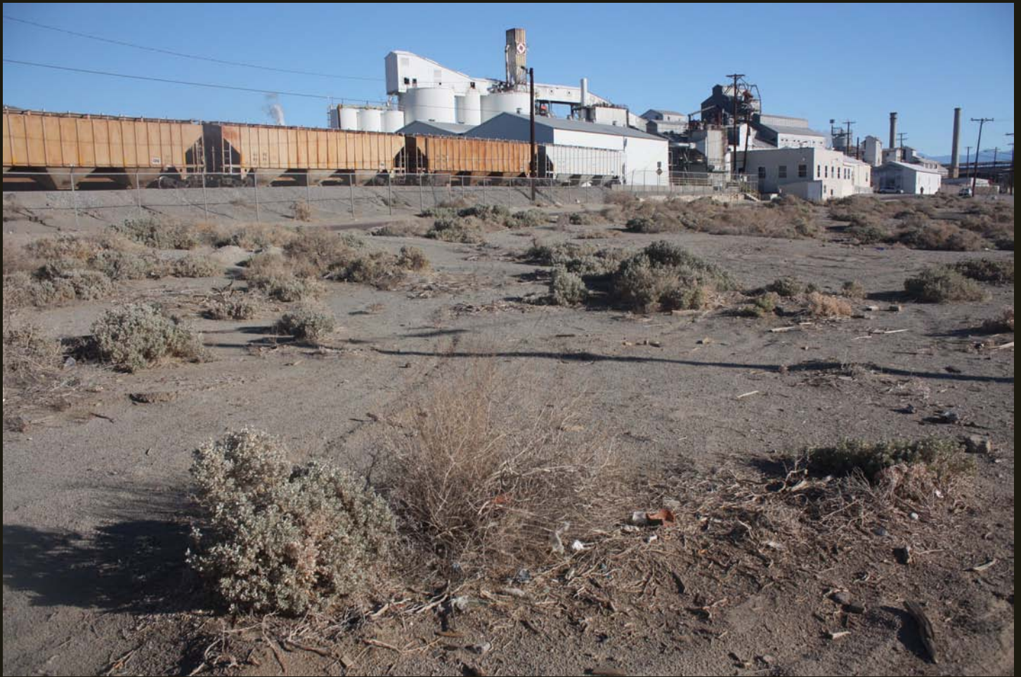
A minerals processing plant along the Trona Railway in Trona.
