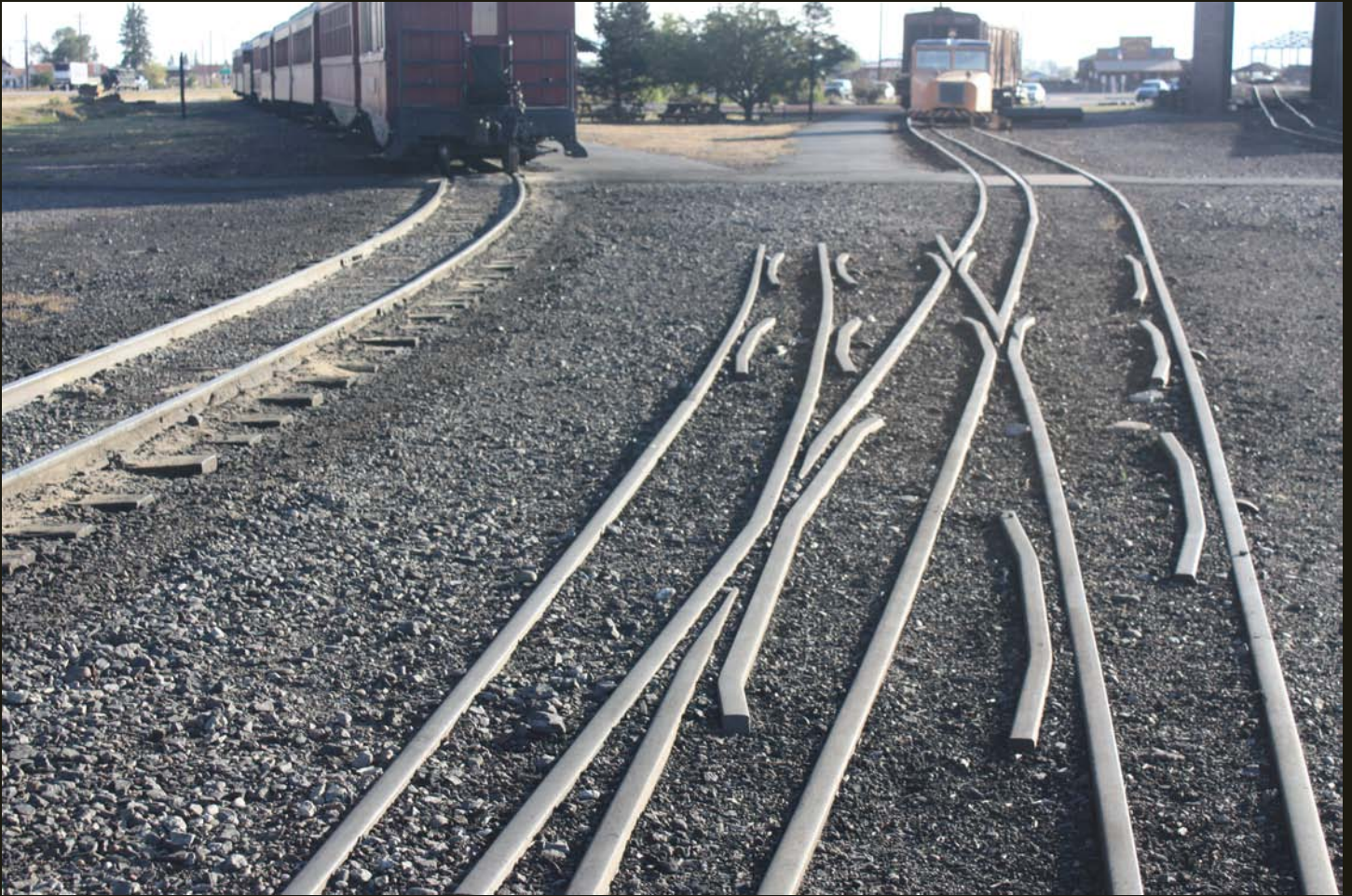
A third rail makes switches a lot more complicated. Note the narrow gauge track on the left.
