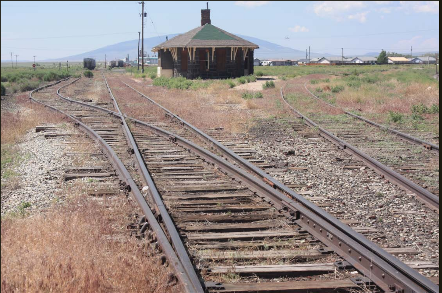
Southward view of the Antonito Depot. The line that goes straight south (to the left of the depot) is the D&RG Chili Line and the line that goes east (to the right of the depot) is the continuation of the San Juan Extension. The next photo is down the line to the left (Chili Line).
