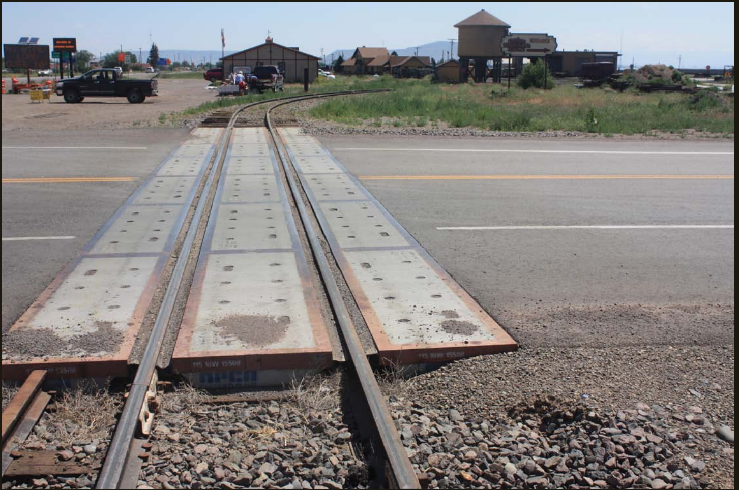
The west end of the C&T yard, facing northeast toward the yard. Note the rusty third (standard gauge) rail in the left foreground. The dual gauge track is on the original narrow- then dual-gauge grade and continued straight through the location of the person, truck, and building, and aligns exactly with the standard gauge track in a previous photo. The curve to the right is the C&T grade and is the general location of an old switch to the D&RG yard.
