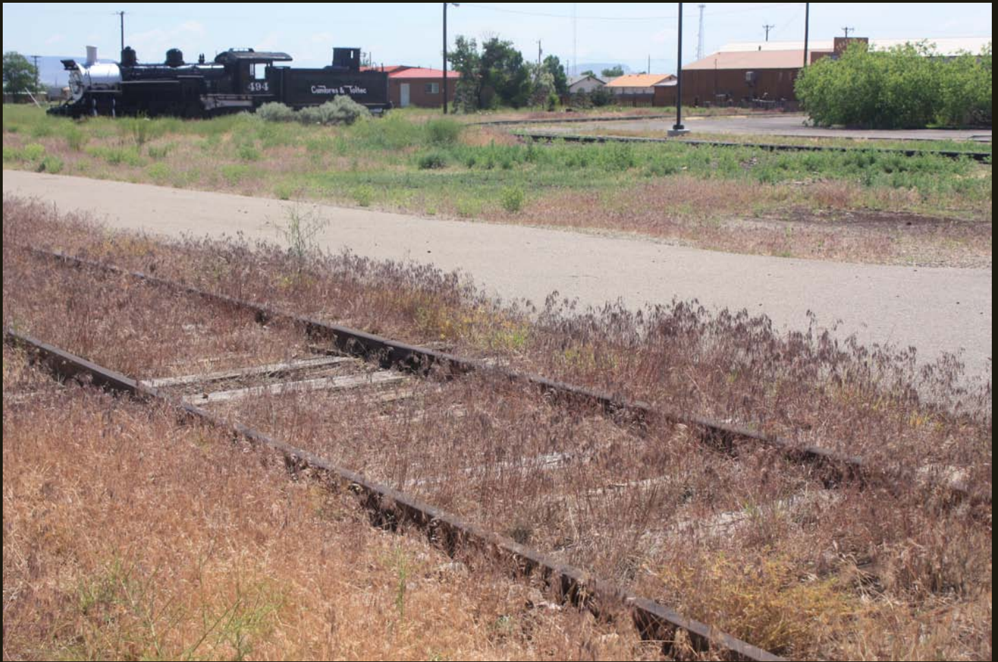
A few steps southwest of the previous photo, with the standard gauge tracks in the foreground and the same narrow gauge locomotive as in the previous photo. The curved track in the upper right was built after 1970 and is the circular turnaround that marks the east end of the narrow gauge C&T tourist railroad. The standard gauge track in the foreground is on the original 1880 grade.
