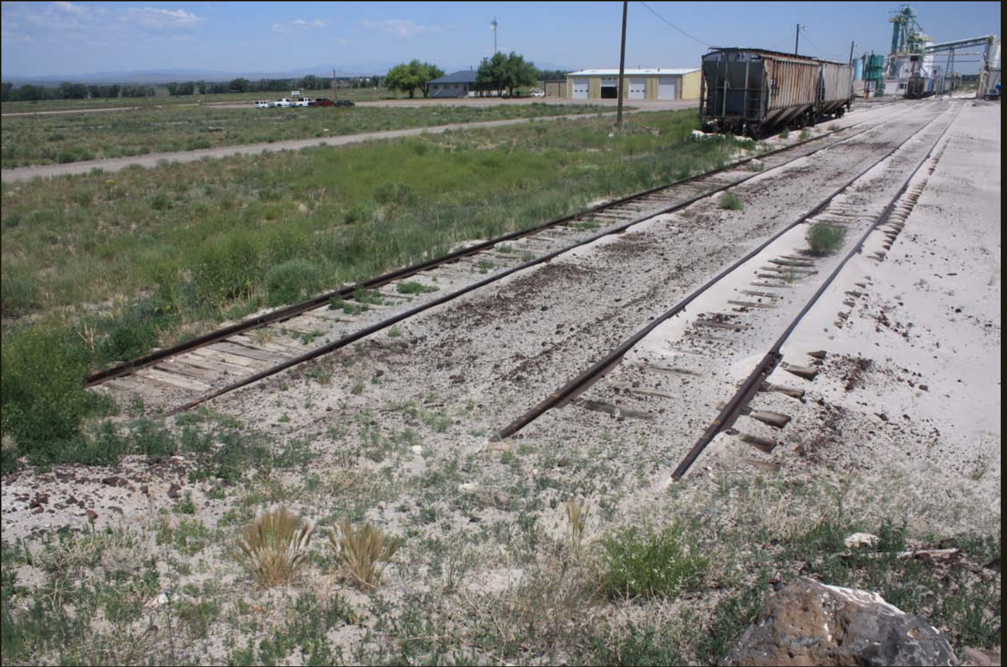
Northward view of the same chemical plant as in the previous photo, showing the southern end of the part of the Chili Line that the D&RGW converted to dual gauge in 1901 and to standard gauge in 1970.
