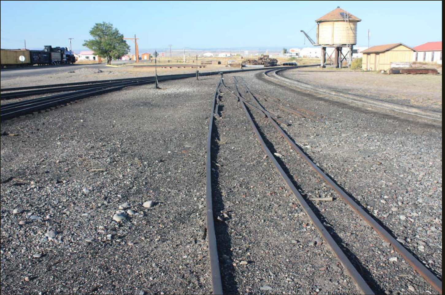
A three-rail (dual gauge) siding and a water tower at the Antonito C&T yard. In the left distance, C&T #484 is moving some cars around the yard.
