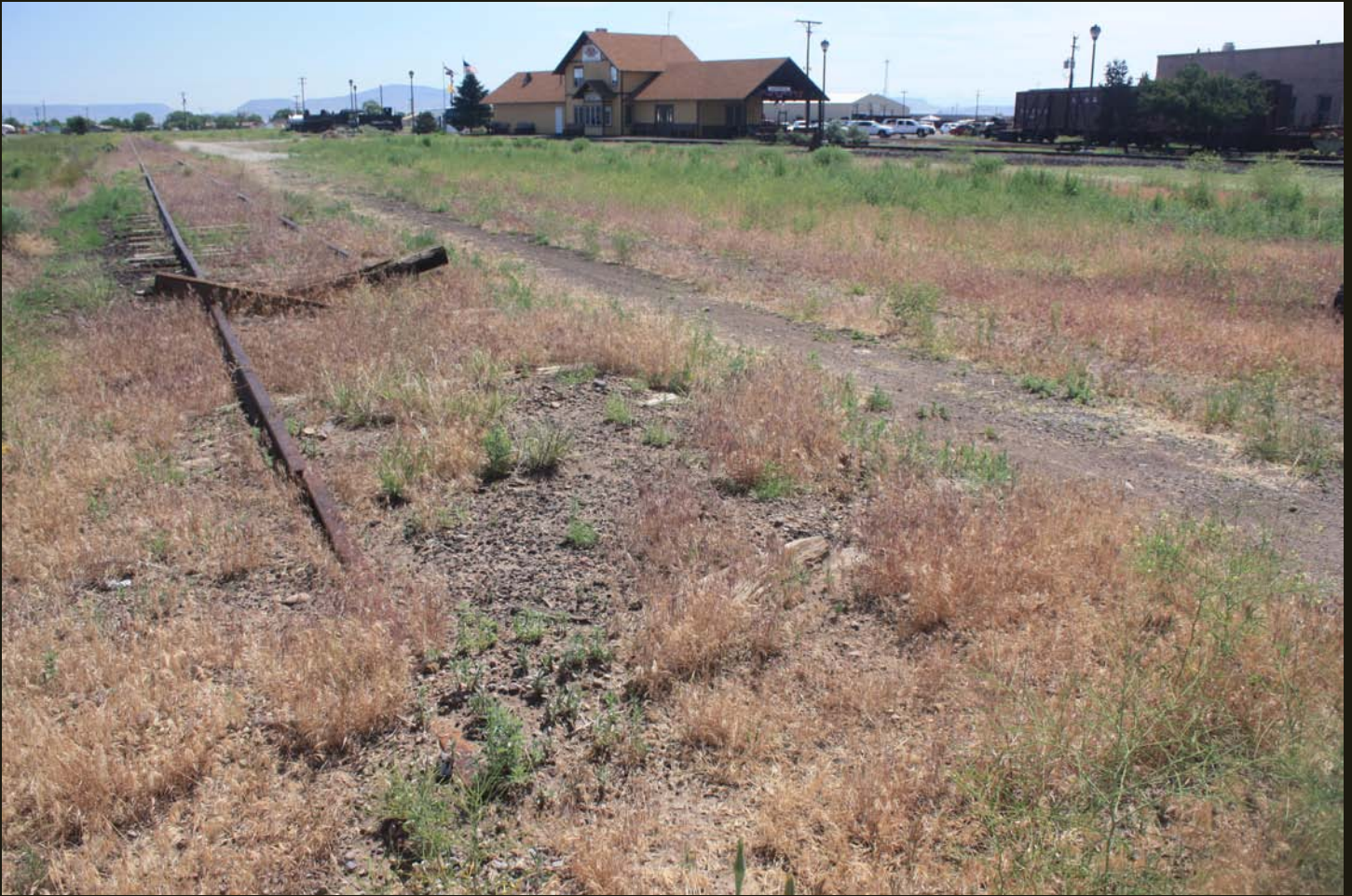
Northeastward view at the end of the standard gauge track, which is on the original narrow gauge grade of the San Juan Extension. About 300 feet behind the viewer (southwest), the C&T re-aligned the narrow gauge line off of this alignment, generally following branches in an old rail yard at this location, and built a new circular turnaround, which passes in front of the C&T Depot in the center distance.
