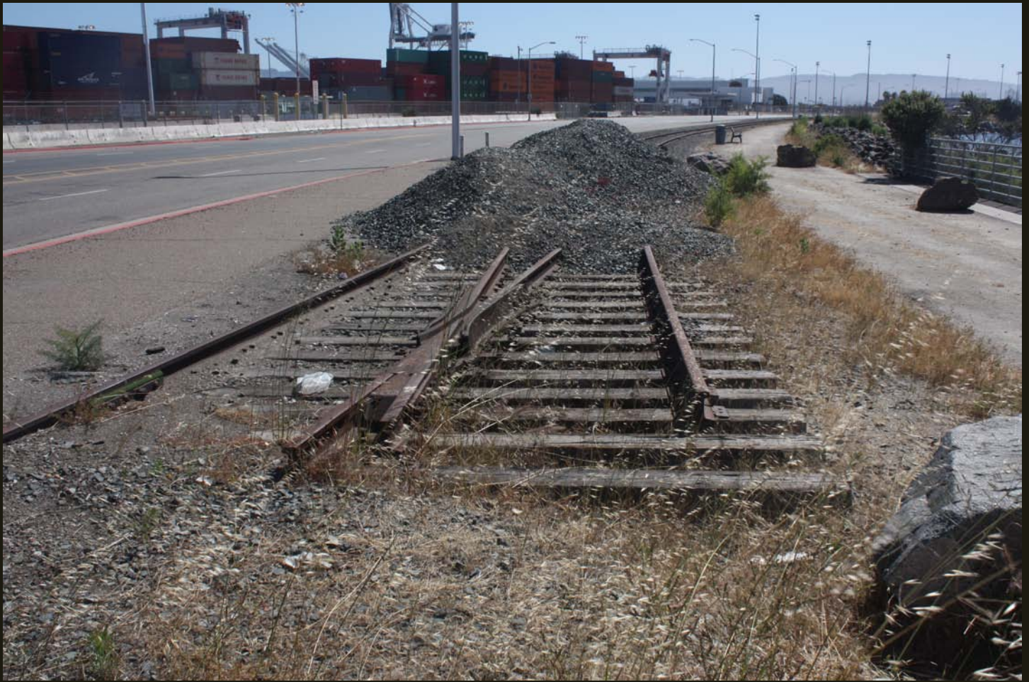
Eastward view of abandon trackage at the westernmost point of land at the Port. These tracks only hint at the history of railroad realignments at the Port of Oakland, especially following the conversion from direct loading of ships, as these bayside tracks attest, to container loading, as the cranes and containers in the distance attest.
