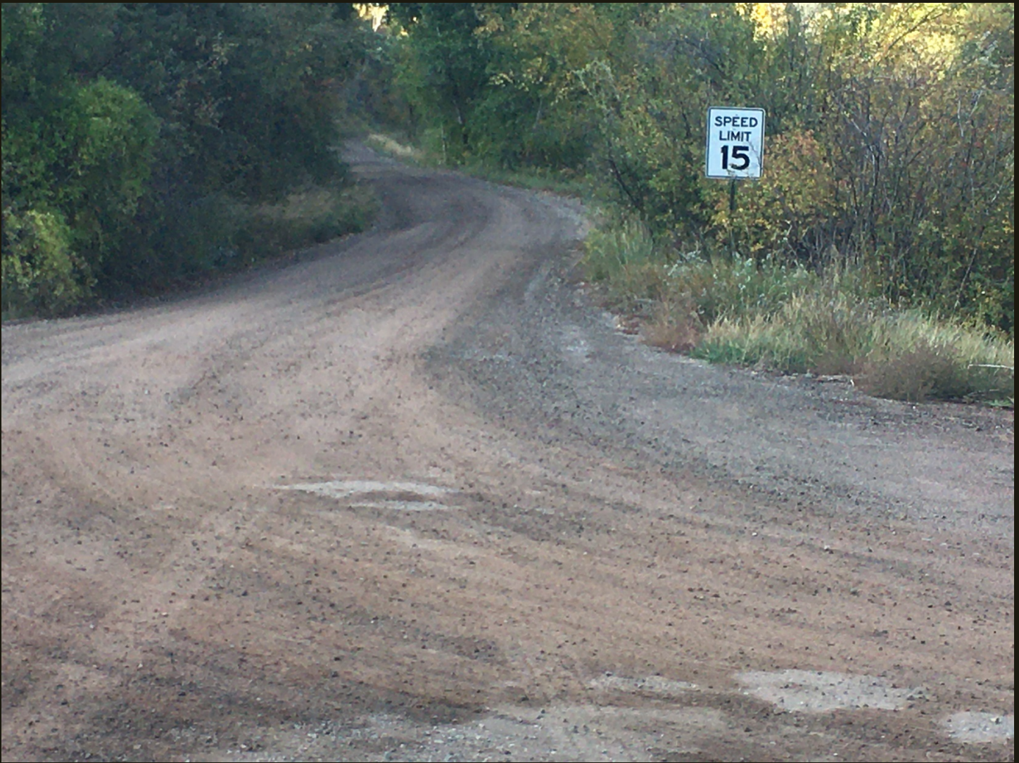
Southward view of the CR Railway (1893n) at the same location as previous. The alignment was regraded to make a road.
