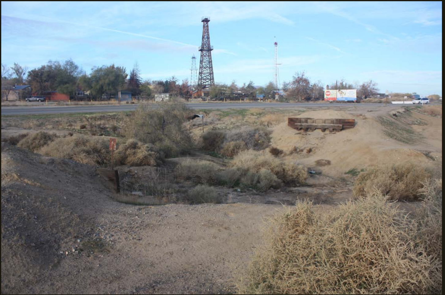
Northwestward view, same location as the previous photo, at the south end of Taft. The old bridge abutments are on the SW Taft Branch, with the fill grade beyond in pretty good shape. The derrick is part of the West Kern Oil Museum.
