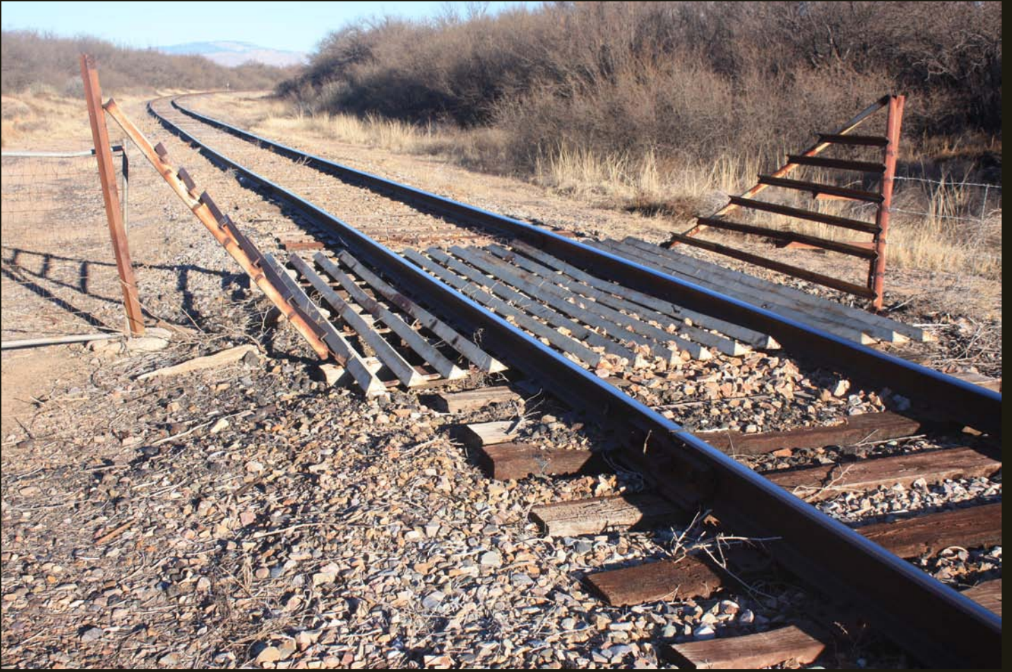
Northwestward view of the A&SE (1894)/EP&SW/SP/SP&SW and cattle guard, 5 miles south of the Benson
