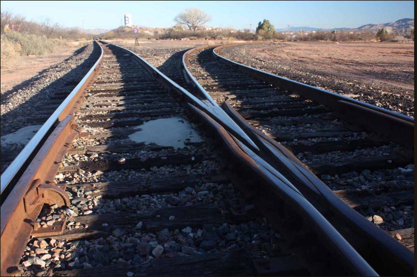
Northwestward view of the tip of the Benson wye. Note the location of the Benson water tower and the tighter curvature of the east (right hand) branch of the wye.
