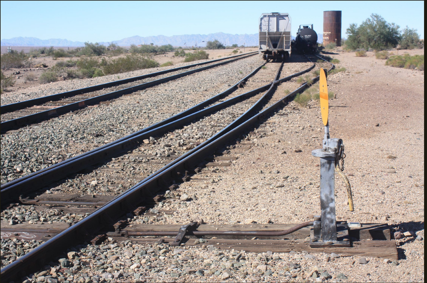
Closer look at the A&C Rice siding, an old water tower is to the right (north) of the tracks. Just out of sight to the left of the track is the siding for the wye junction with the California Southern (1920).
