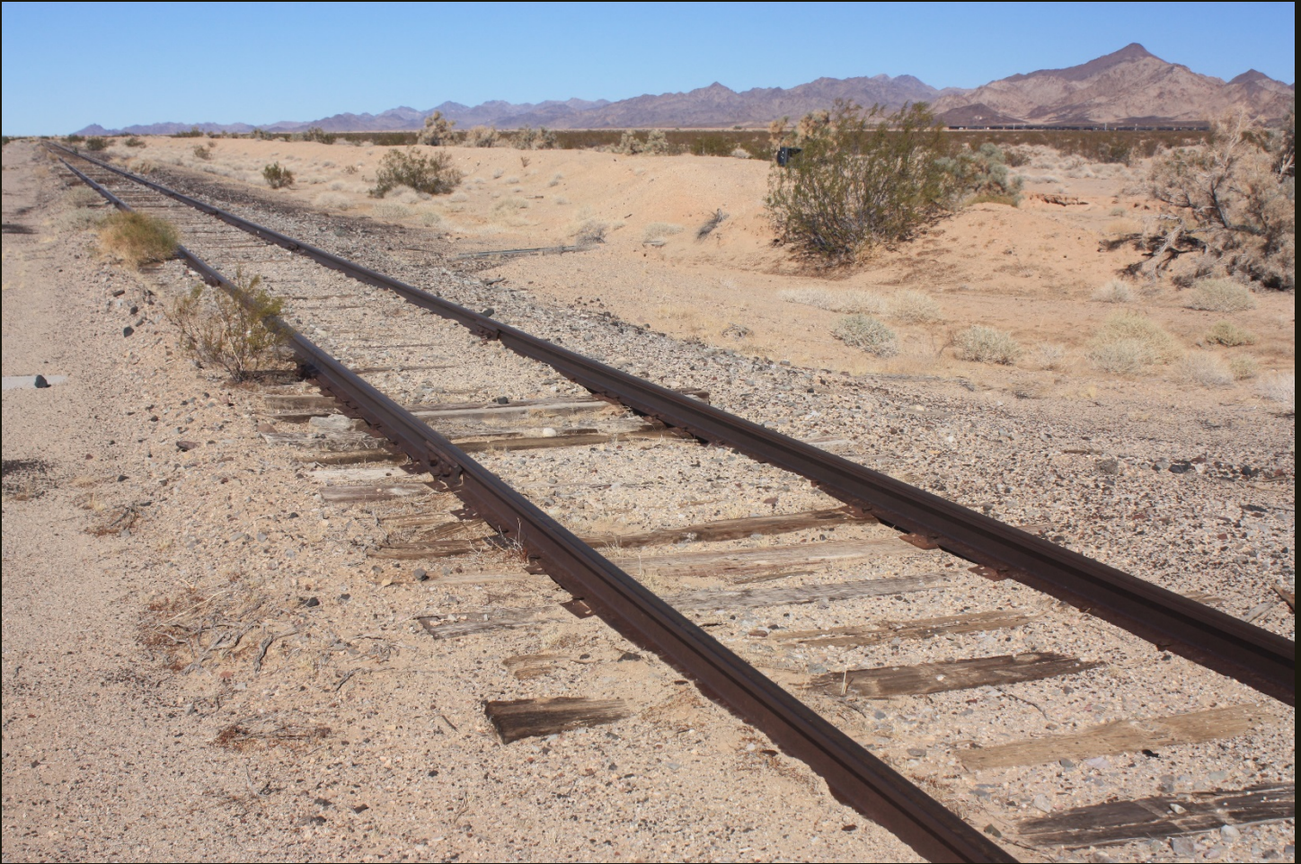
Northward view of CS (1920), 1.8 rail miles from Rice, located where stored cars are visible in the right distance. The tracks run northwest here, then turn through an almost horseshoe bend to eastward, then a 90-degree left to approach the Rice wye on a northward alignment. The sinuous route is apparently to lower the grade on this alluvial slope.
