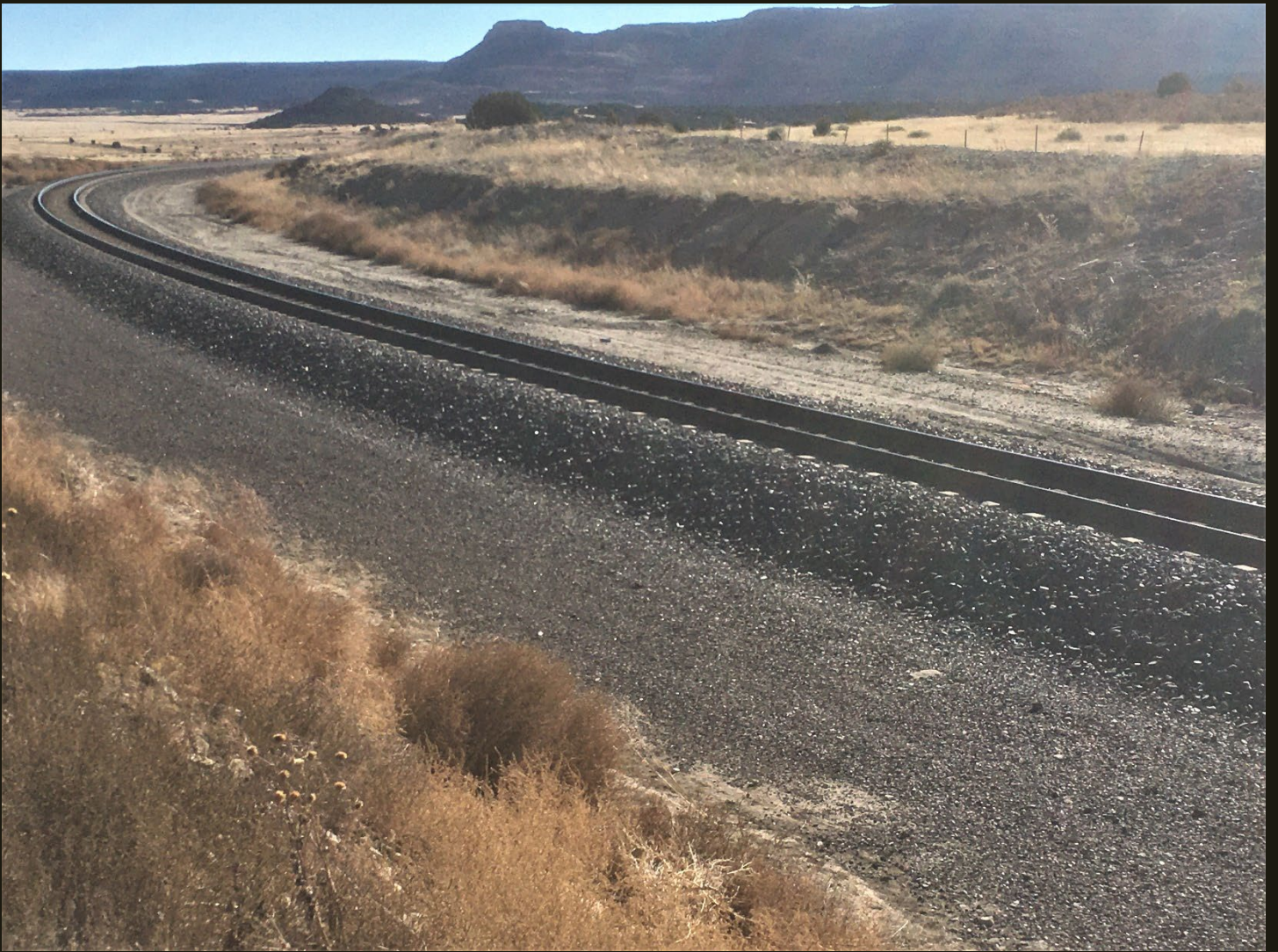
Southeastward view of the DT&FW (1888) at the same location as previous. This is high-grade welded track on concrete ties.
