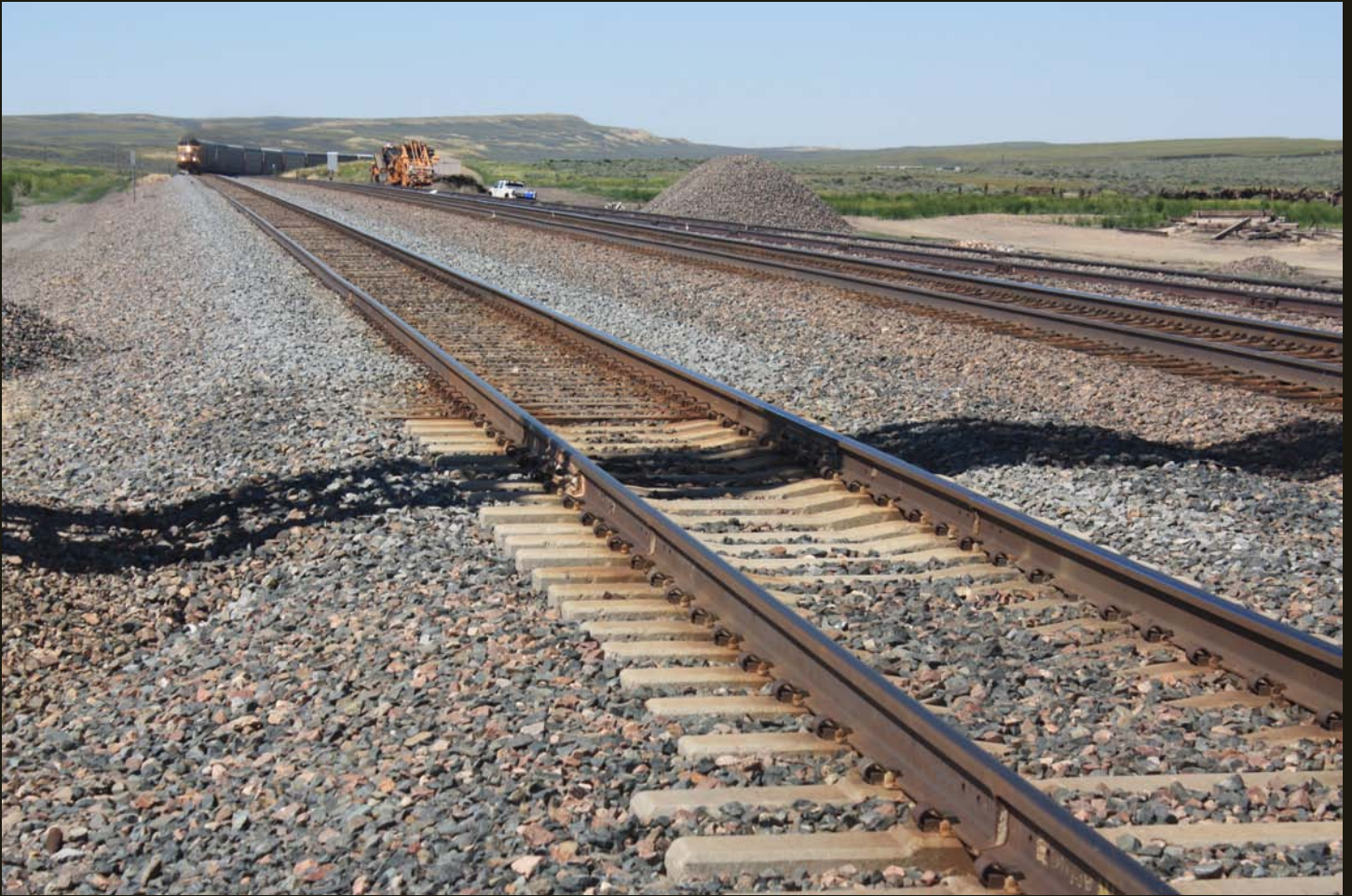
A UP consist plies the western crossing of the Great Divide. Note the partial replacement of wooden ties with concrete ties.
