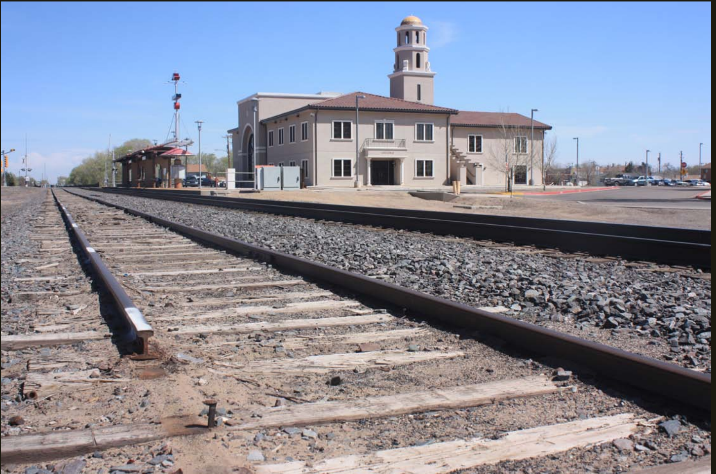
This bolted-rail siding looks out-of-service and was either an older version of the AT&SF mainline or more likely an old siding.
