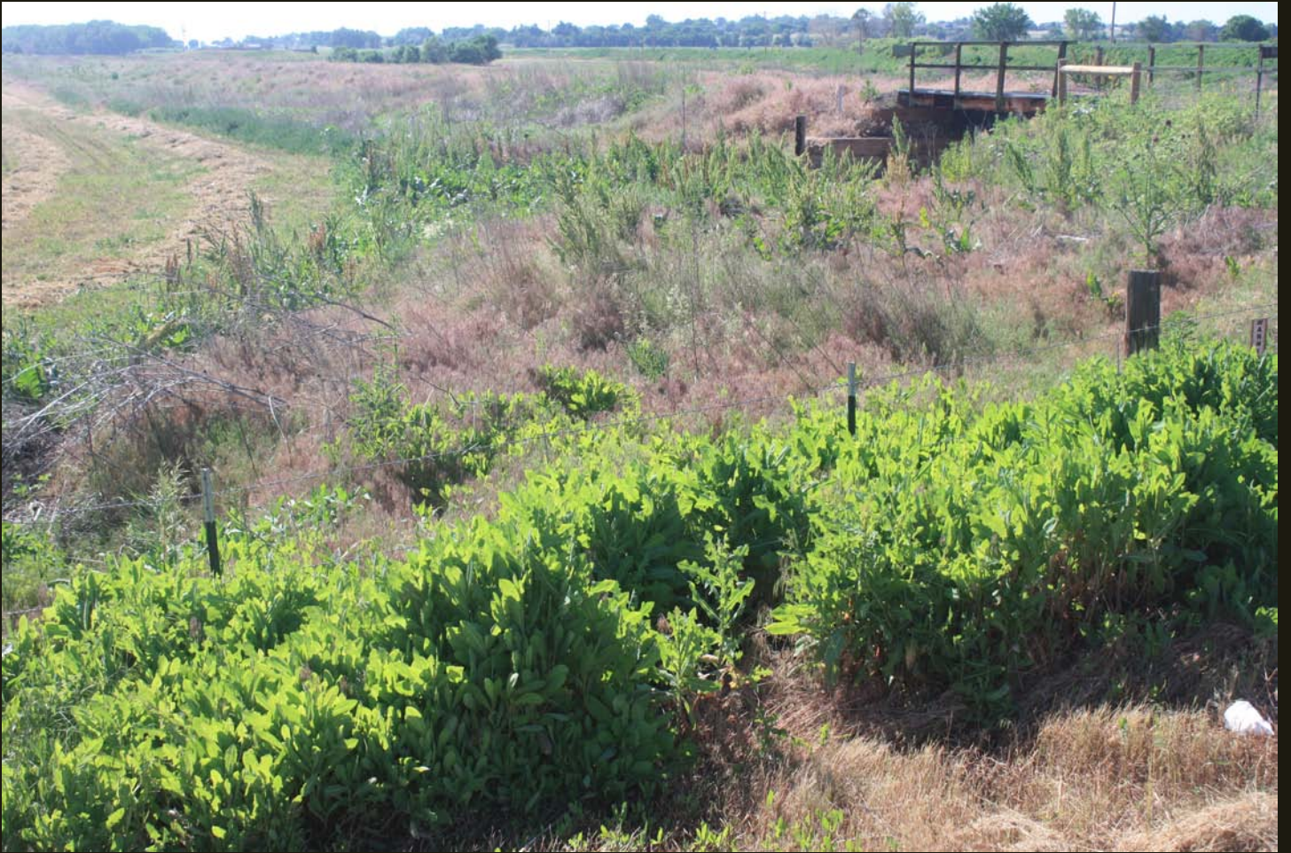
Another view of the small bridge visible in the previous photo for the grade of the UP Julesburg Branch.
