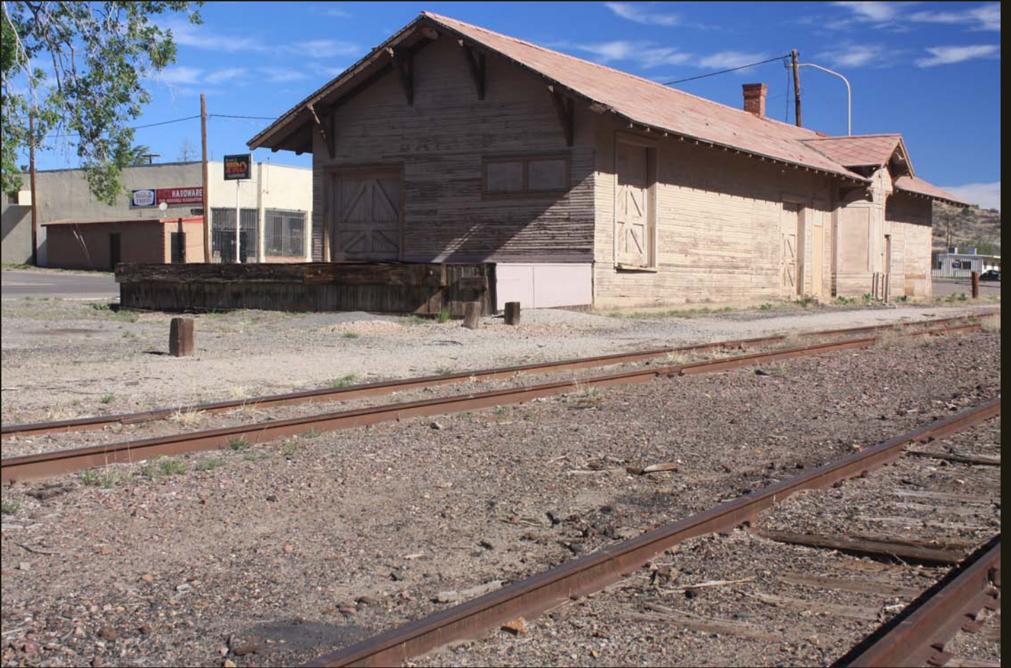
The abandoned SC&N depot at Bayard, about 5 miles north of Hurley.
