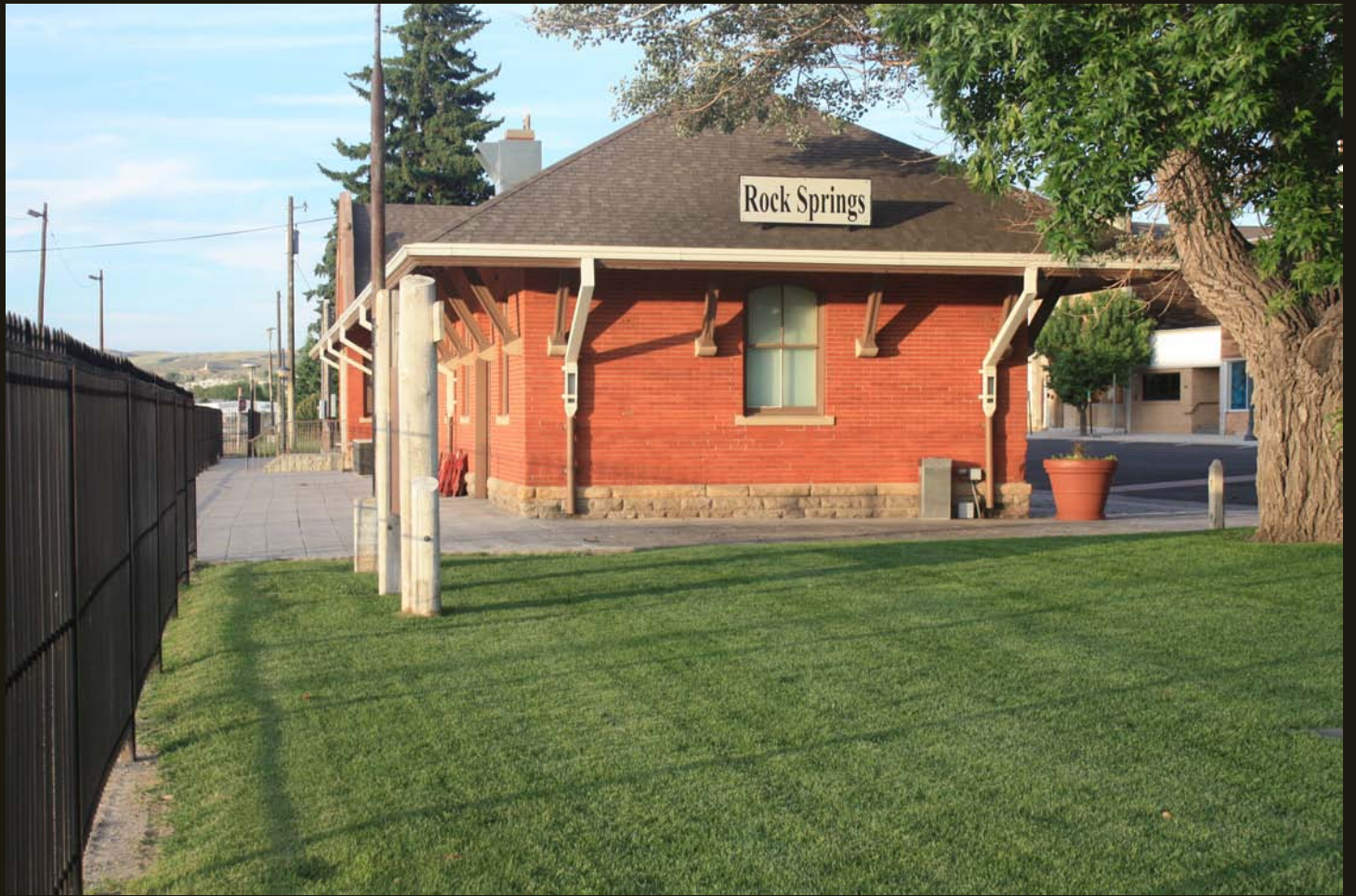
The Rock Springs Depot; the UP mainline is to the left of the fence.
