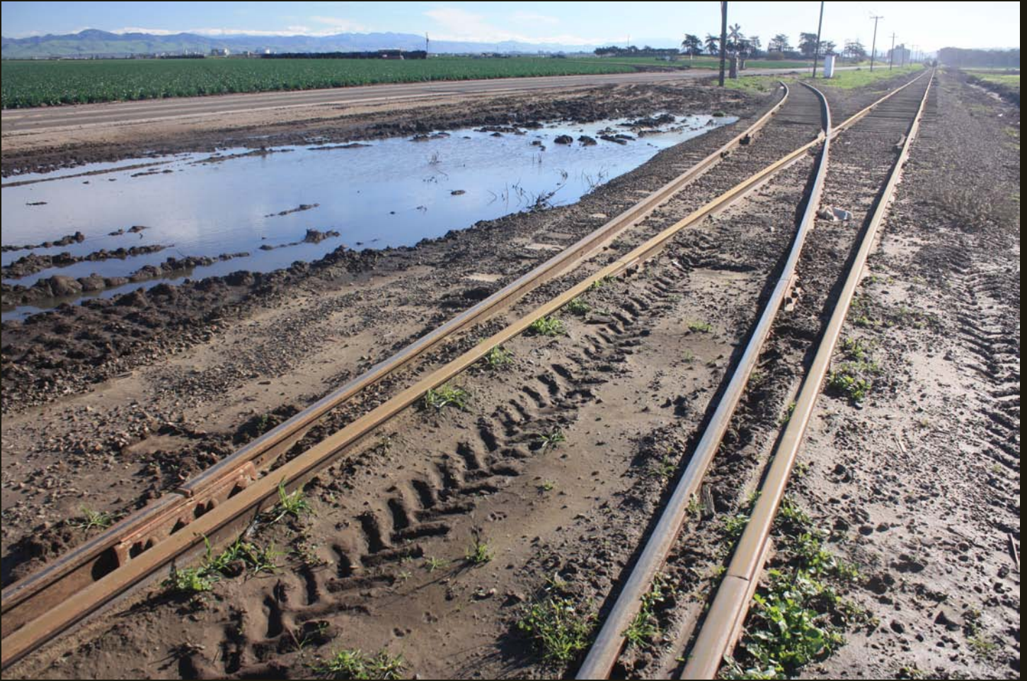
Eastward view of Betteravia Junction, same location as the previous photo. The switch is between the SMV main line to Santa Maria (left) and the spur to the Betteravia beet processing plant (right).
