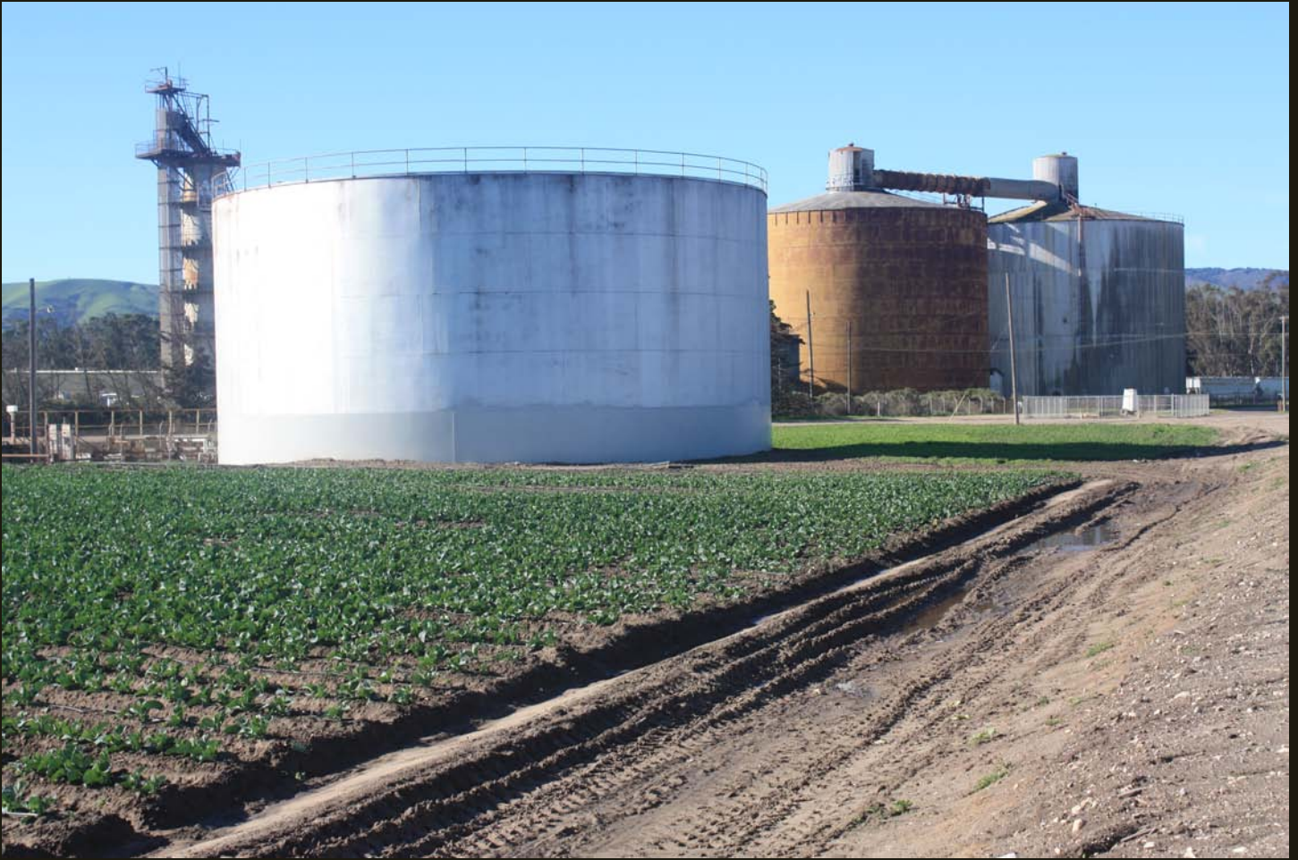
The Betteravia sugar plant facility, which closed in 1993 and is now the SMV headquarters. Note the rolling stock on the longest of the Betteravia spurs.
