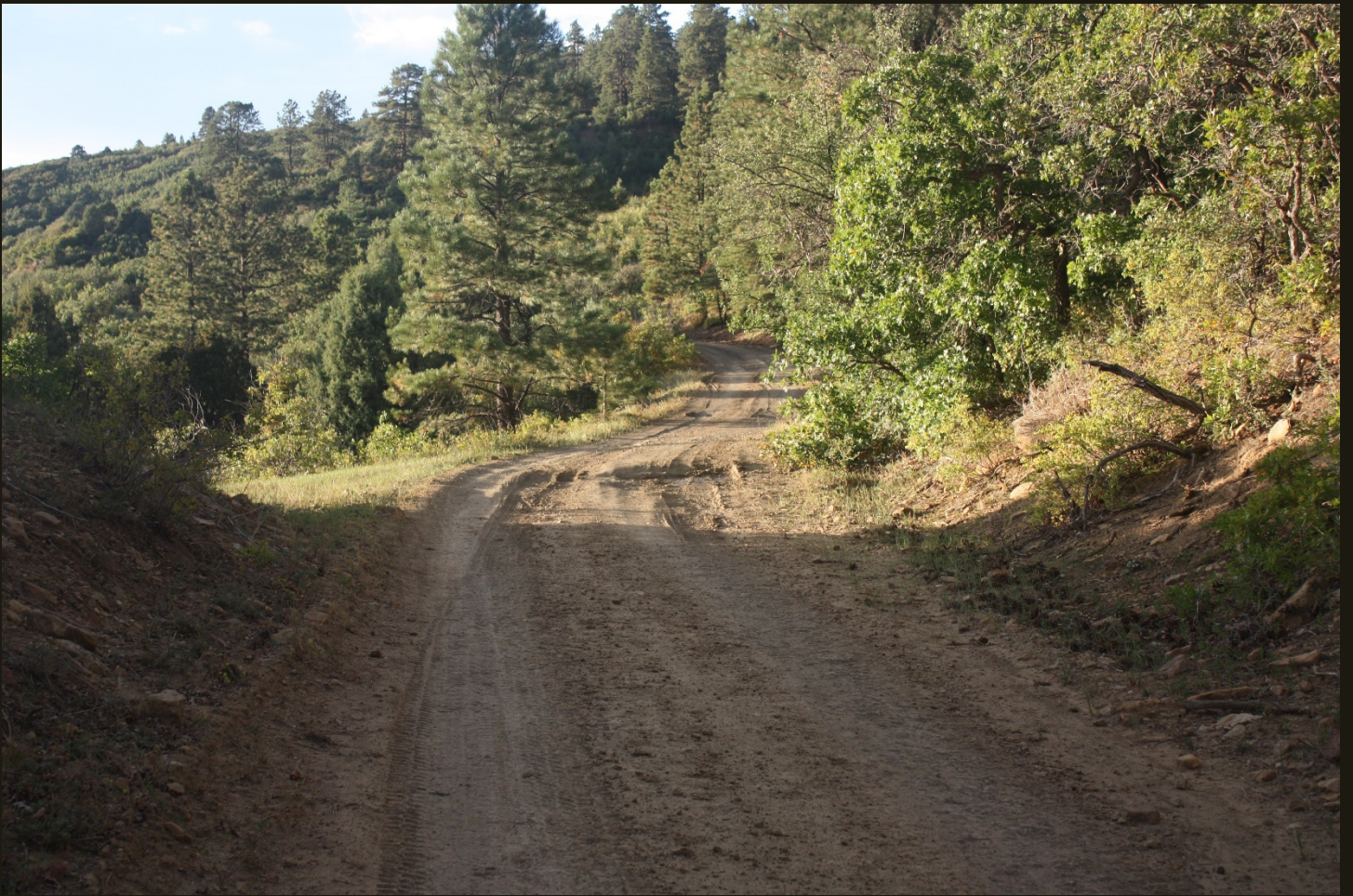
Westward view of the RGS (1891n) at the west end of the deep cut in the previous photo.
