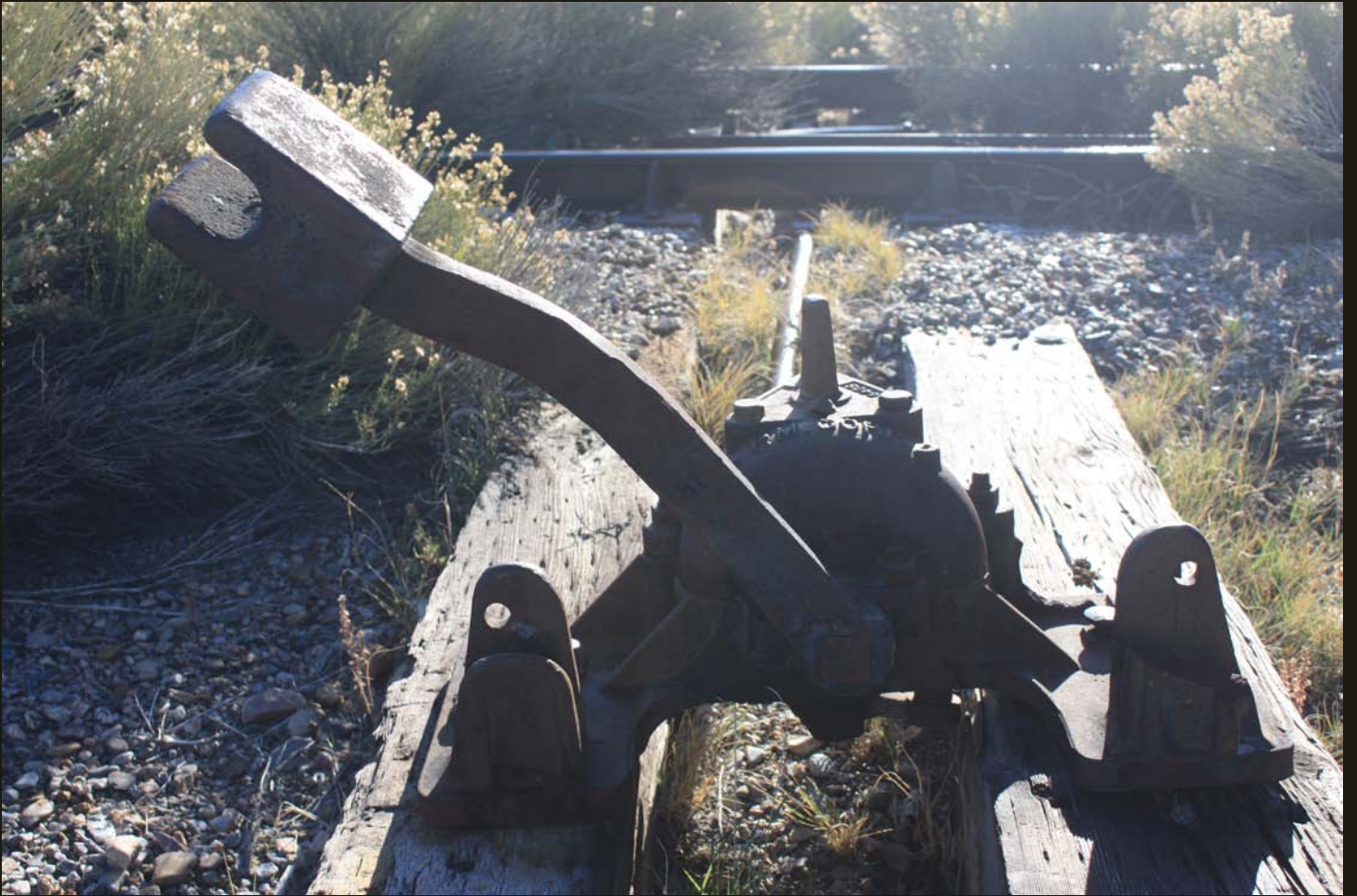
The switch for a siding at Cherry Creek station.
