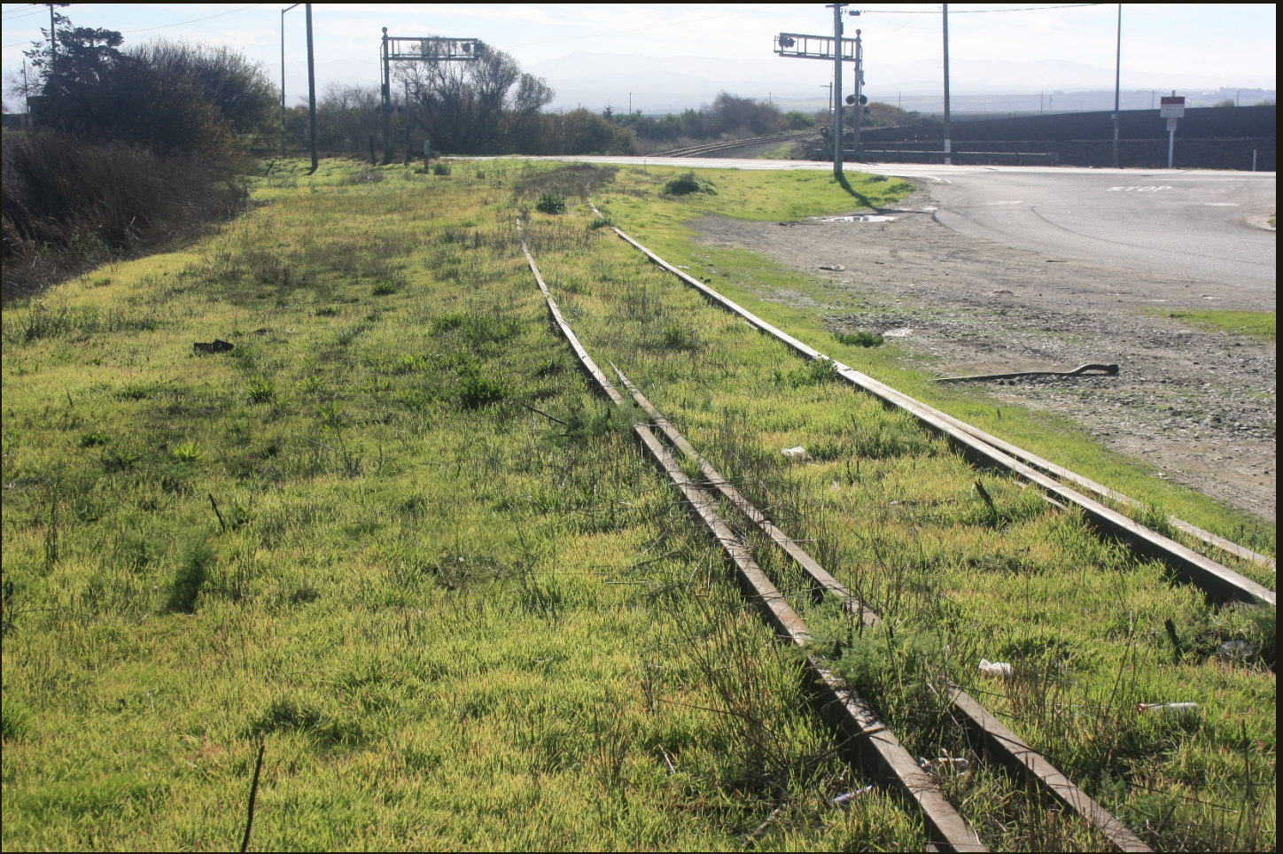
Now we've moved south about 100 yards south looking southwestward at the north branch of the wye for the SP Monterey Branch (1879); the switch in the foreground is the spur to the agricultural facility. The south branch of the abandoned wye, visible in satellite imagery, joins the south branch 1,000 feet down the line (in the distance to the southwest).
