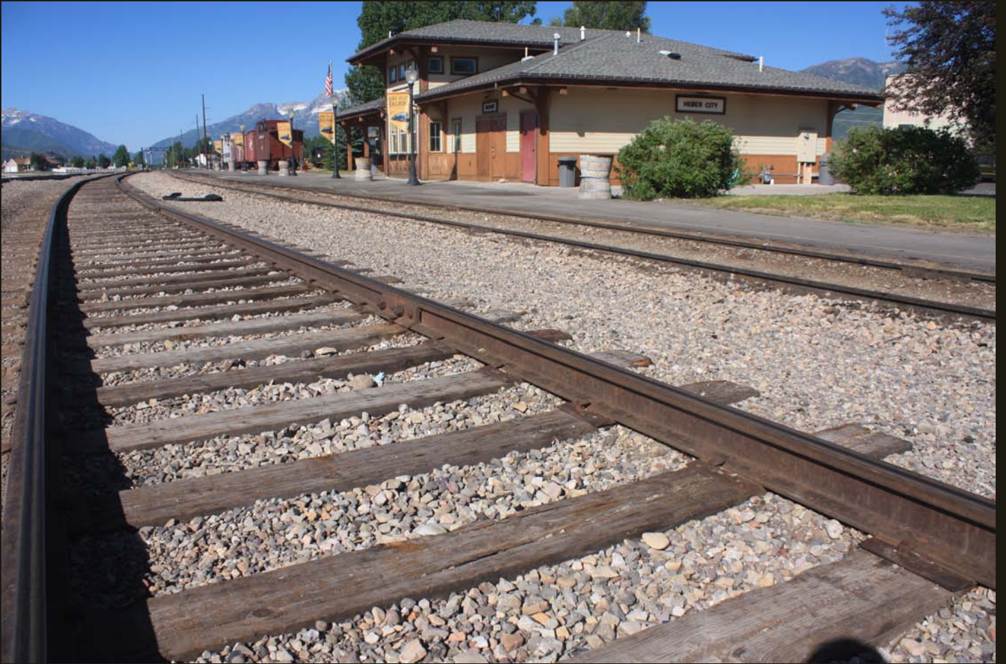
The HV Depot at the end-of-track in Heber City.
