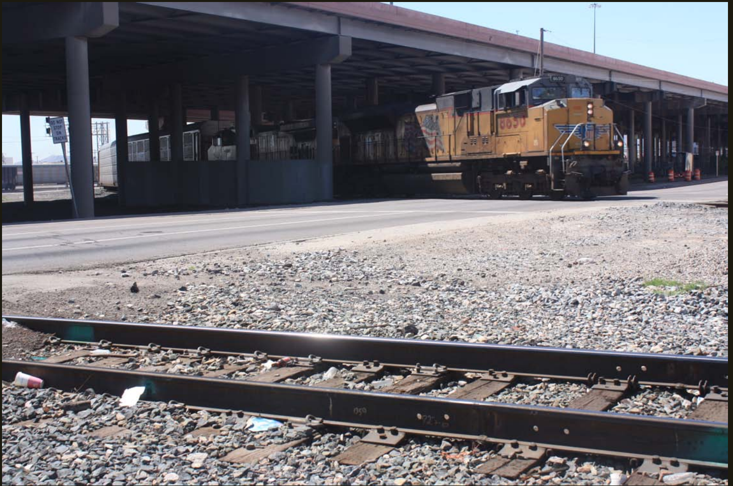
An eastbound UP train switches onto the EP&NE (now UP) line at the El Paso wye; the second leg of the wye is in the foreground.
