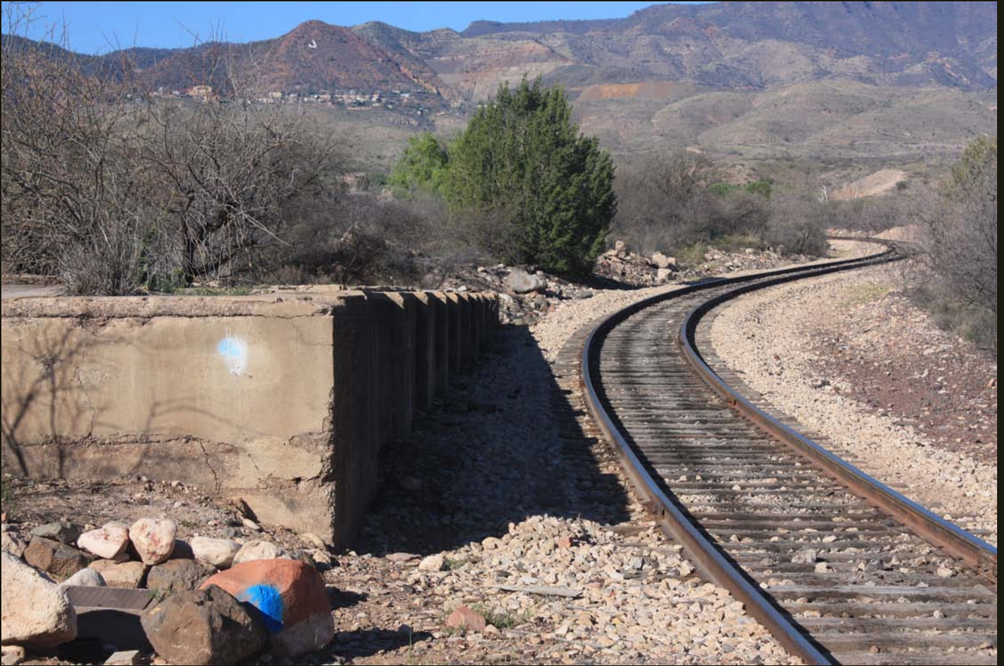
A few hundred yards above the upper end of the Verde Canyon Railroad Depot at an old loading dock. The line winds another 2 miles to the end-of-track at a cement plant (out of view on the right). The town on the side of the hill is the colorful mining town of Jerome.
