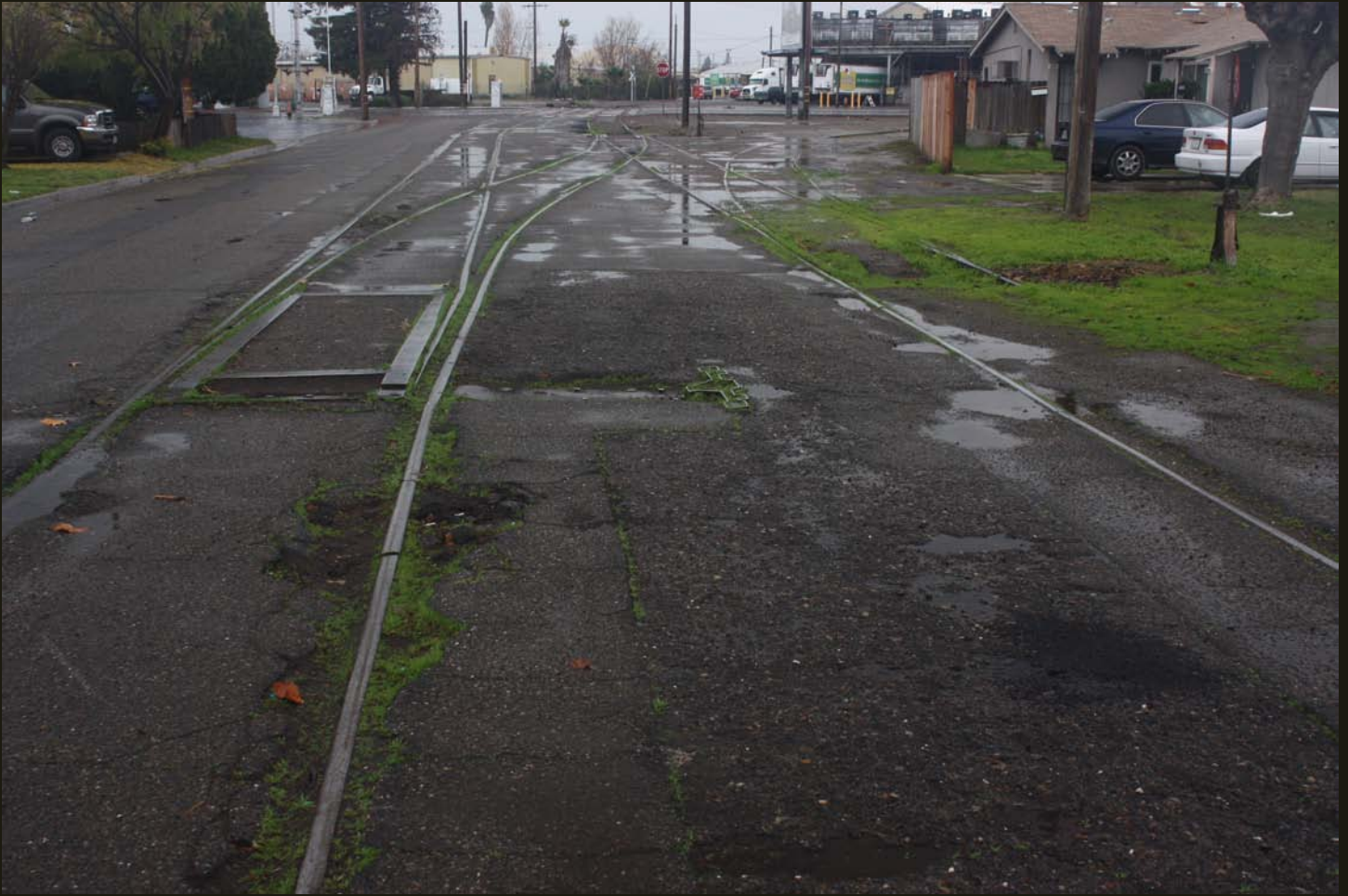
Eastward view at the end of Castor Street and of the Turlock residential area. The two TS (1917) tracks have a crossover and split into spurs at the beginning of the old industrial TS end-of-track in Turlock. Note the switch in the residential yard to the right. I want that!
