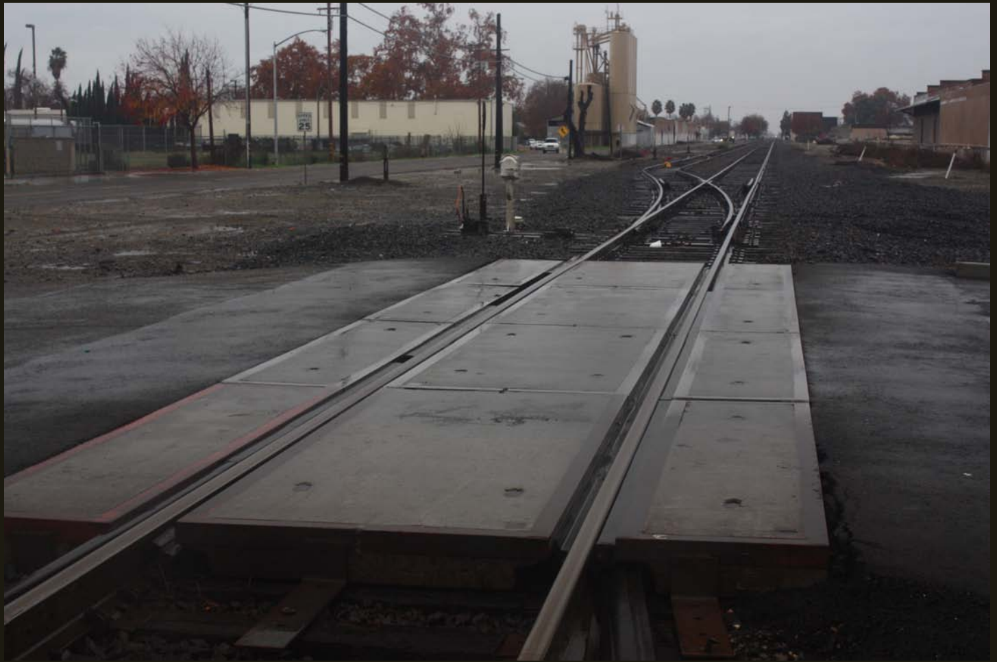
Northwestward view of the SP (1876) at Turlock, a third of a mile southeast of the previous location. The SP (now UP) mainline and siding split just past the road crossing, and the siding splits into a second siding visible in front of the cylinders on the left (west) of the siding. That second siding once connected to the TS (1917), but the tracks are now partially removed (previous photo).
