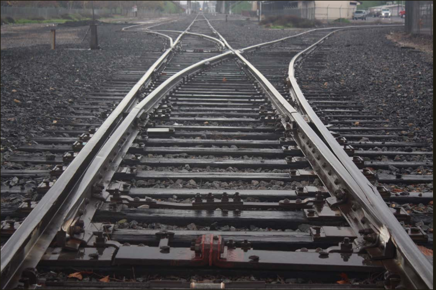
Westward view of the TS (1917), the light in the distance is same train as in the previous photo. Sidings and spurs provide rail access to various agricultural facilities in west Turlock.
