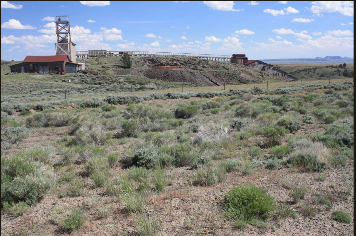
The Carissa Mine, which was never served by rail. Ore was shipped out by wagon and later by truck.
