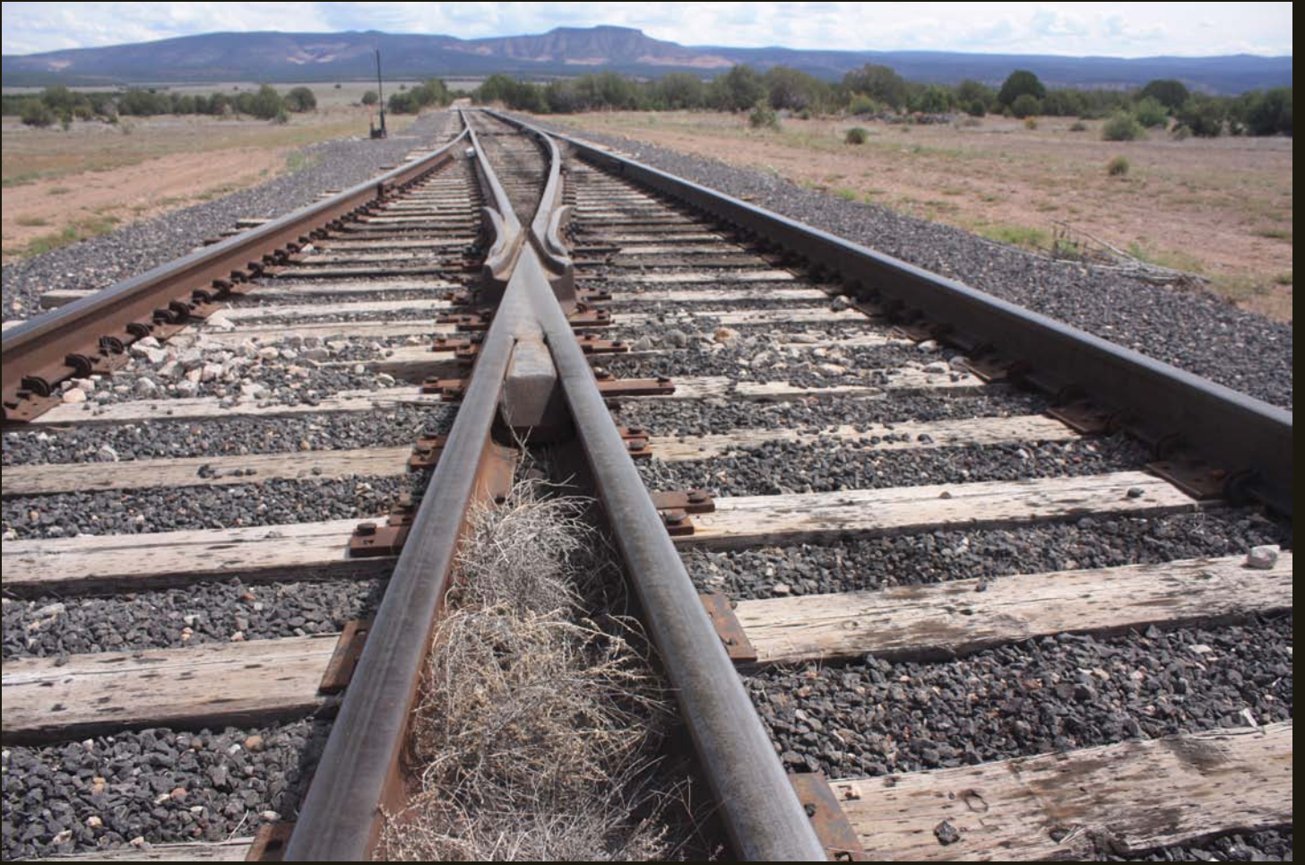
Eastward view of the VV, same location as previous, where sidings converge to one track. Note the relatively flat terrain in the distance, which made the first 5 miles of the VV grade fairly easy, but after that the grade winds its way down to then along the Verde River all the way to Clarkdale.
