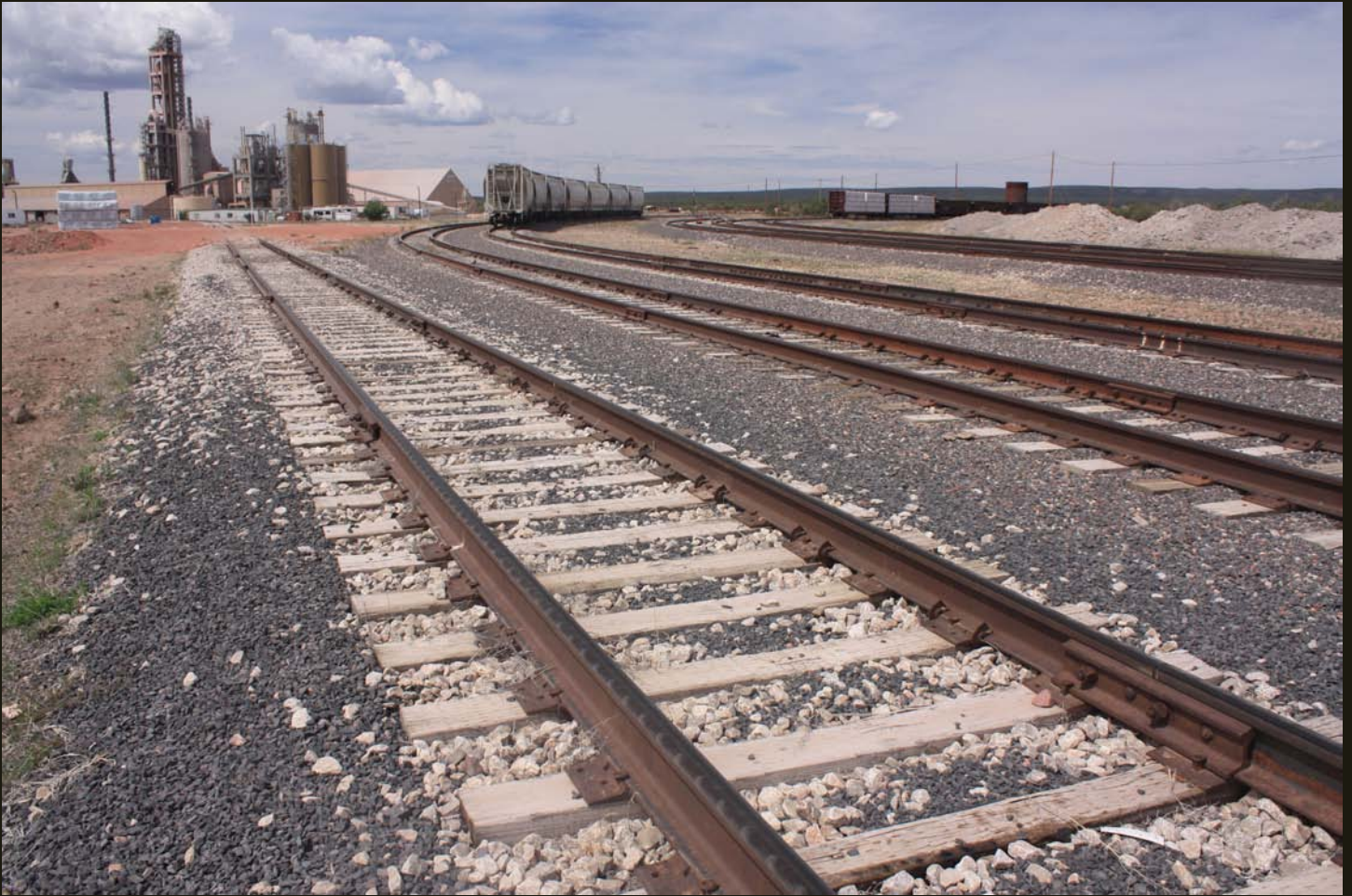
Westward view of sidings along the VV. The eastern switch on the wye, where the two legs meet, is between the two groups of stored cars. Note the back side of the same steel water tower as previous photos. The siding in the foreground services the Drake Cement Plant.
