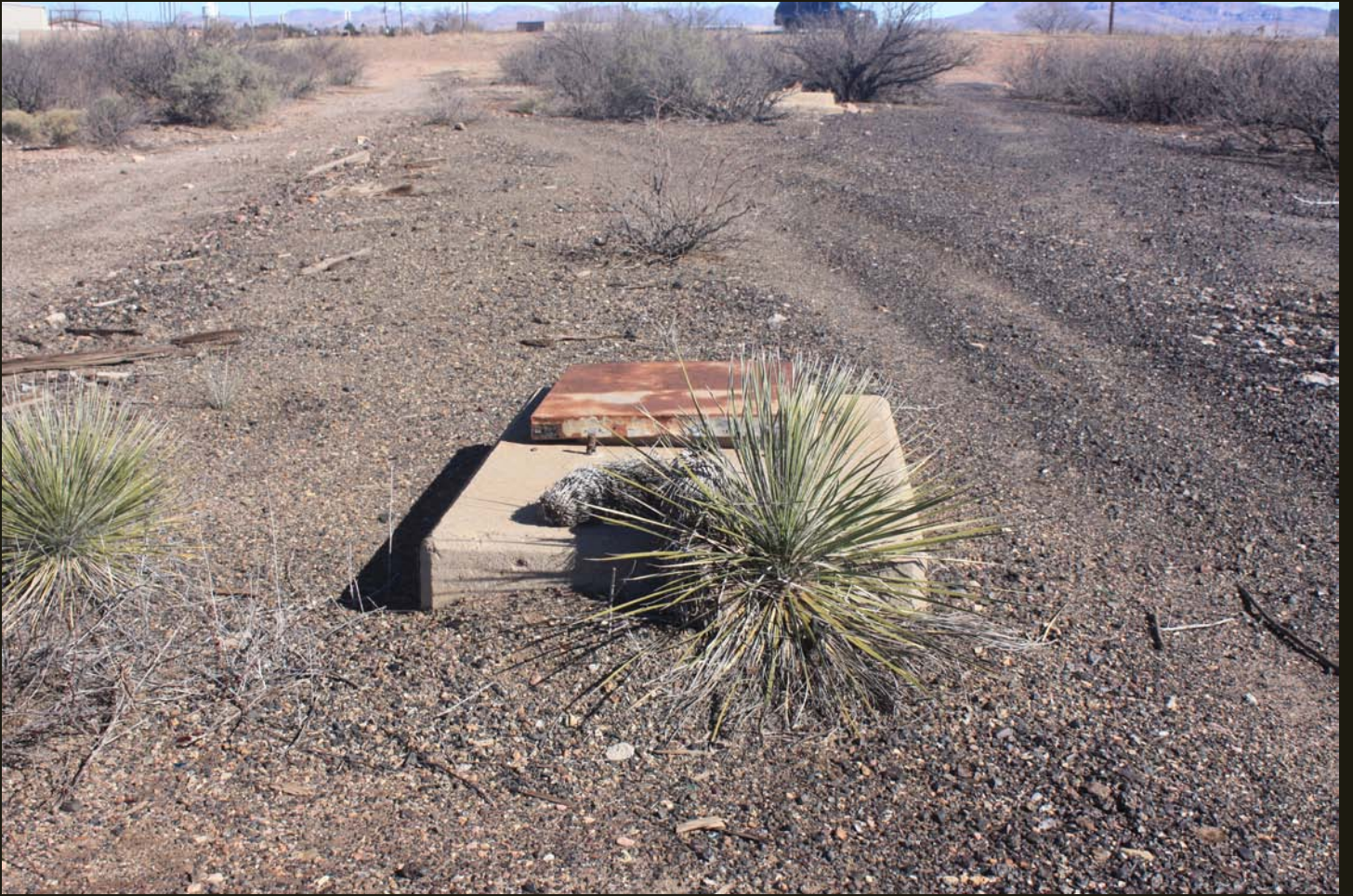
Northeastward view of the EP&SW (1902) on the right and the M&C (1908) on the left. An old foundation is still present between the two.
