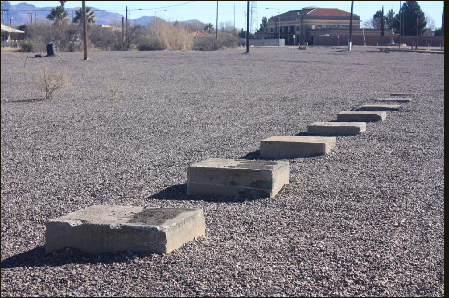
More foundations in the Douglas yard.
