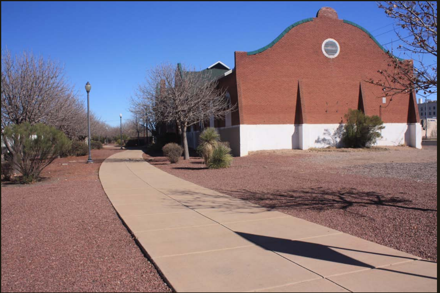
Northward view of the abandoned Nacozari (1902) a half mile south of the previous location. The grade is now a rail-to-trail that follows the railroad grade from the Douglas Depot to the Mexican border. The building was built in 1905 by the EP&SW as a recreation facility for its employees and now is the El Paso and Southwestern Railroad YMCA.
