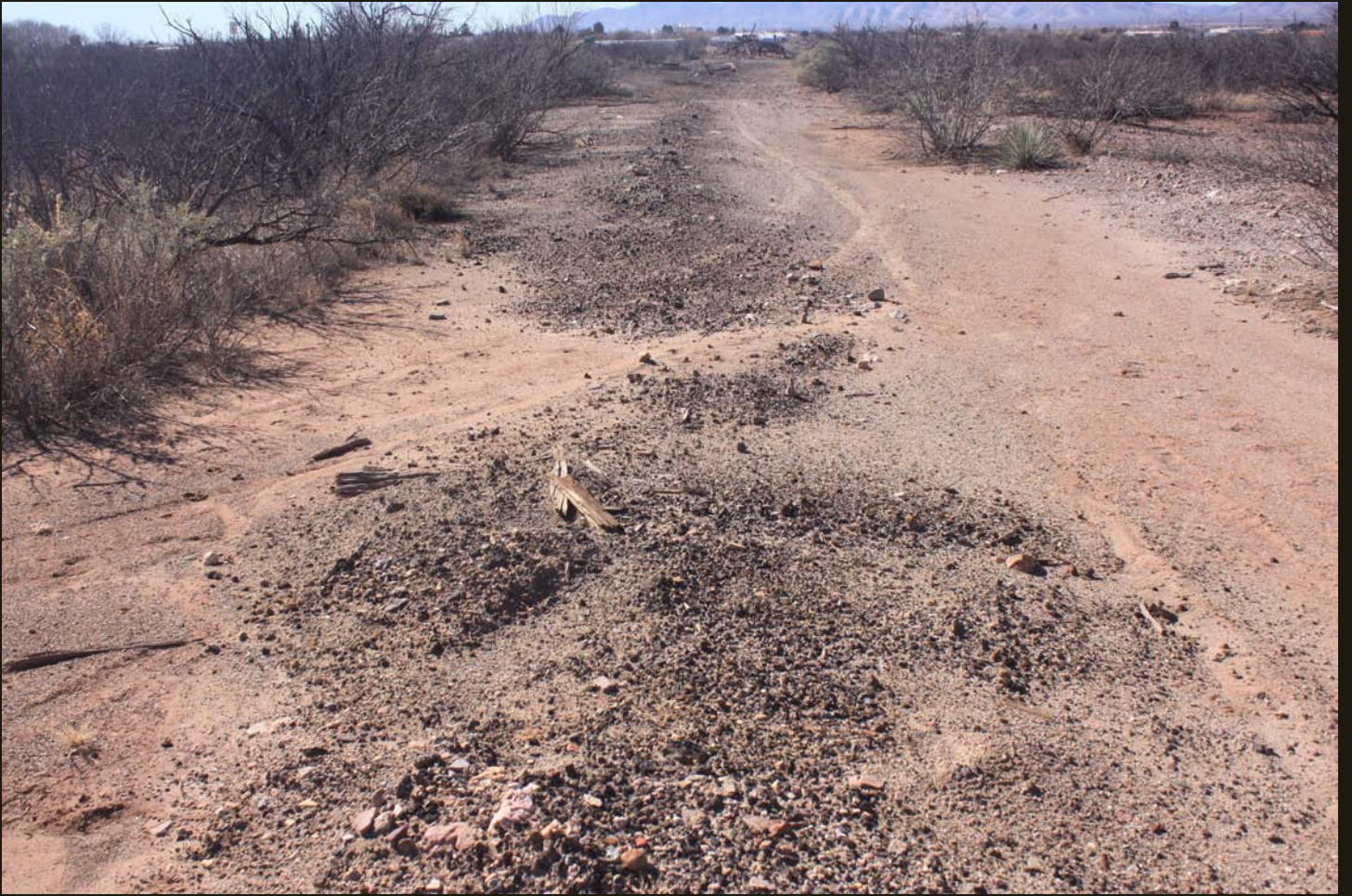
Southwestward view of the M&C (1908) showing detail of the roadbed.
