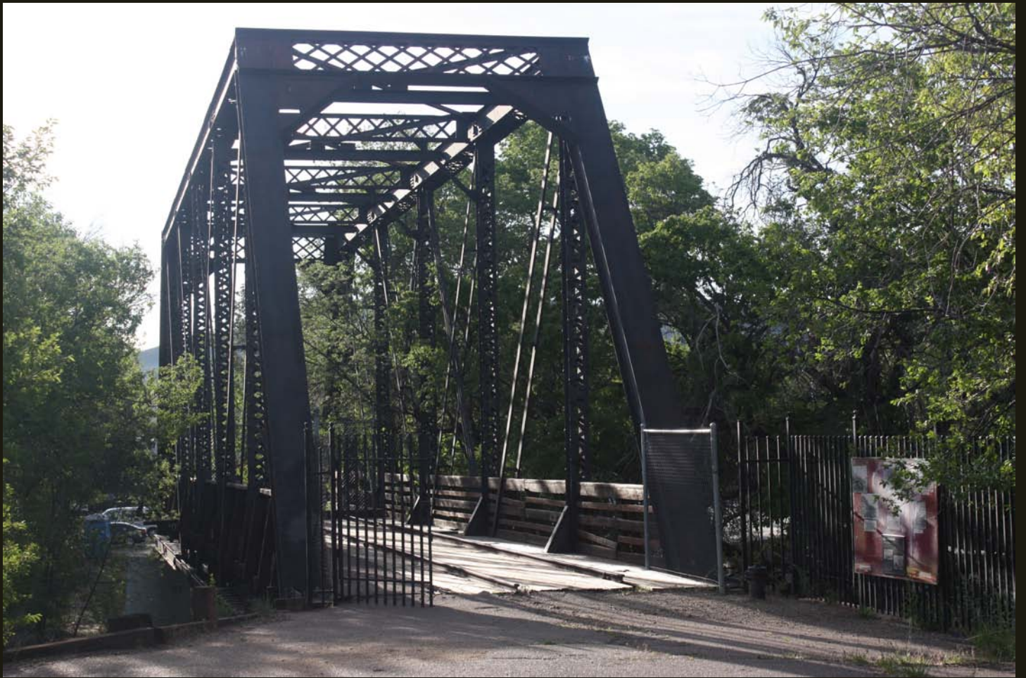
East end of the Granite Creek Bridge in Prescott.
