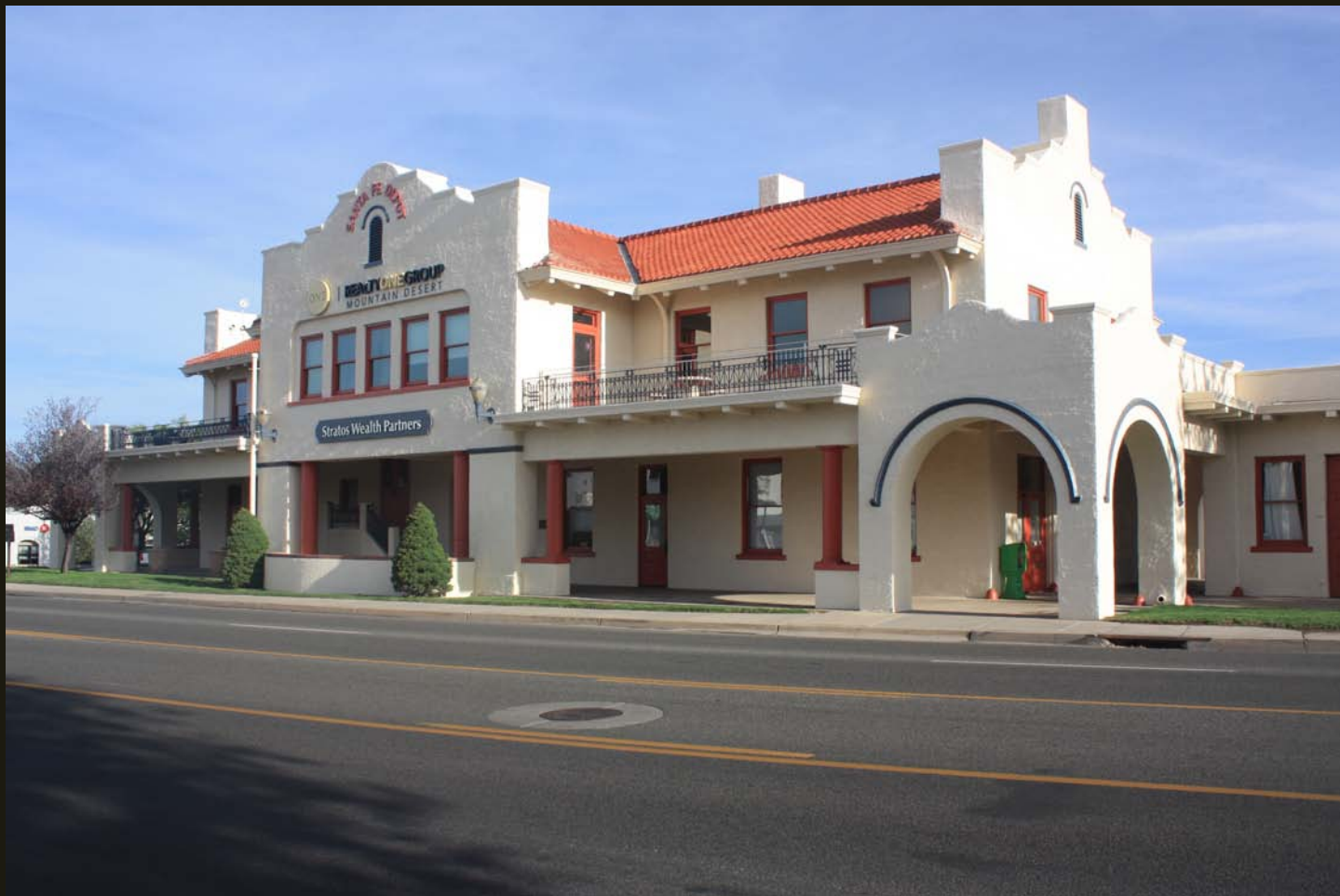
The SFP&P/AT&SF Depot in Prescott is 500 feet east of the Granite Creek Bridge and is now office space; but notice the nod to the building's history as the "Santa Fe Depot."
