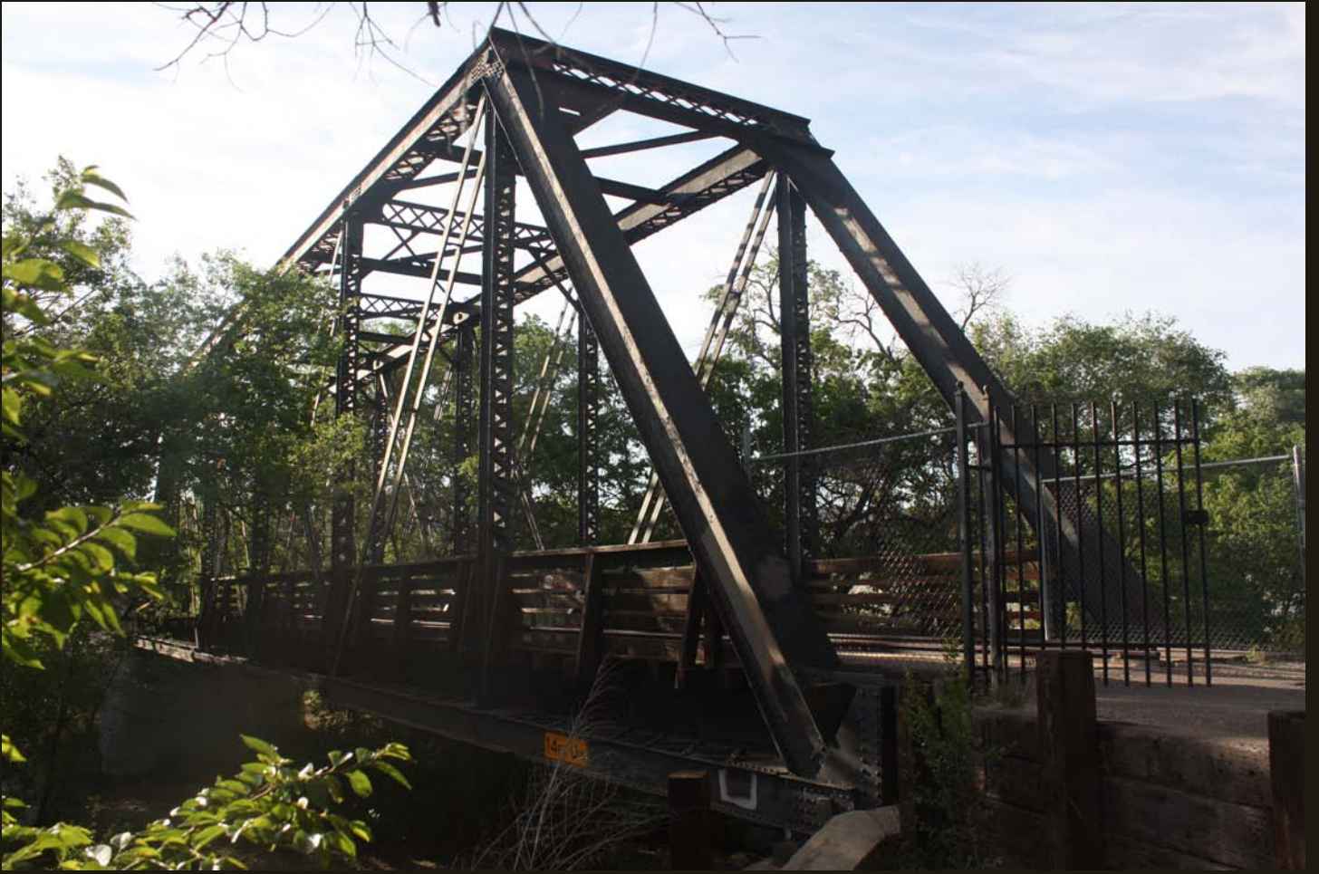
Another view of the Granite Creek Bridge, originally built in 1893 by the SFP&P.
