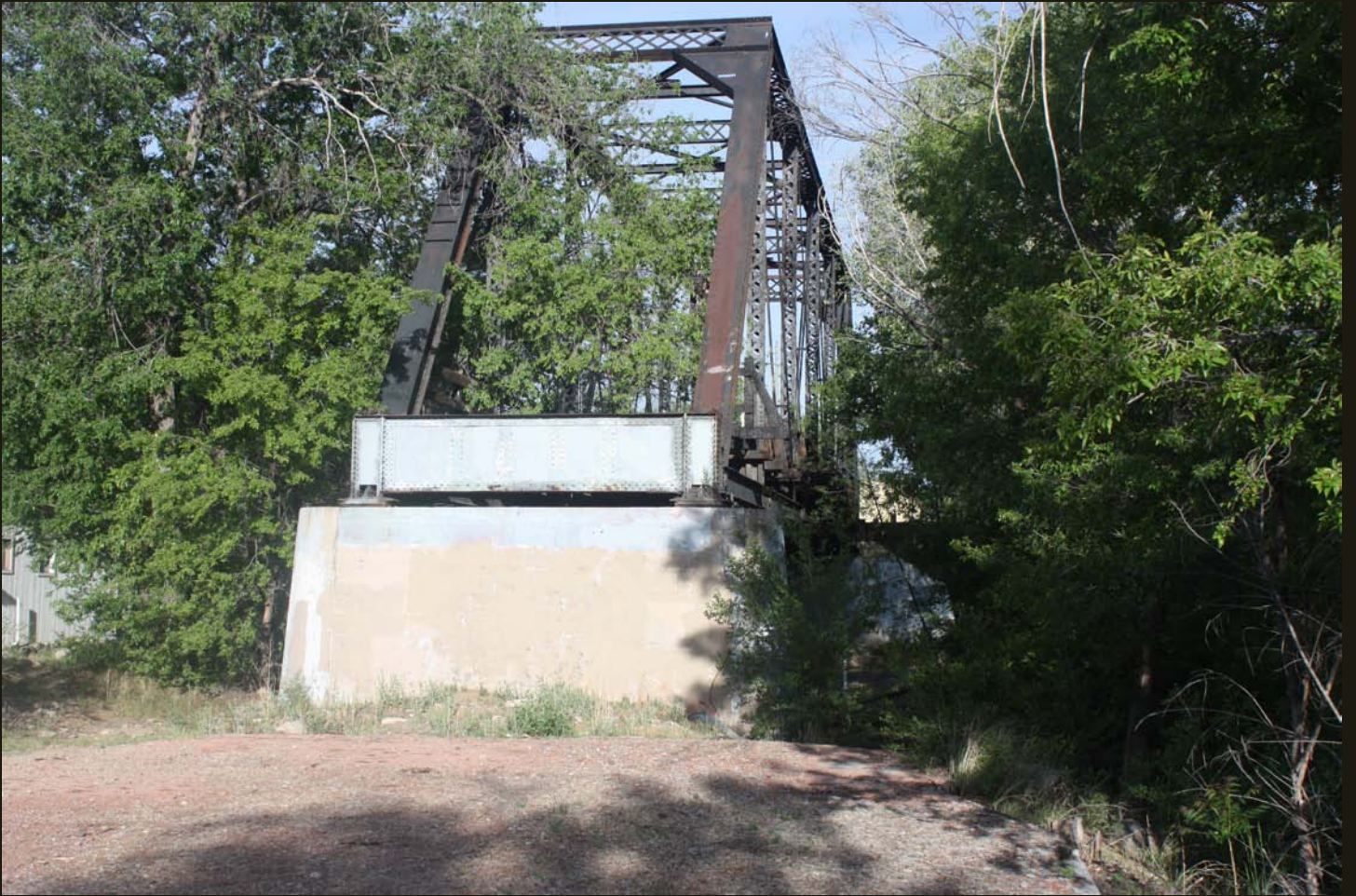
West end of the SFP&P's 1893 Granite Creek Bridge.
