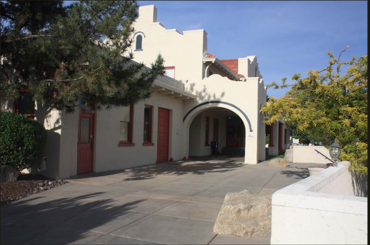
The back of the SFP&P/AT&SF/Santa Fe Depot with a covered passenger loading area; the tracks ran about where the wall on the right is.
