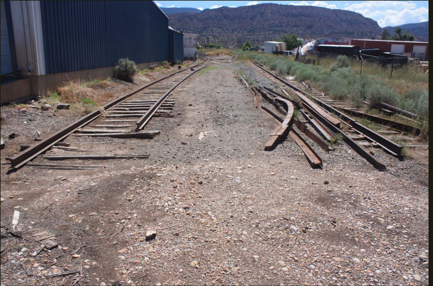
Siding on the Cedar City Branch in Cedar City.
