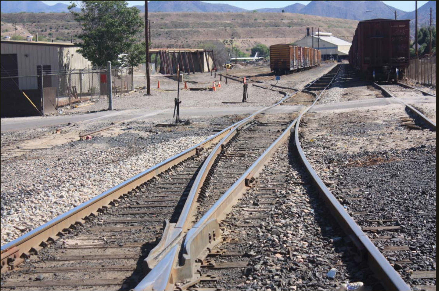
Sidings and car storage on the AE Miami Extension in Miami. Note the tailings pile in the distance.
