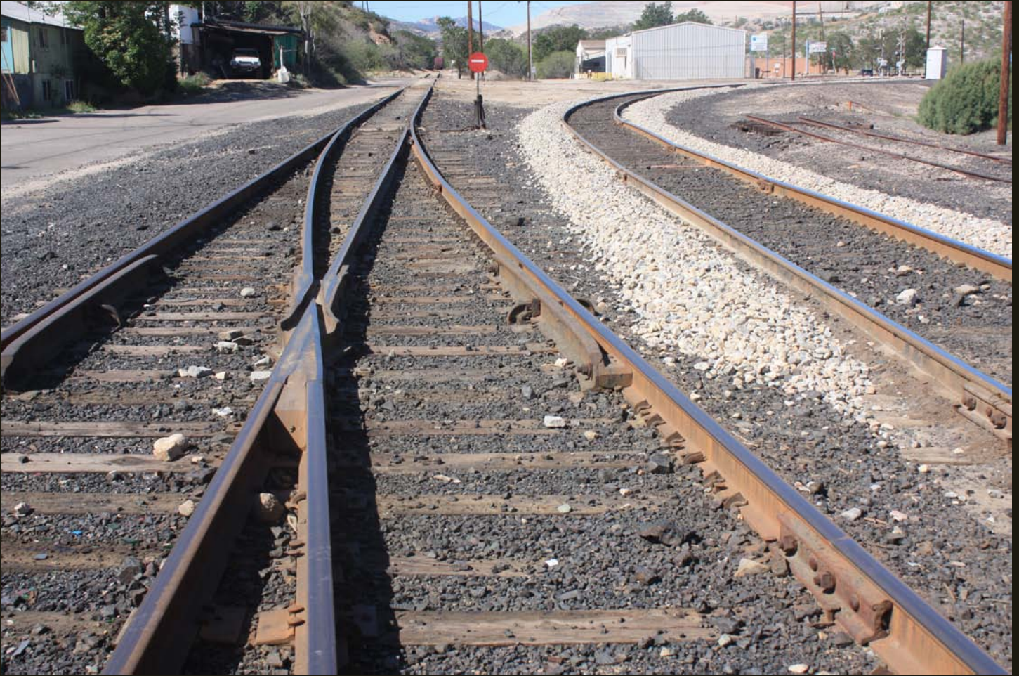
The AE Miami Extension mainline continues up the valley in this westward view and the switchback for the Miami ore processing facilities veers to the right.
