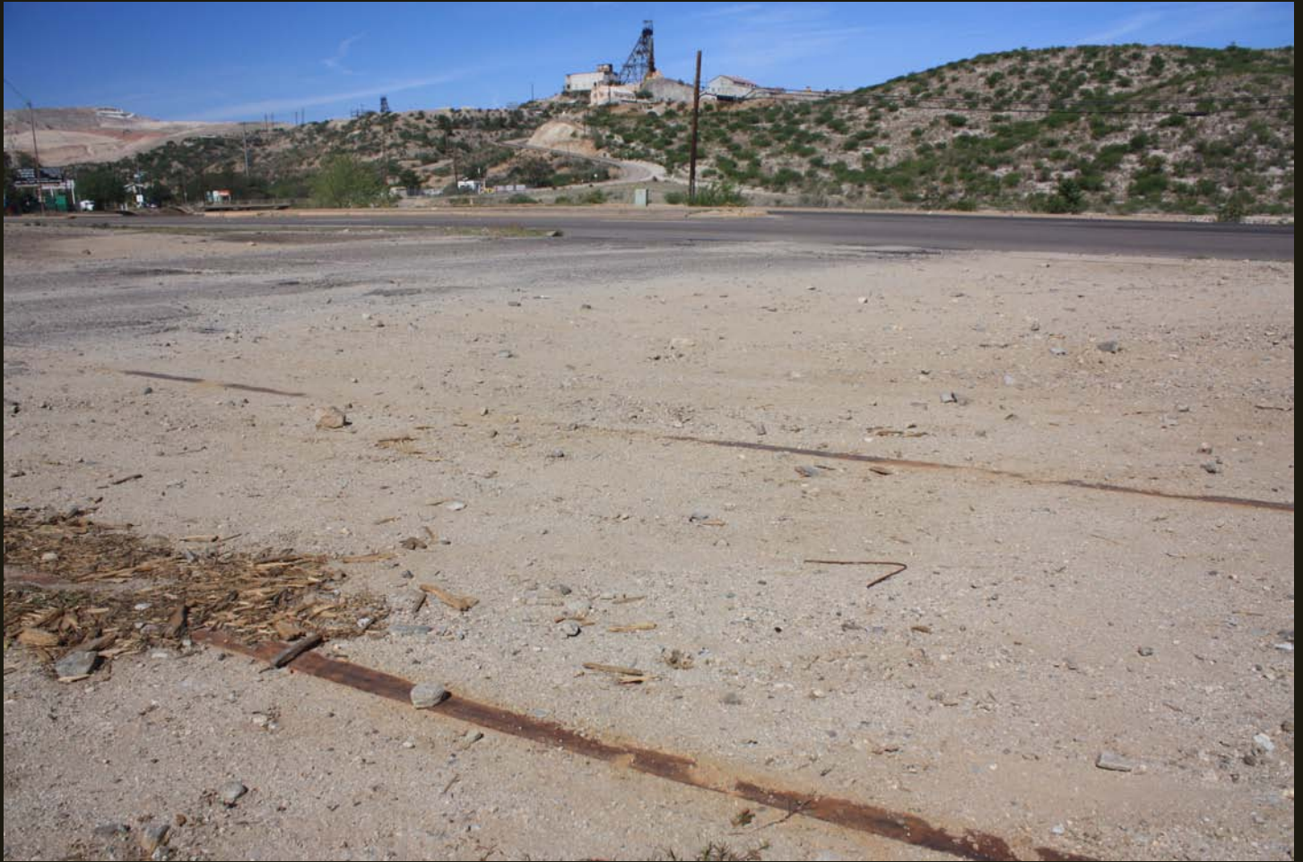
The AE Miami Extension mainline peters out beyond the switchback for the Miami ore processing facilities. Note the old mining headworks in the distance.
