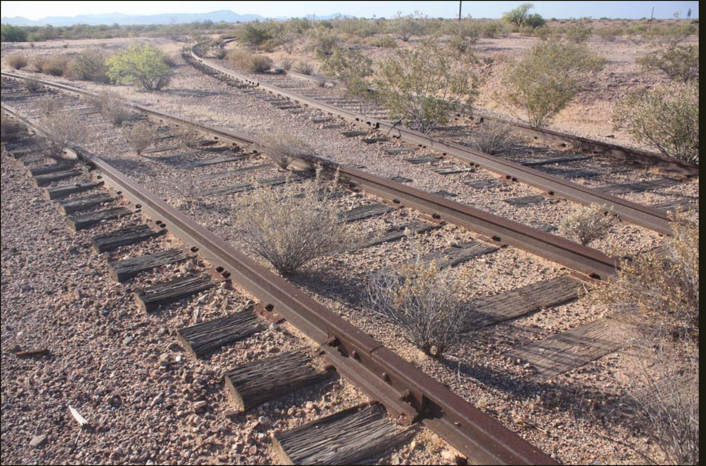
Southeastward view of the two branches of the turning wye near the tip of the wye.
