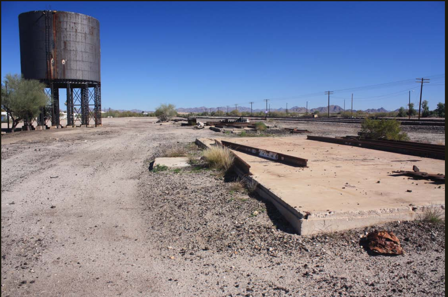
Eastward view of the SP yard at Gila Bend; the tracks for the SP (1881) mainline and sidings are visible to the right, and the sidings and junction for the TC&GB (1916) lie beyond (south of) the SP. The tracks for the SP yard, which once ran near the water tower and loading facilities, have been removed. The old water tower will serve as a reference point in the following photos.
