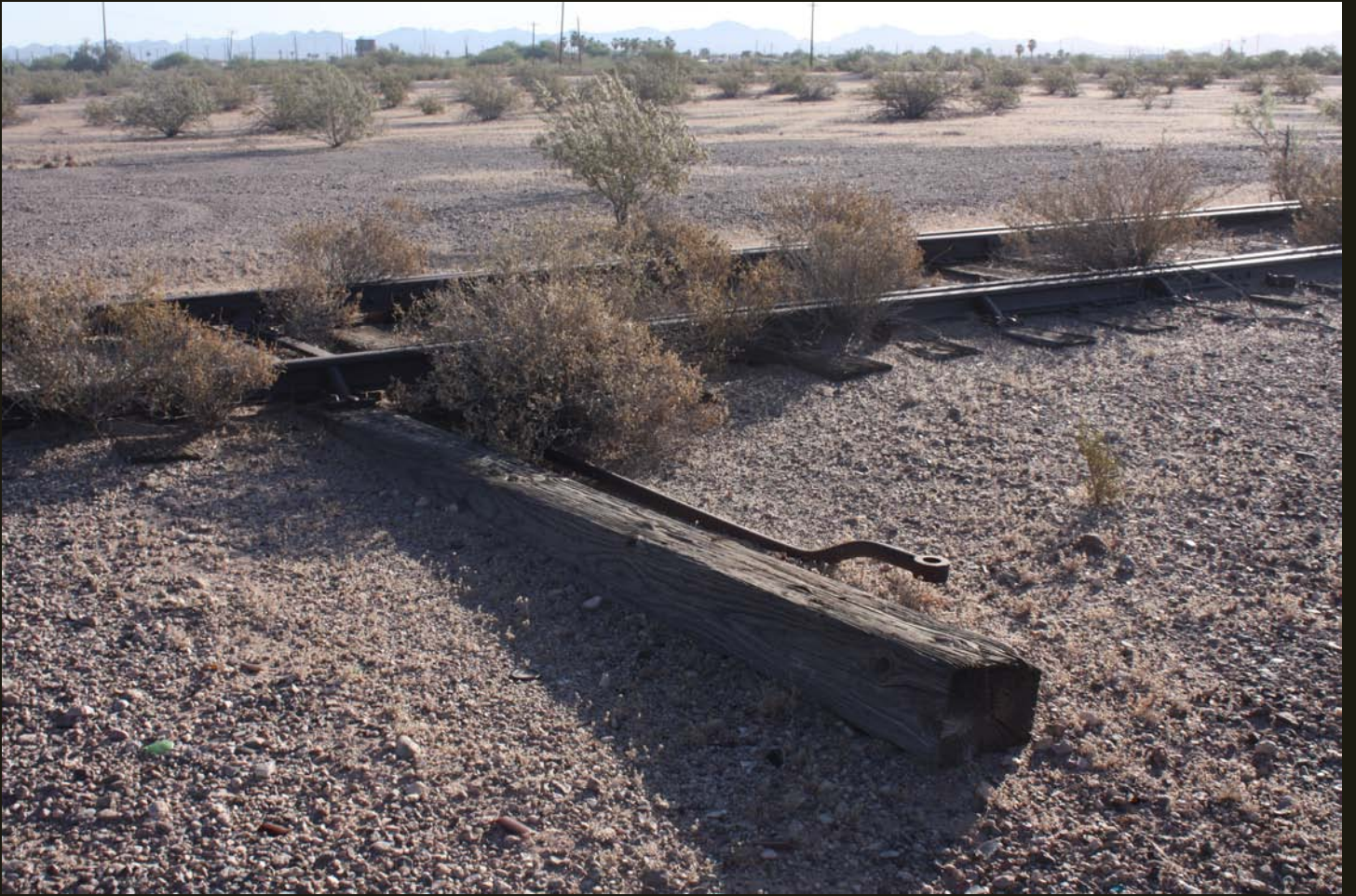
Northeastward view of the switch at the tip of the turning wye; note the same water tower in the distance.
