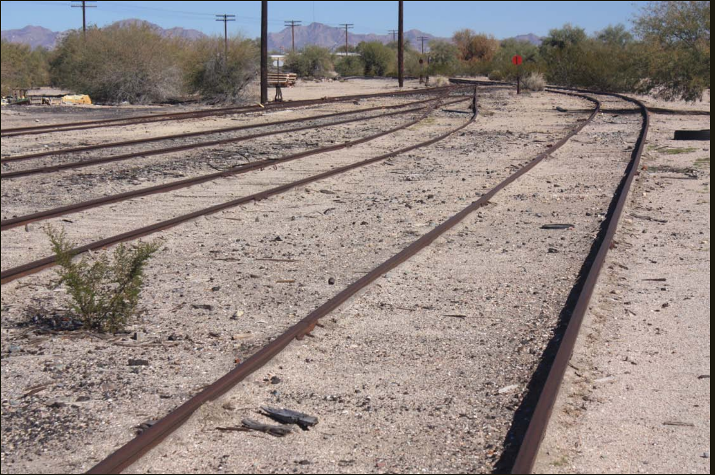
Eastward view of more switches that split the track into the sidings of the TC&GB yard at Gila Bend.
