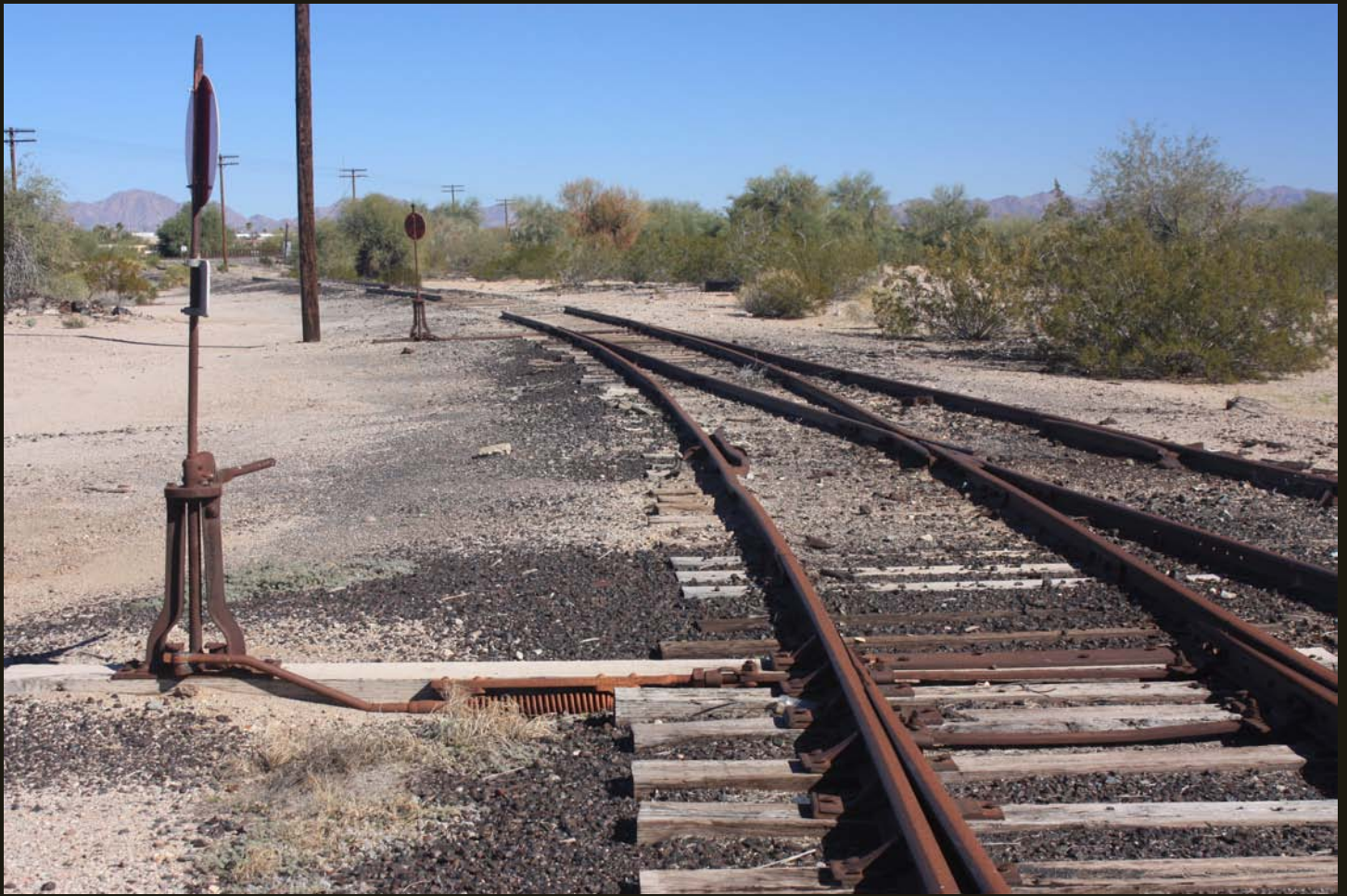
Eastward view of the junction of the SP (1881) and the TC&GB (1916) at the first split of the track entering the TC&GB yard.
