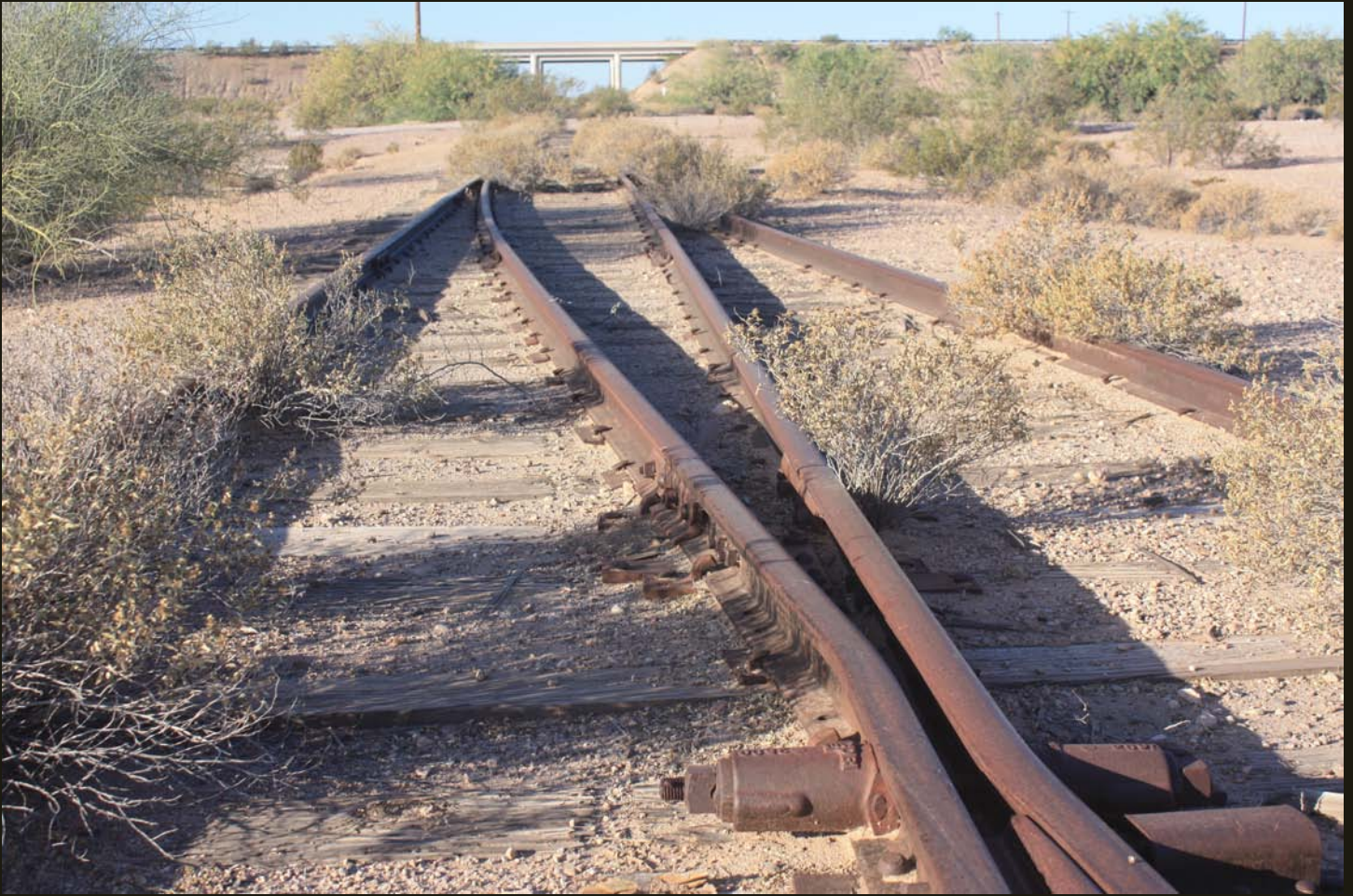
Southwestward view of the southern branch of the turning wye (coming in from the right) and TC&GB (1916) mainline as it heads under Interstate 8 and on to Ajo.
