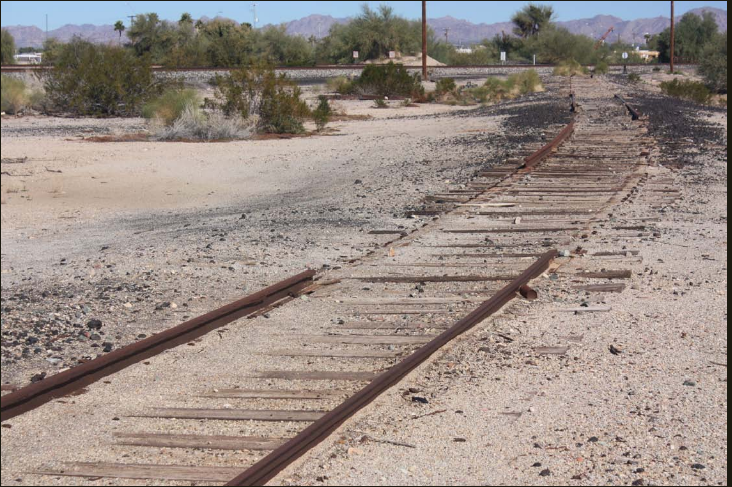
Northeastward view of the junction between the SP (1881), which runs across the entire image in the distance, and the TC&GB (1916) in the foreground. This is the TC&GB's only connection to other roads and is clearly not usable – the TC&GB is cut off from the outside world at this location.
