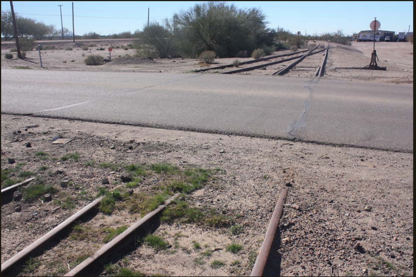
Westward view of the converging tracks at the west end of the TC&GB yard, same location as previous. In the distance, the TC&GB (1916) converges to the single track that curves southward to Ajo. Because the TC&GB-SP junction is a single switch, shown here (rather than a full wye), and a turning wye was built 2,000 feet down the line.
