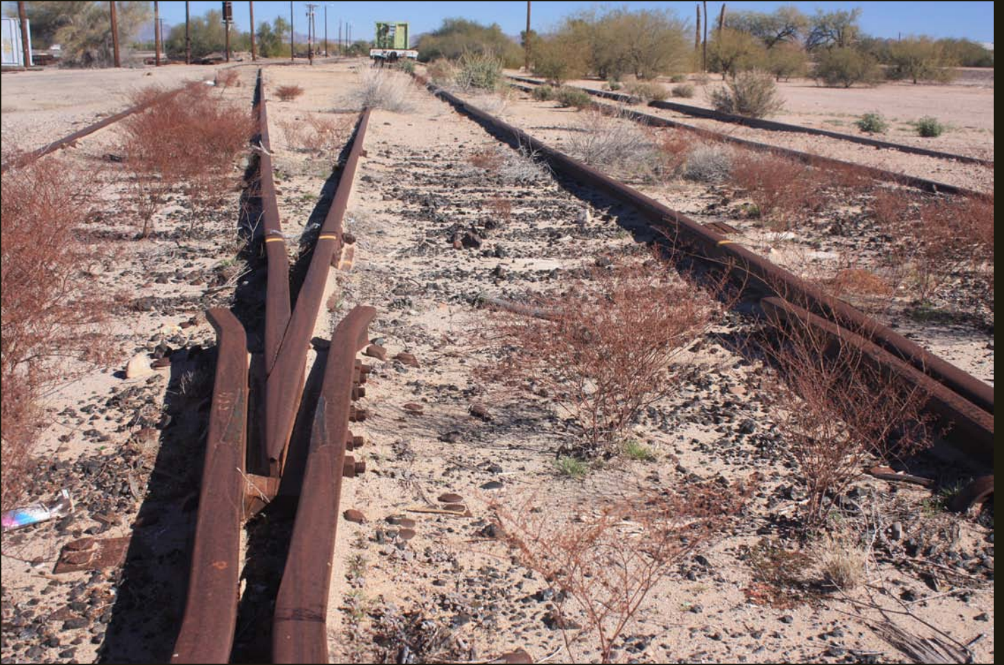
Eastward view of the converging tracks at the west end of the TC&GB yard, same stored cars as before.
