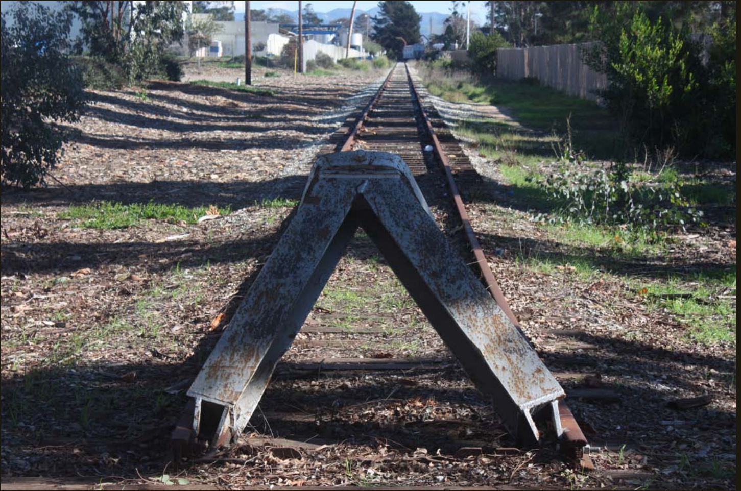
Eastward view of the SMV (1911) southern end of track, 3 miles south of the previous location and a half mile west of the PC (1887) grade; this is a spur of the SMV, just north of the World War II airbase.
