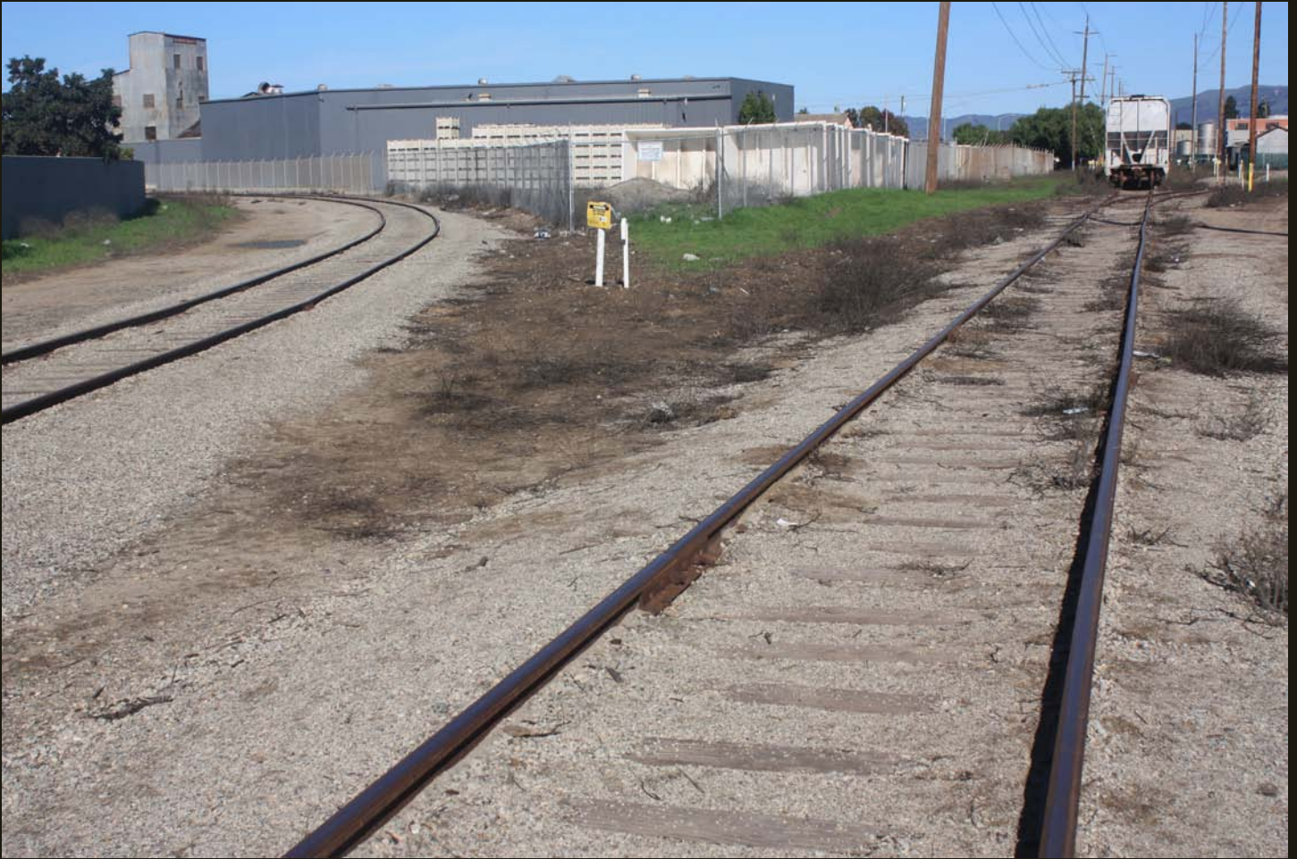
Northward view of the PC (1887) grade, a few steps south of the previous photo, with the same stored car and the switch for the eastern half of the wye in the right distance. The branch to the left is the western half of the wye, built by the SMV in 1911 on a larger radius than the eastern half of the wye.
