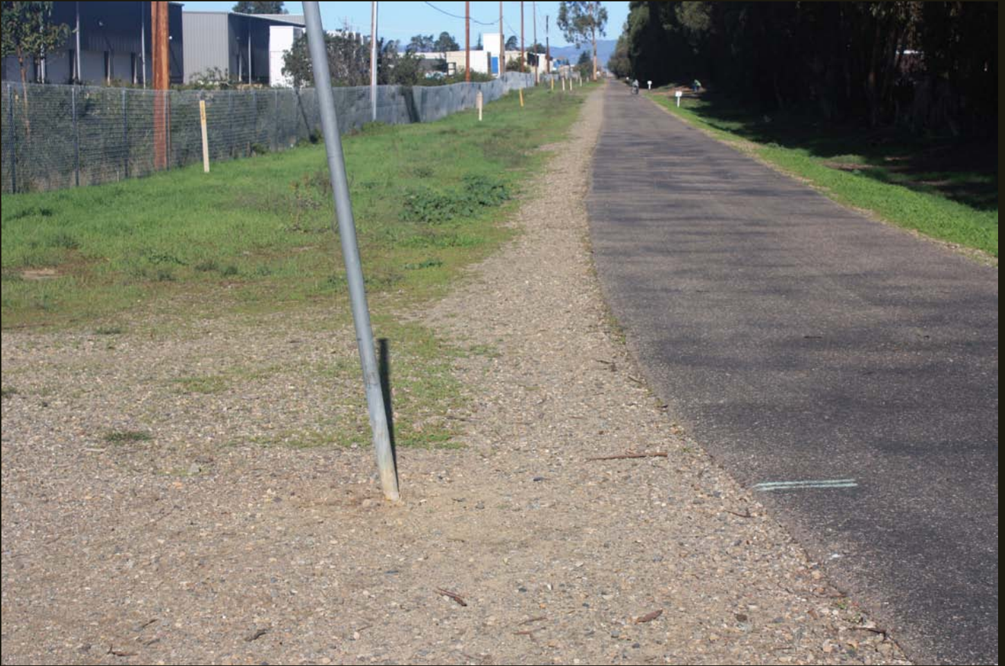
Northward view of the PC (1887) grade, a half mile south of the junction with the SMV spur in the previous photo. The abandoned grade is now the Santa Maria Valley Railroad Trail. Note the jog in the trail off of the railroad grade in the foreground.
