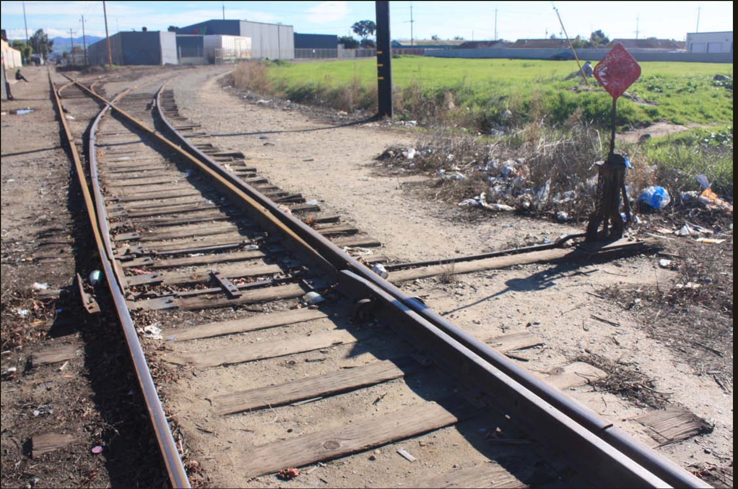
Eastward view of the SMV (1911) a few hundred feet west of the crossing, which is in the left distance. The branch to the right is the western half of the SMV wye. Note that the western branch of the wye does not have rust, but the siding (second switch) and the main line to the east are rusty.
