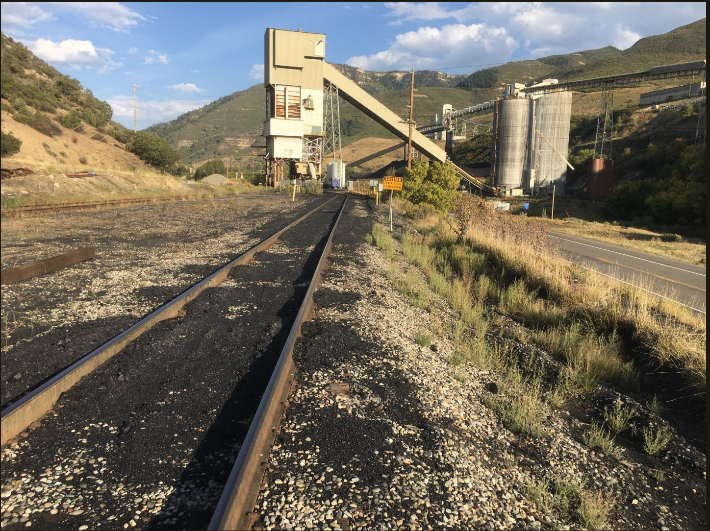
Eastward view of the D&RGW North Fork Branch (1902n) 1 mile to the east of the town of Somerset (previous location) and 1 mile shy of the end of track. The facility is for loading coal conveyed from mines higher up the mountain. Note the coal incidentally spilled along the tracks. There are no coal facilities past this point, just 1 mile of track to line up hopper cars for loading at this facility.
