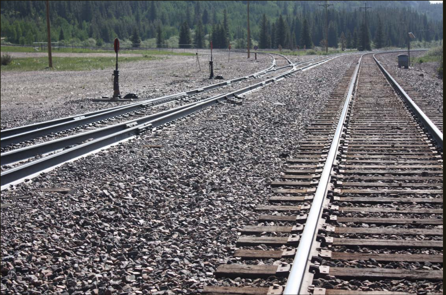
Eastward view of the DNW&P (now UP) mainline and the west branch of the wye; the first switchback of the DNW&P Rollins Pass Route is in this view but was re-graded as a turning wye when the Moffat Tunnel was completed.
