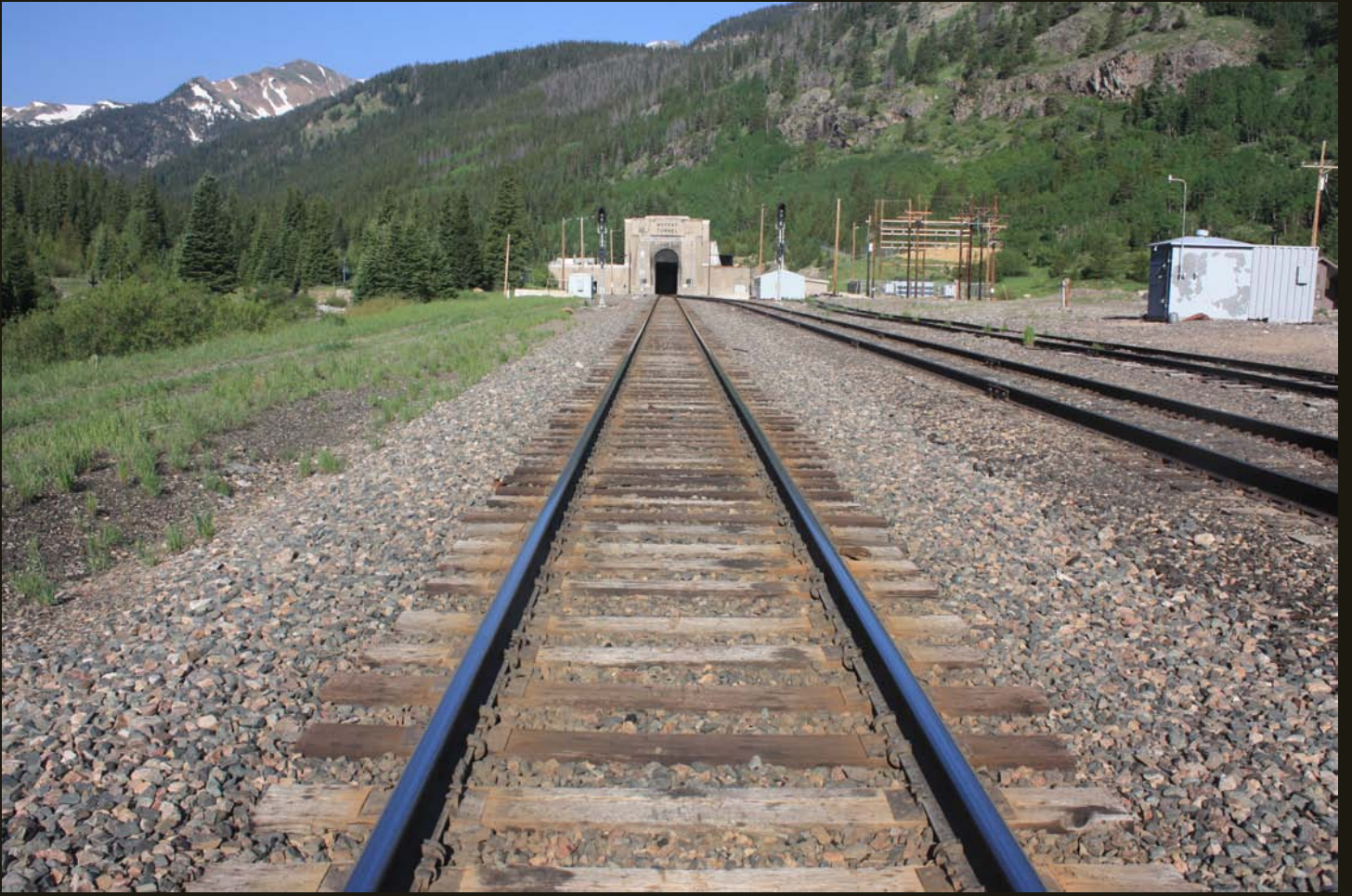
The East Portal of the Moffat Tunnel. The structure to the left of the tunnel is the outlet of the Moffat Water Tunnel.
