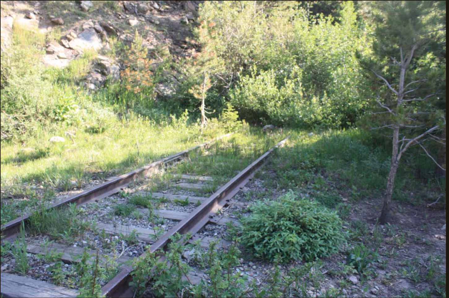
The end of the wye, same location as the previous photo, on the grade of the DNW&P Rollins Pass Route.
