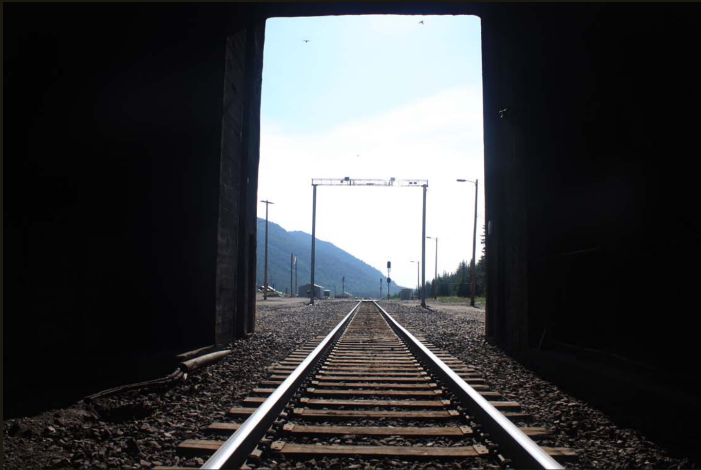
View out of the East Portal of the Moffat Tunnel.
