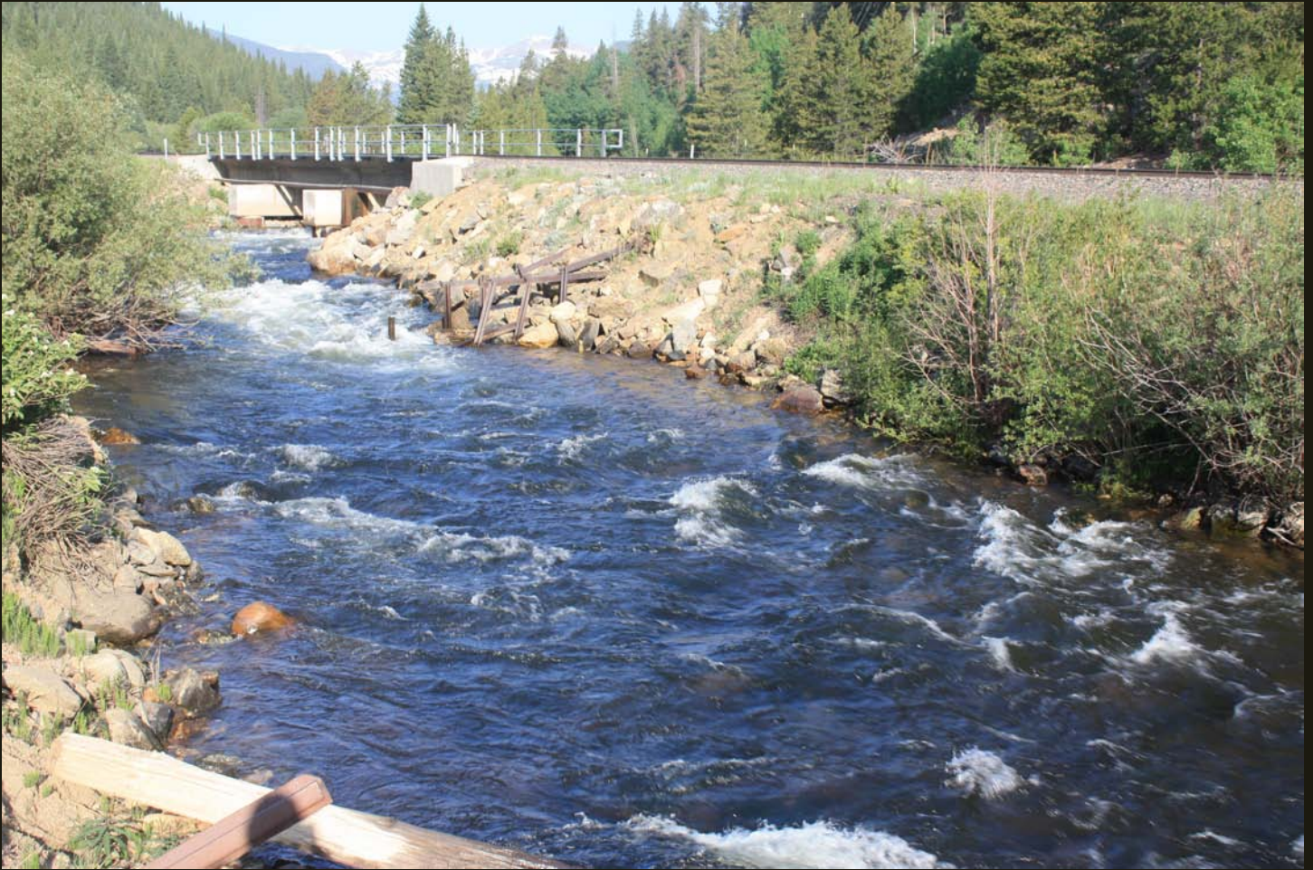
Westward view of the DNW&P (now Union Pacific) line 5 miles east of the Moffat Tunnel East Portal, where the tracks cross to the south side of Boulder Creek.
