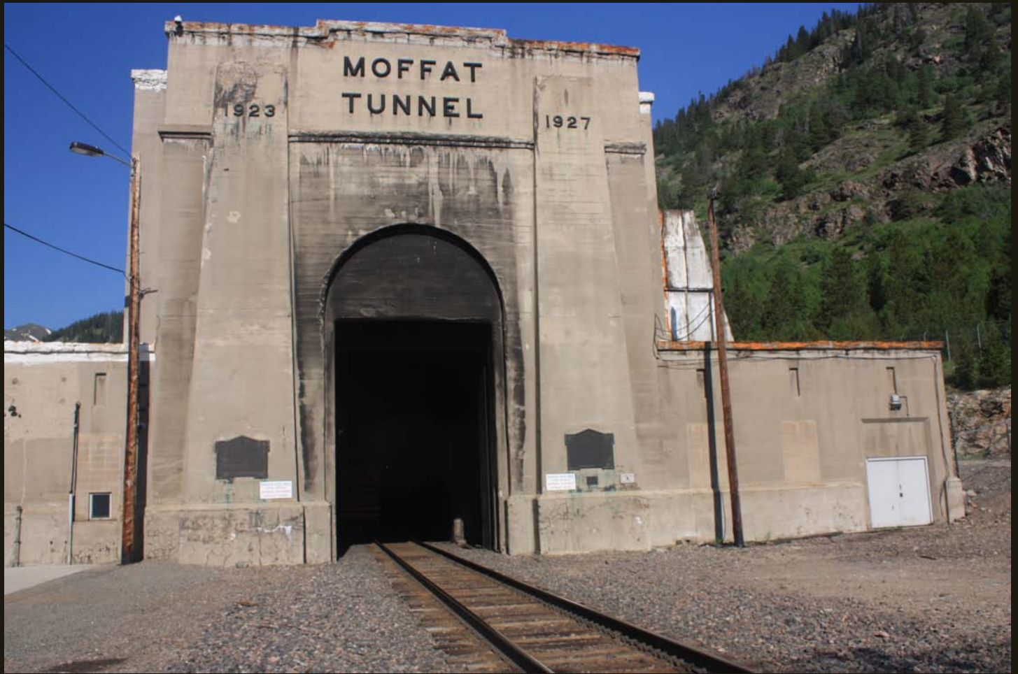
The East Portal of the Moffat Tunnel.
