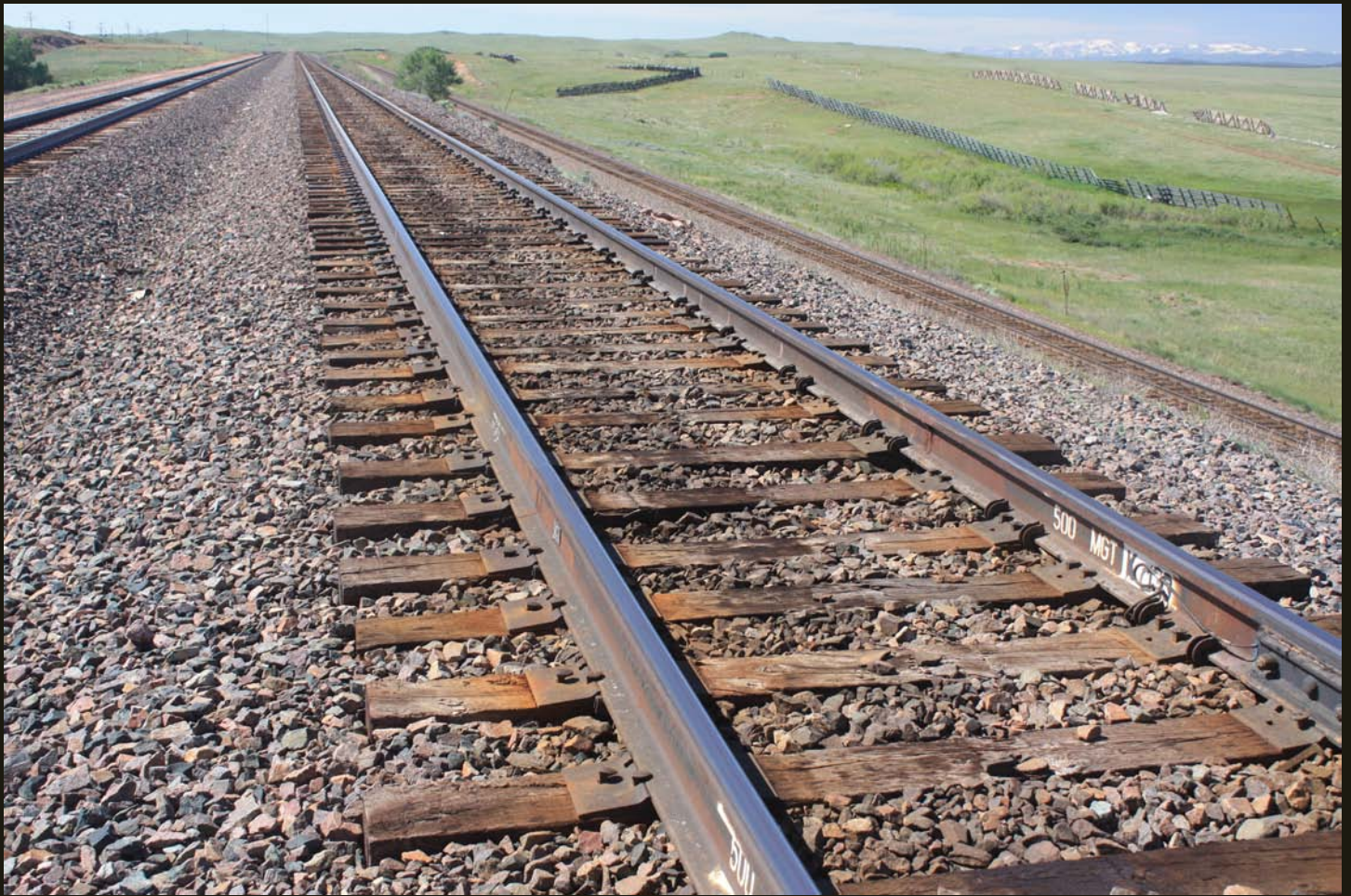
Eastward view of UP triple track. The right (south) track is the 1901 re-alignment and descends and follows the 1868 grade to Laramie. The two tracks on the left follow a new grade completed in 1917 from this point to Laramie.
