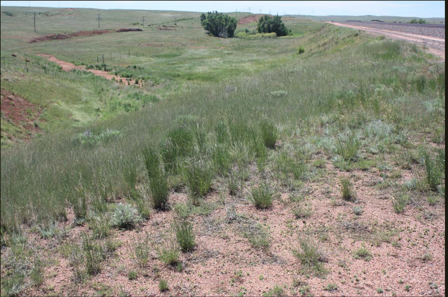
Near the same location as the previous photo, abandoned grades are visible north and east of current tracks. In this southeastward view, the active triple track is on the right, and an abandoned grade for a siding on the left is marked by a cut slope.
