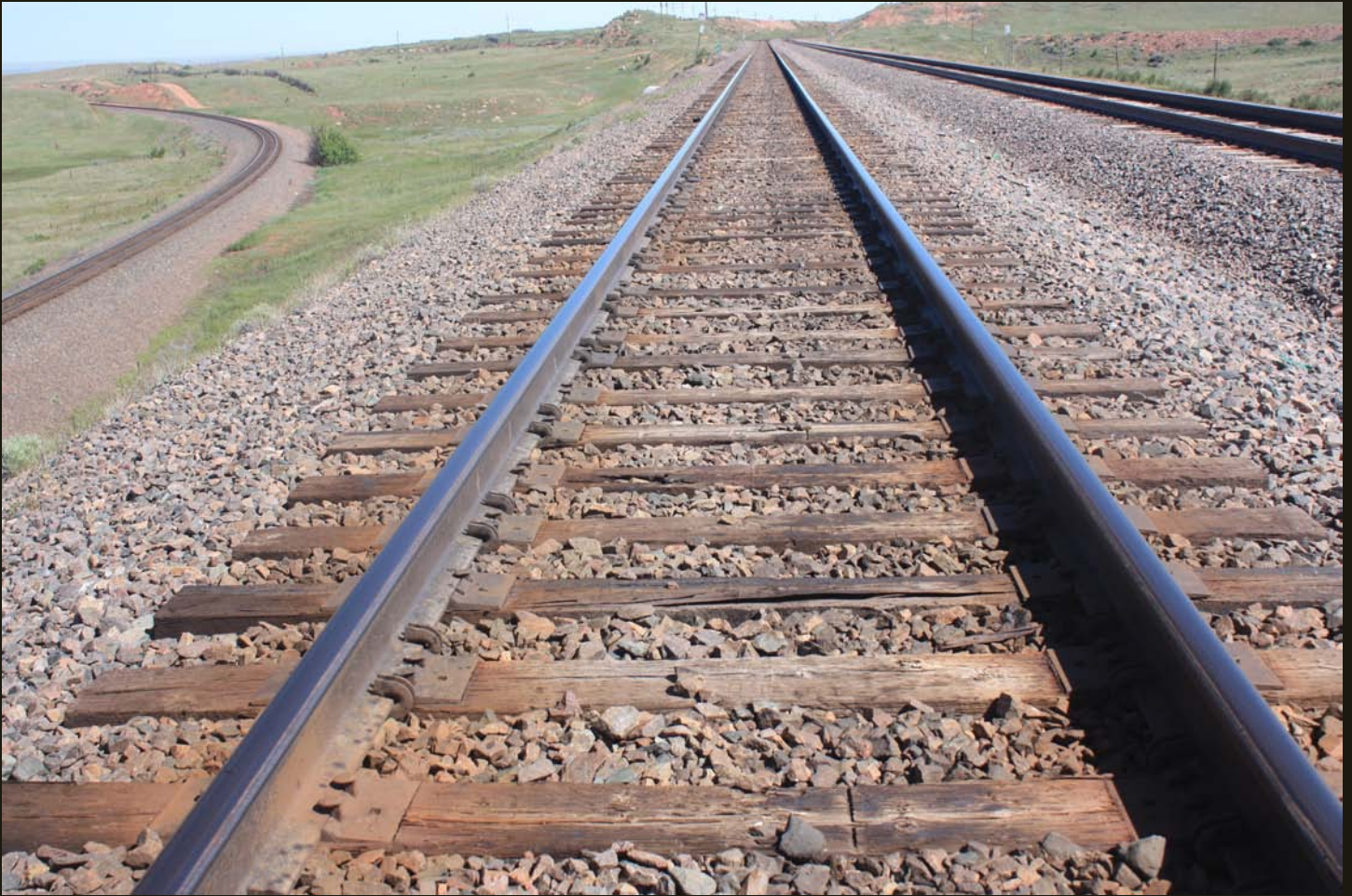
Westward view of UP triple track at same location as above. The left (south) track is the 1901 grade, which descends and joins the 1868 grade which it follows to Laramie. The two tracks on the right follow the 1917 grade to Laramie. The bare dirt area in the upper right corner of the photo is the abandoned 1868 grade, which crosses the double track and joins the single track in the upper left corner of the photo, just beyond where the single track disappears into a cut.
