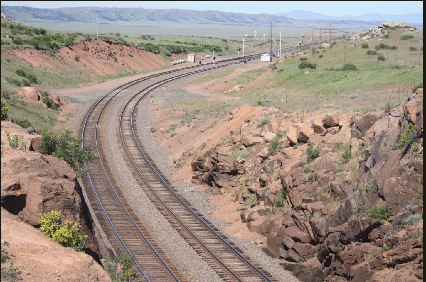
Eastward view near east portal of the Hermosa Tunnel on the 1901 grade. Note that beneath the signal, there are switches from each track to a third track in the middle.
