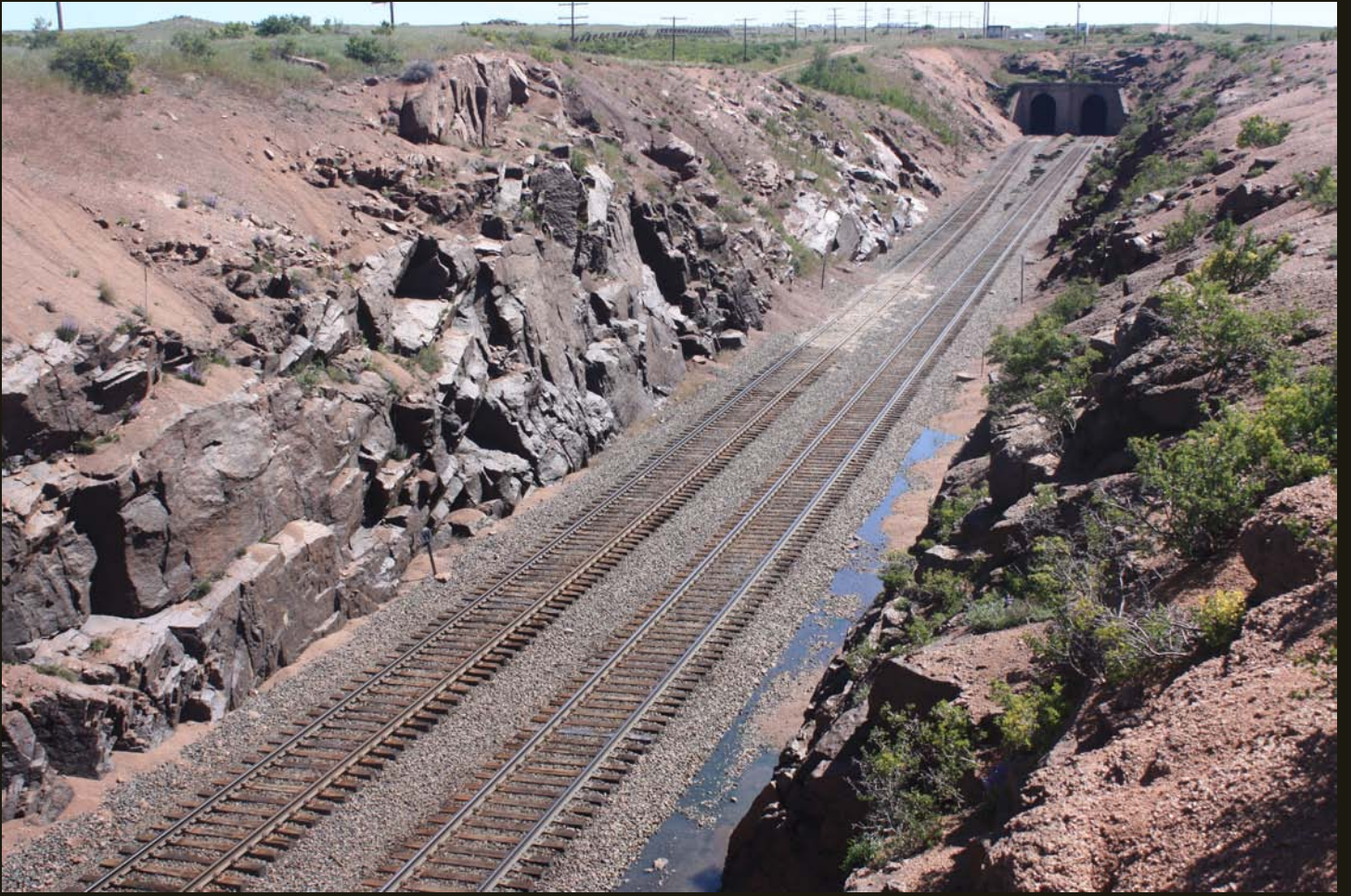
West portal of the Hermosa Tunnel.
