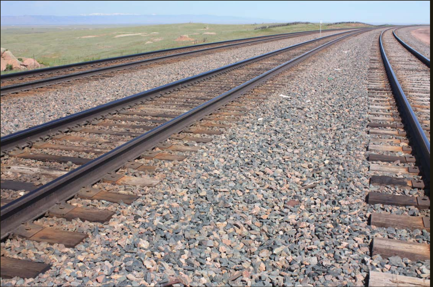
Westward view at about the same location as previous photo. The left (south) track starts to descend in the distance and follows the 1868 grade to Laramie. The two tracks on the right follow a new grade completed in 1917 from this point to Laramie.
