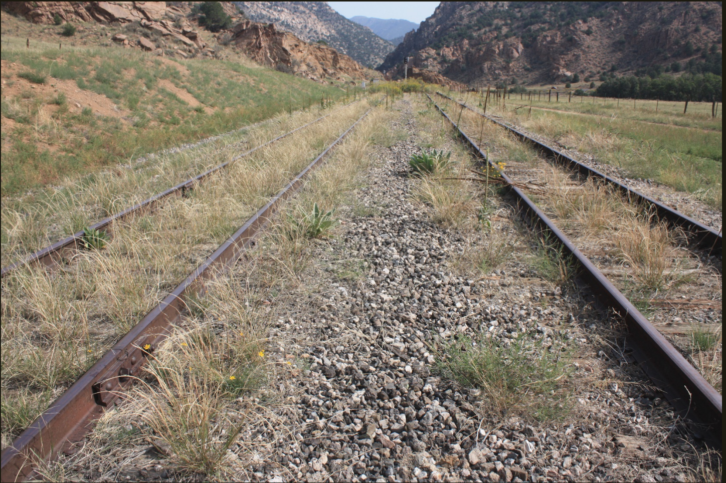
Northeastward view of the D&RG Leadville Branch (1880n) 1,000 feet southwest of the previous location. The Arkansas River is out of sight on the right and flows down the Arkansas River Canyon (center distance), entering the Royal Gorge 12 miles downstream.
