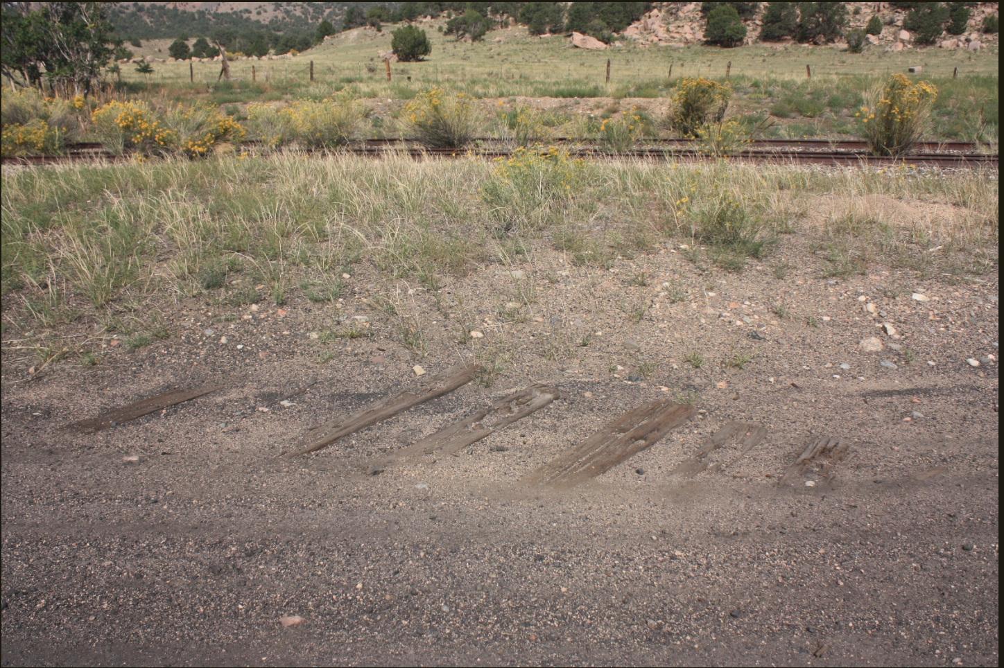
Northwestward view of the D&RG Leadville Branch (1880s) 700 feet southwest of the previous location. The ties in the foreground are the southwest branch of a wye, presumably for the D&RG Westcliffe Branch (1900).
