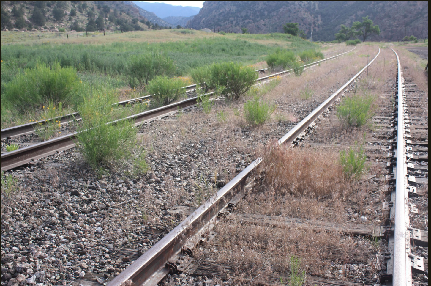
Northeastward view of the D&RG Leadville Branch (1880n) 1,000 feet southwest of the previous location. The mainline is on the left, the siding for the junction with the D&RG Westcliffe Branch (1900) is on the right, and the two large trees just beyond where the tracks disappear is the location of the presumed wye for the Westcliffe Branch. The flat topography used by the railroad is the floodplain of the Arkansas River.
