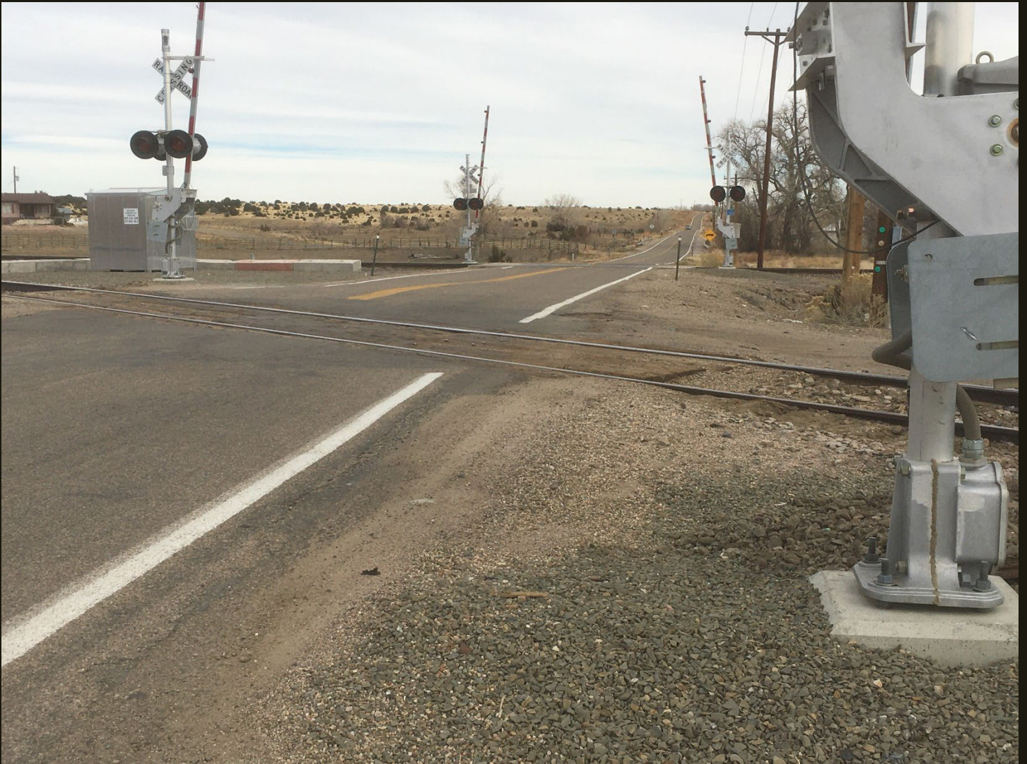
Northeastward view of Colorado Highway 239 a few steps west of the previous location. The highway crosses the original UPD&G (1895) in the foreground and the ca 2000 re-alignment beyond.
