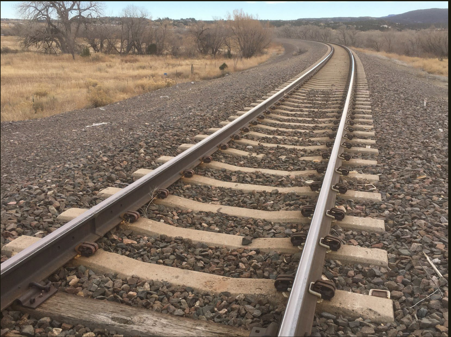
Southeastward view of the ca 2000 re-alignment of the UPD&G (1895) a few steps from the previous location. This line continues its 180-degree curve and just past the bend crosses the P&AV (1878) and the Purgatoire River to head northeastward and back onto the DT&FW (1888) alignment.
