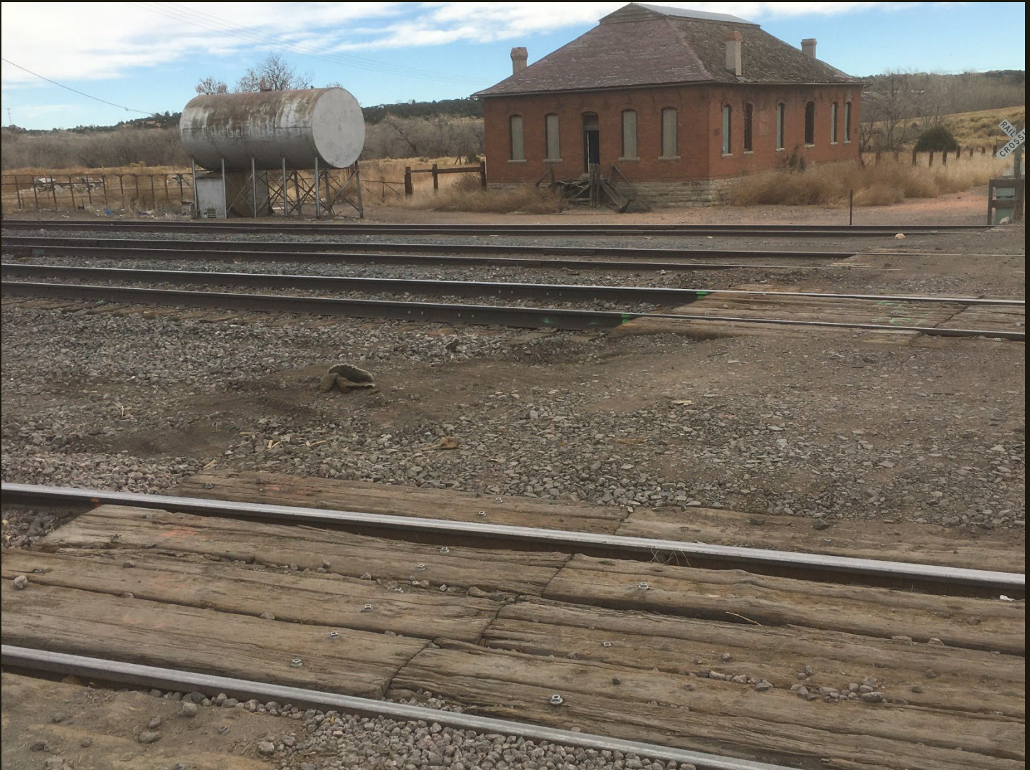
Southeastward view a few steps northwest of the previous location. The track in the foreground is the original alignment of the UPD&G (1895) and beyond it are the P&AV (1878) mainline and the two sidings visible in the previous photo. The brick building appears to be a depot, presumably AT&SF, but I could find no information on this building.
