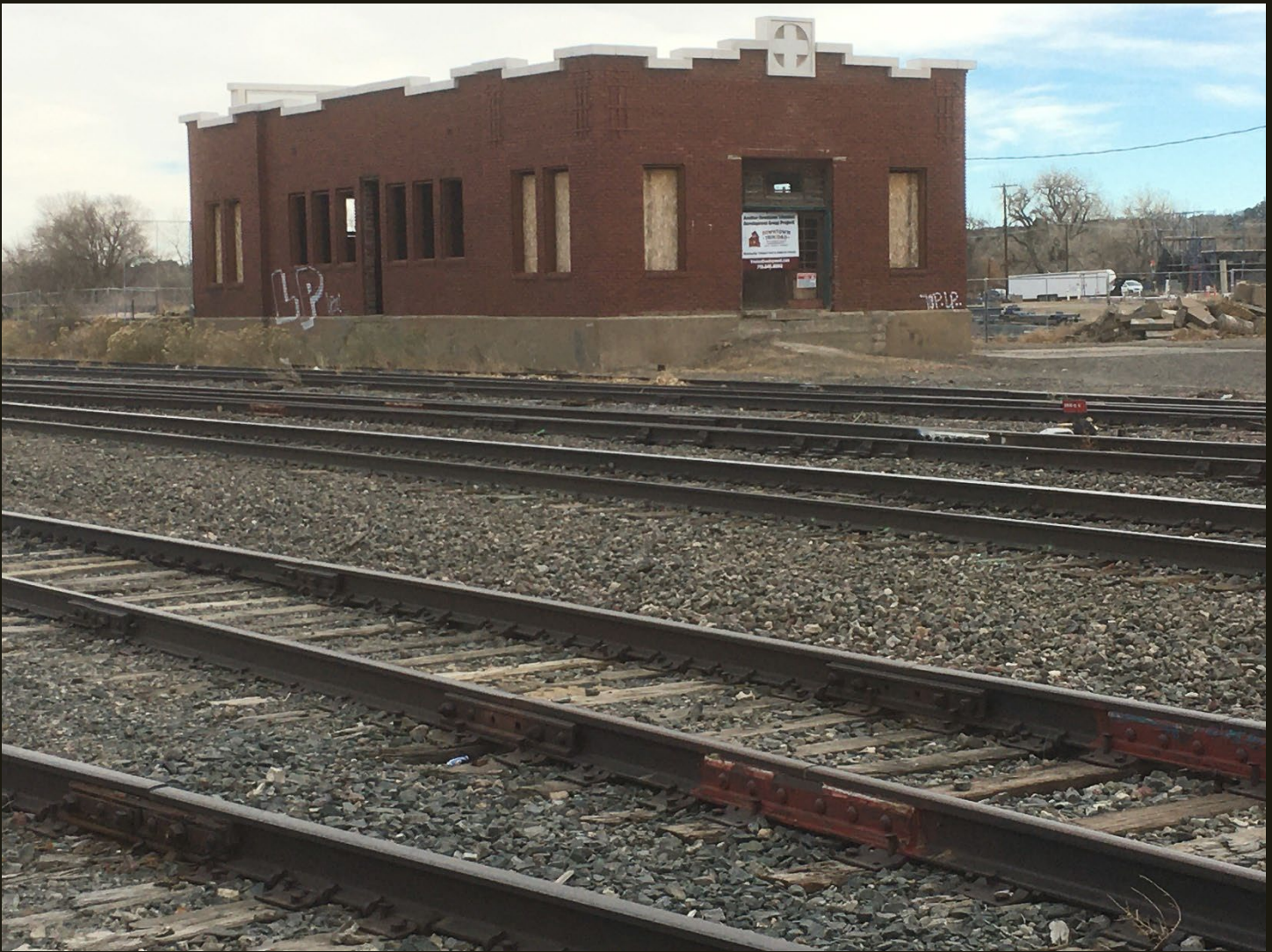
Closer view of the AT&SF Trinidad depot. The cross-in-a-circle logo identifies this as an AT&SF depot, but I could find no information whatsoever on the history on this building.
