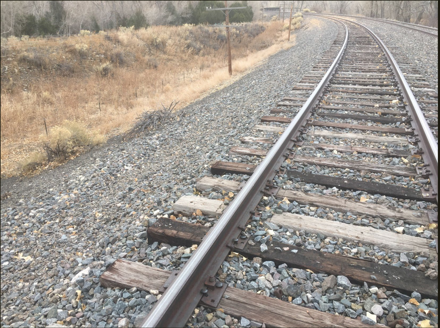
Southward view of the P&AV (1878) at the same location as previous. The 45 degree curve to head south toward Raton Pass continues and the bridge over the Purgatoire River is visible in the distance. Note the berm on the left; this could be an earlier alignment of P&AV (1878) or just a levy to contain the Purgatoire River.
