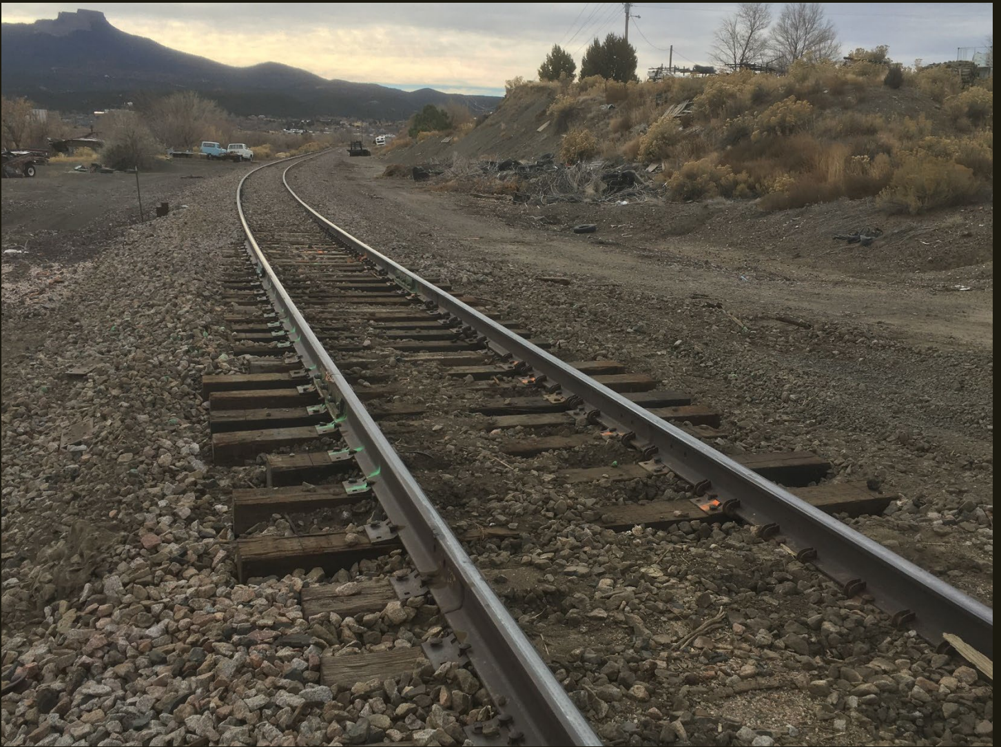
Southward view of original UPD&G (1895) at the same location as previous. This line heads into Trinidad in the distance.
