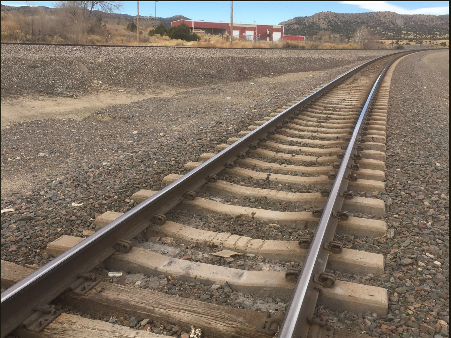
Now we are 400 feet southeast of the previous location looking northwest. The ca 2000 re-alignment of the UPD&G (1895) is in the foreground and the original 1895 alignment runs across the image in the distance.
