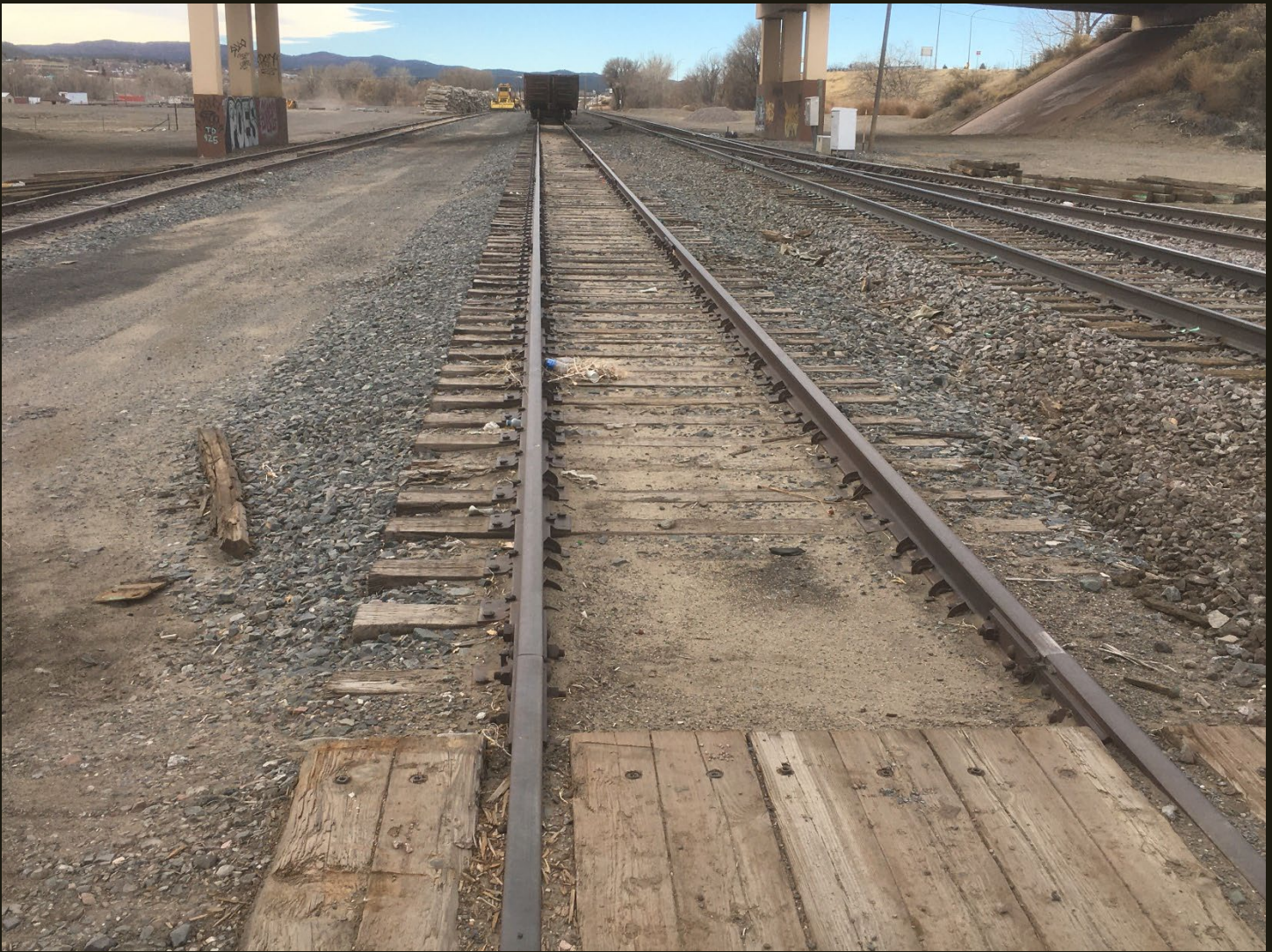
Southwestward view of the P&AV (1878) a few steps south of the previous location. Buildings in Trinidad are visible in the distance. The parked railcars are on the first siding, which is the track in the immediate foreground. The track on the far right that merges with the P&AV (1878) mainline via a switch is the UPD&G (1895), which in a 1988 (and earlier) topo map is shown to cross, not merge with, the P&AV (1878). 1,000 feet in the distance is a switch to the continuation of the UPD&G (1895) to the left (south) of the P&AV (1878).
