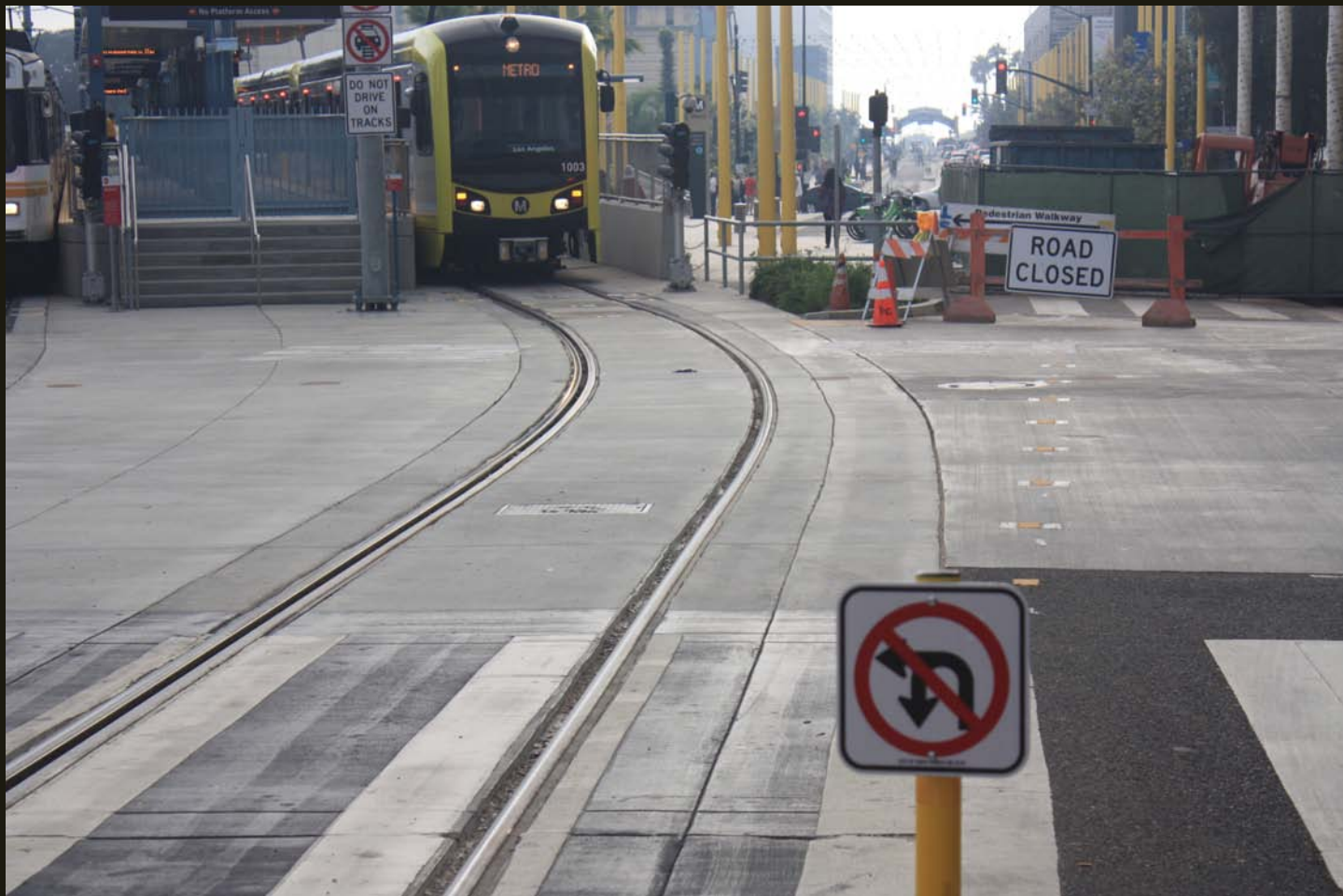
Westward view at Santa Monica, same location as previous. The curved track is a new alignment to today's Metrolink Station and the end of track. The archway in the distance is the entrance to today's Santa Monica pier; the original wharf was a little to the right (north) of the current pier.
