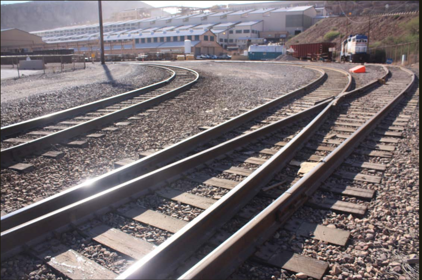
Closer view of the MS at the Morenci processing plant and splitting of the line near the end-of-track.
