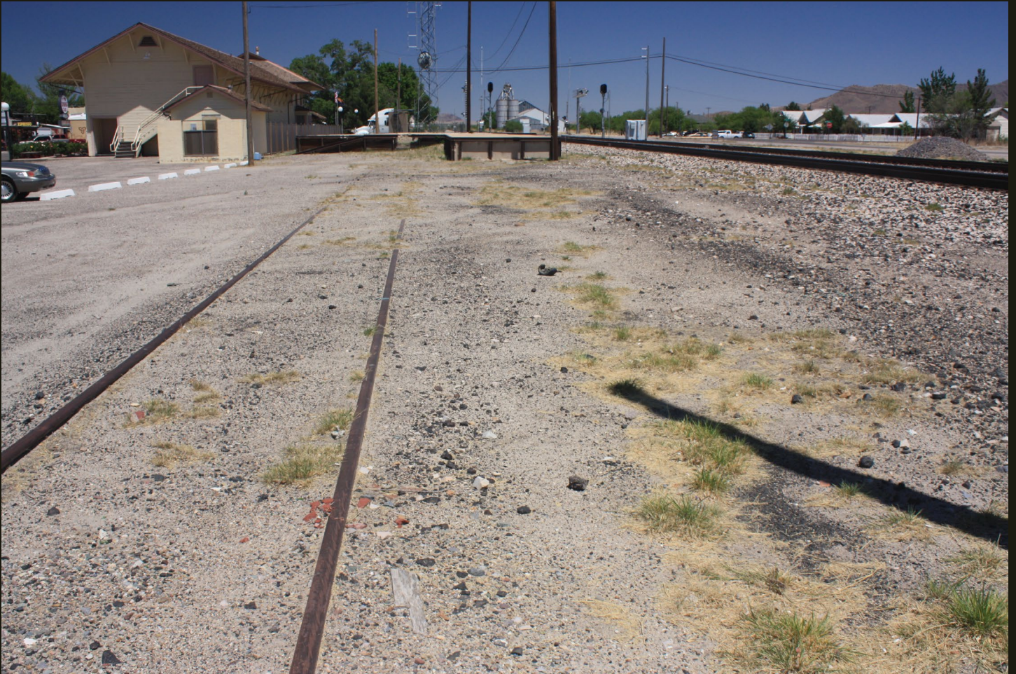
Northeastward view from the other side of the Willcox Depot (upper left), showing an old spur to a loading platform. The double-track SP (now UP) mainline is on the right.
