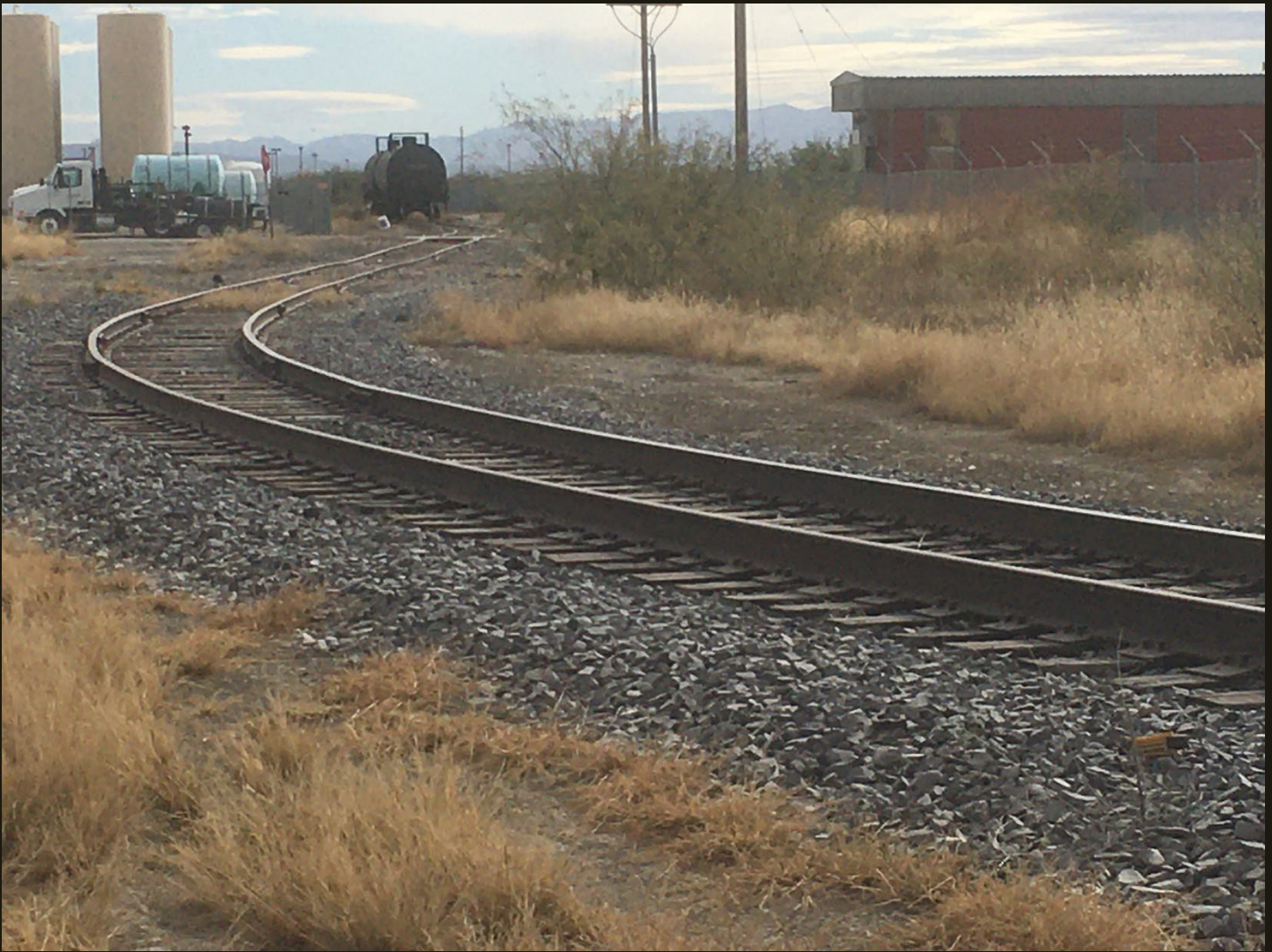
Eastward view of the industrial spur, same location as previous. There is no obvious reason for this jog in the track, which may have something to do with the M&W (1915) junction reconfiguration for the spur.
