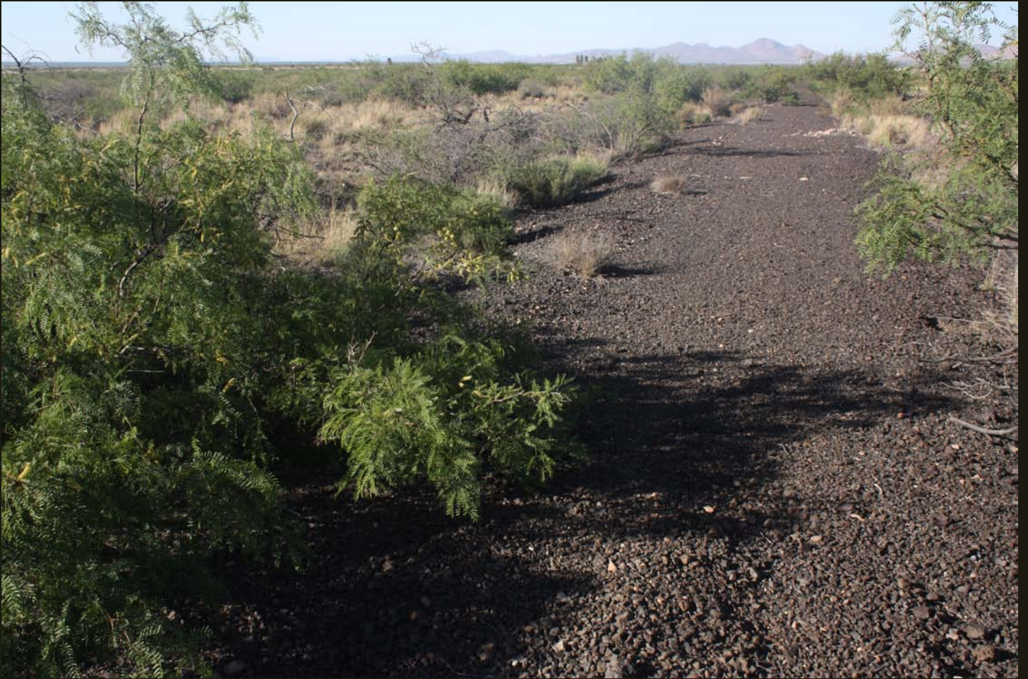
Northeastward view of the EP&SW (1902) about 25 rail miles northeast of the first photo and 3 miles northeast of the former whistle stop of Apache. Note the black slag ballast typical of EP&SW grades.
