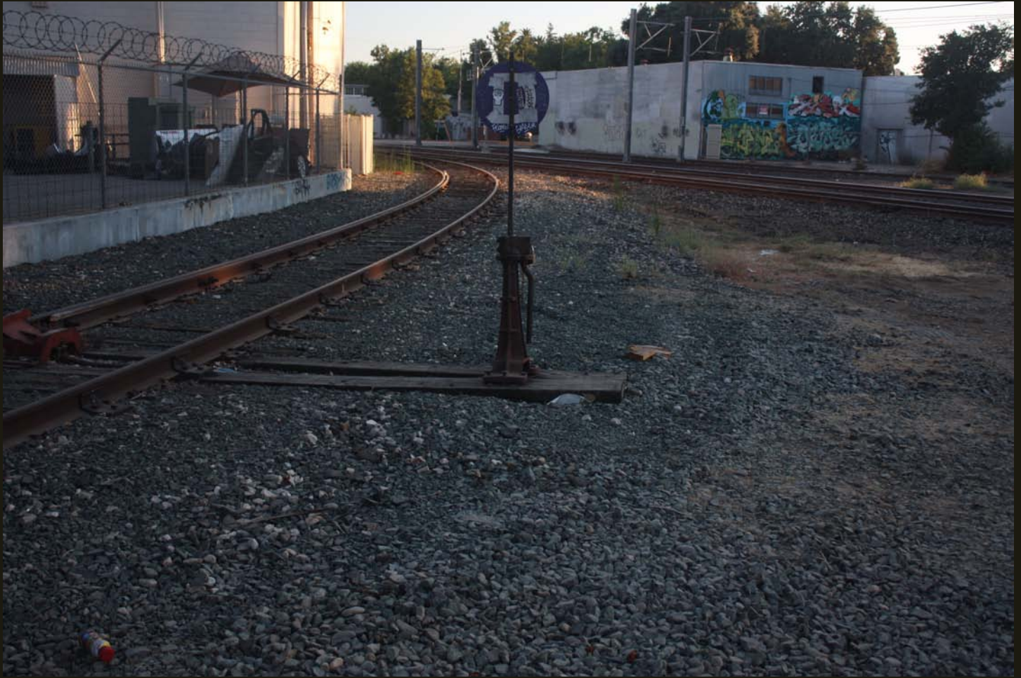
Southwestward view a few steps from the previous location showing the connection between the WP (1909), which is the straight track in the distance, and the SV alignment, which is behind the viewer.
