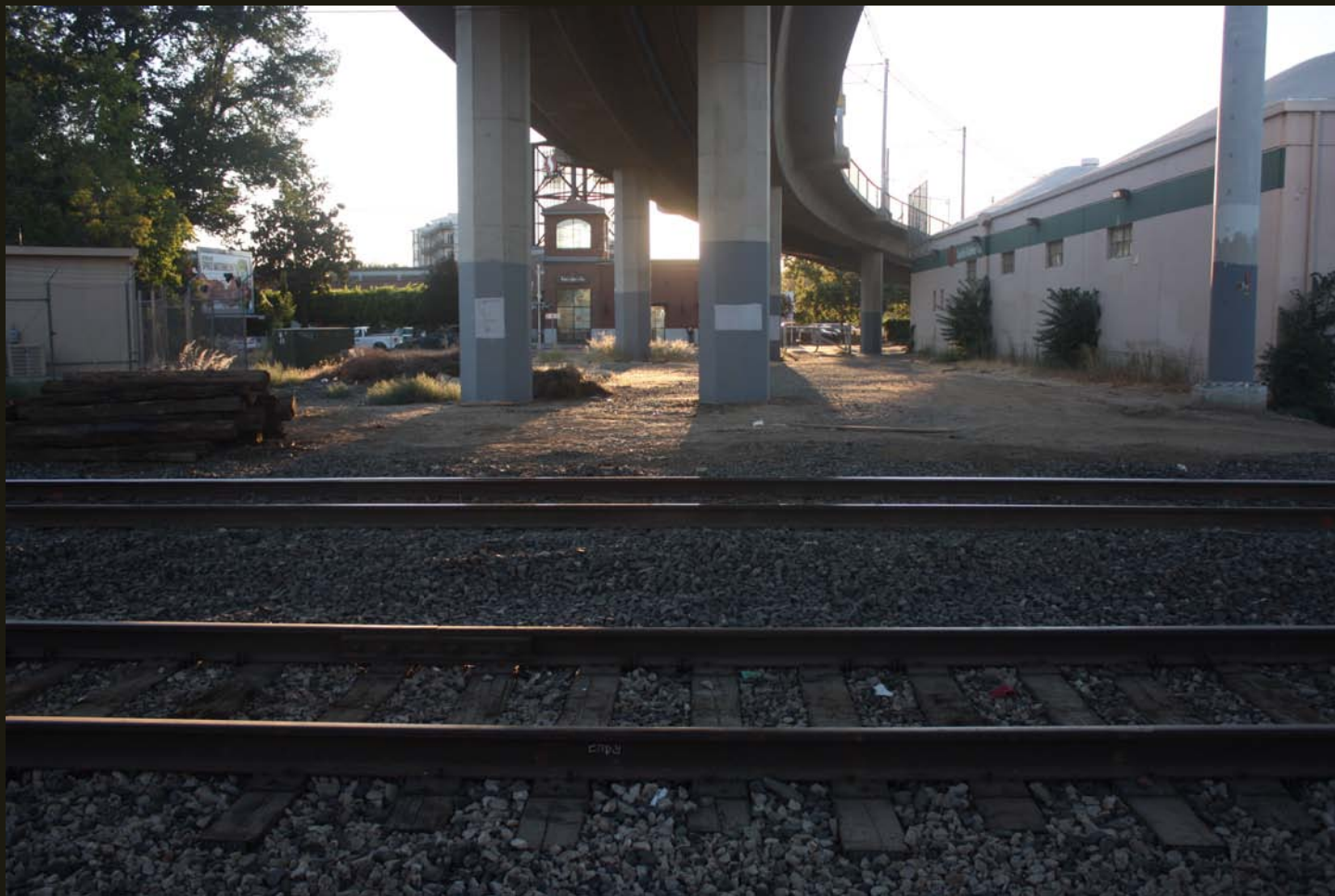
Westward view of the SV alignment, 1,300 feet east of the previous location between 19th and 20th Streets; note the same red brick building as in the previous photo. The SV/S&P/SP/UP tracks are gone. The tracks in the foreground are the Western Pacific (1909) (the second WP), where once a grade crossing existed. The overpass is the Gold Line commuter line, which curves to the right (north) to leave the SV alignment and parallel it to the west (as seen on the photo before the previous photo).
