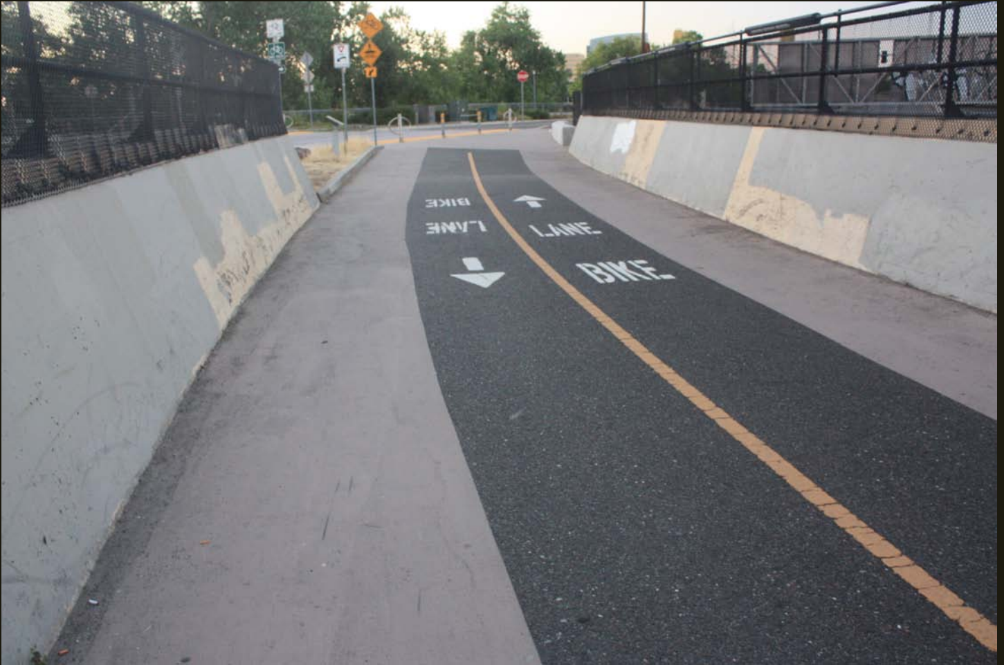
Northwestward view of the SV (1856) alignment, now a bike path. This is the middle of the curve where the SV left the Sacramento River and turned east-southeastward down R Street. This is a former railroad bridge over Interstate 5, which carried trains until about 2000.
