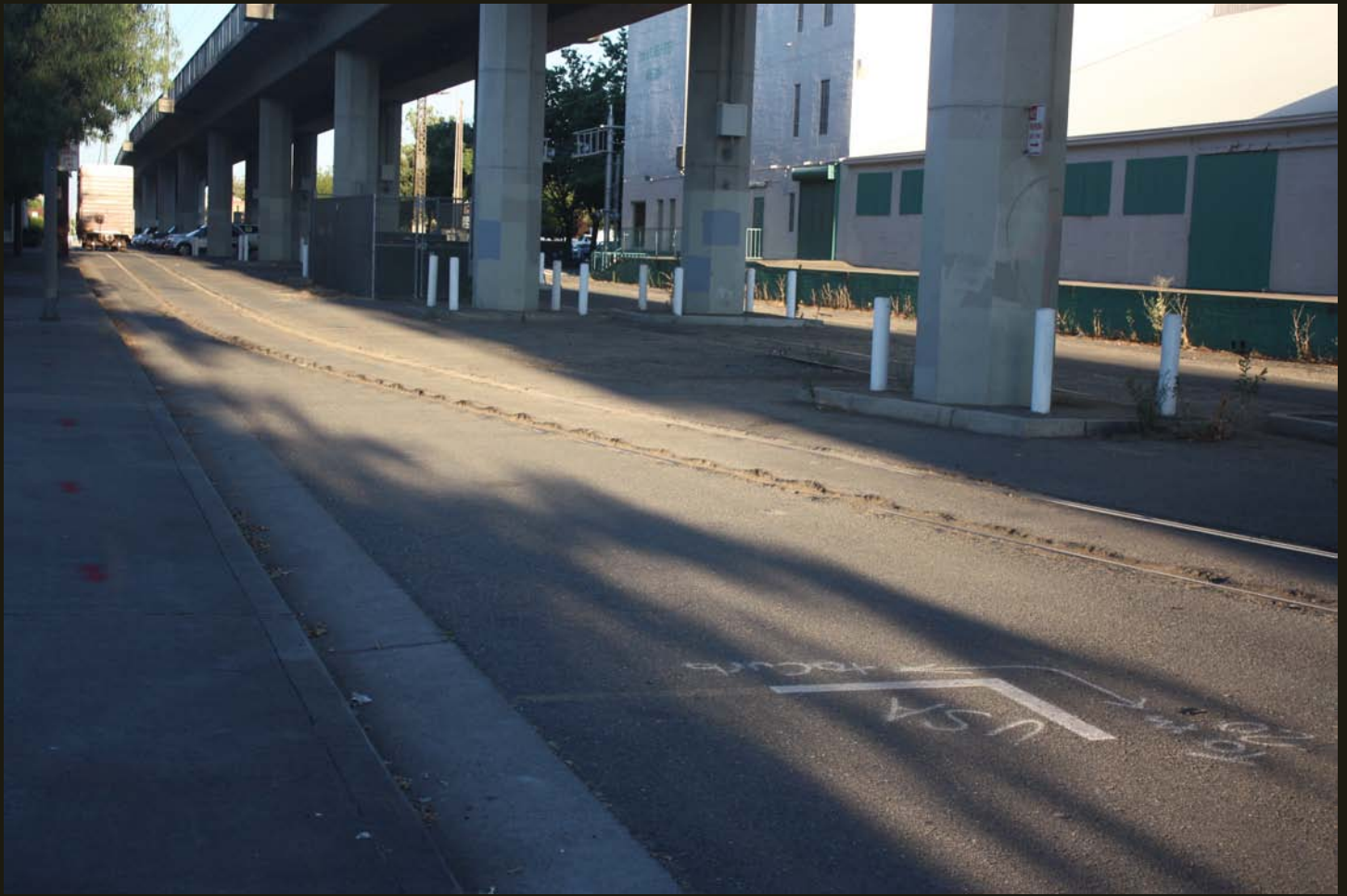
Southeastward view a few steps north of the previous location, showing the active siding with a stored box car, the SV/S&P/SP/UP mainline under the concrete pillars of the Gold Line, and an old siding along a loading platform on the other side of the pillars. The box car is at 21st Street and the siding it's on continues to 23rd Street, where a current or recent customer is located.
