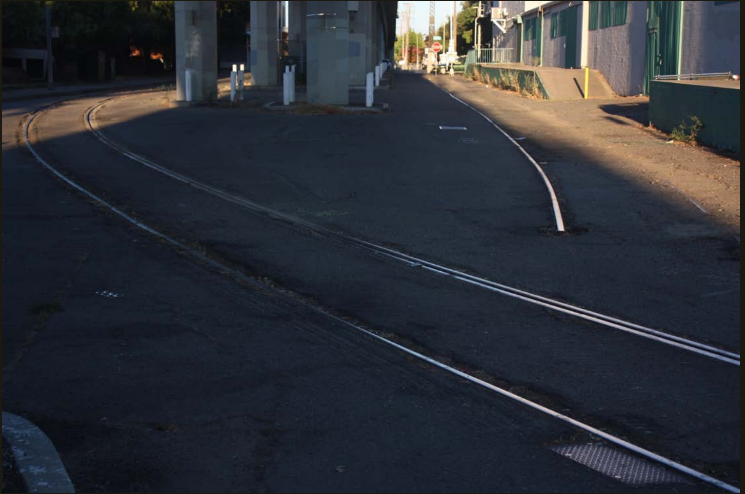
Northeastward view from the same location as previous, showing the connection between the WP (1909), which is behind the viewer, and the SV/S&P/SP/UP alignment. The concrete pillars support the Gold Line and are built right on the SV/S&P/SP/UP mainline alignment; an old siding is to the right (south) of the mainline and an active siding is to the left. The pavement is R Street.
