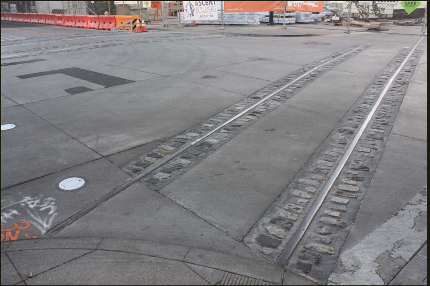
Northeastward view of the SV/S&P/SP/UP trackage on R Street at 17th Street, one and a quarter miles east-southeast of #2. There are numerous spurs and switches preserved in the paved-in historic trackage; note two more tracks across the street. This must once have been an industrial area with numerous rail customers. The bricks look the same as those in the previous photo; my guess is they are re-used bricks that were recently placed into their current positions as part of the track preservation project because there is no place for the wheel flange.
