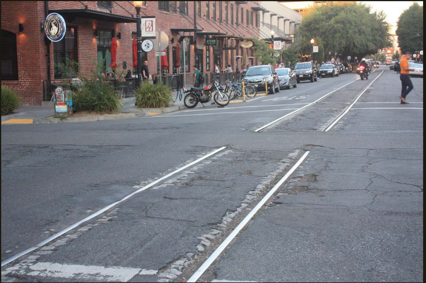
Eastward view of the SV/S&P/SP/UP trackage on R Street at 14th Street. Note the brick pavement under the asphalt, hinting at the long history of the railroad and of R Street.
