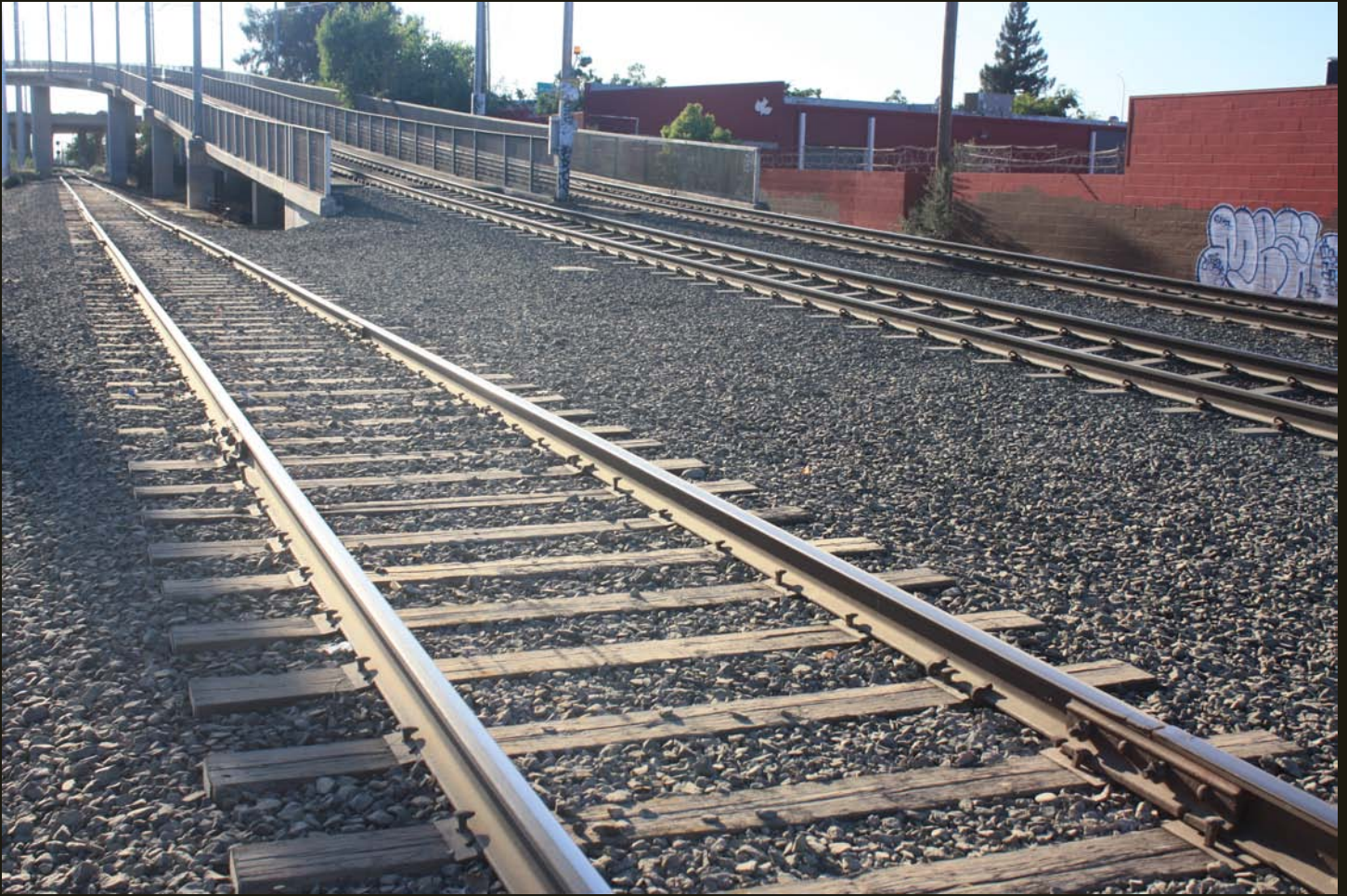
Westward view of the SV (1856) alignment, 500 feet east of the previous location. The track in the foreground is the original SV/S&P/SP/UP alignment. The two tracks on the right are the Gold Line overpass, which is today's representation of the SV-WP grade crossing at Brighton (location #4).
