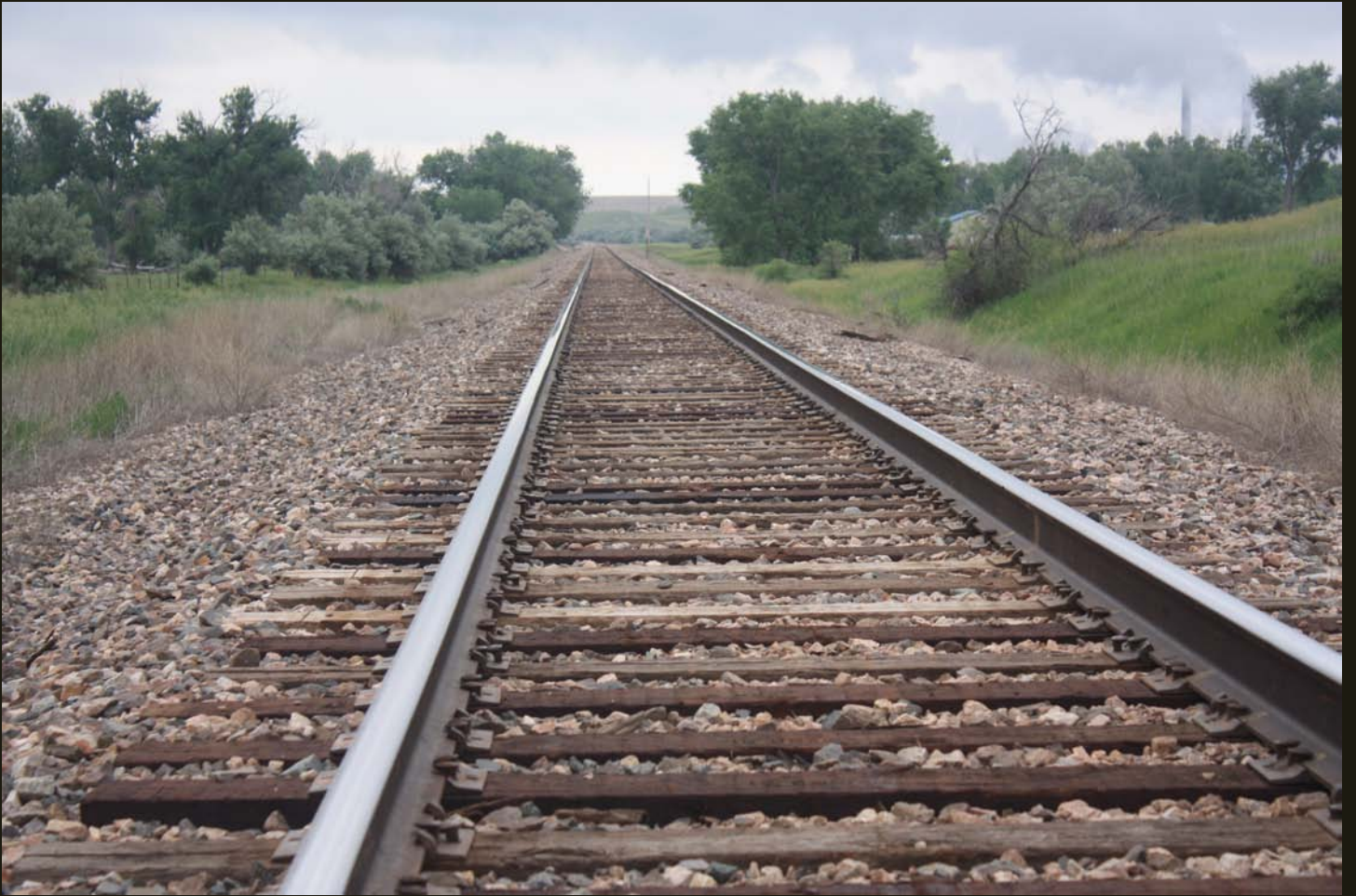
Eastward view of the 2-mile-long spur to carry coal trains to the power plant in the upper right distance.
