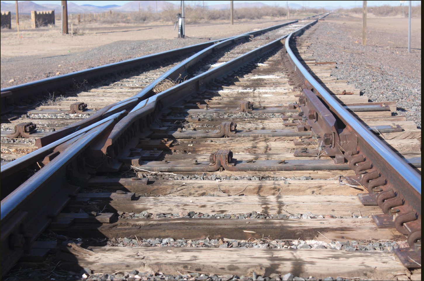
Northeastward view of the AT&SF's RGM&P (1881)(now SW) line from Rincon to Deming showing the switch for the siding in the previous photo.
