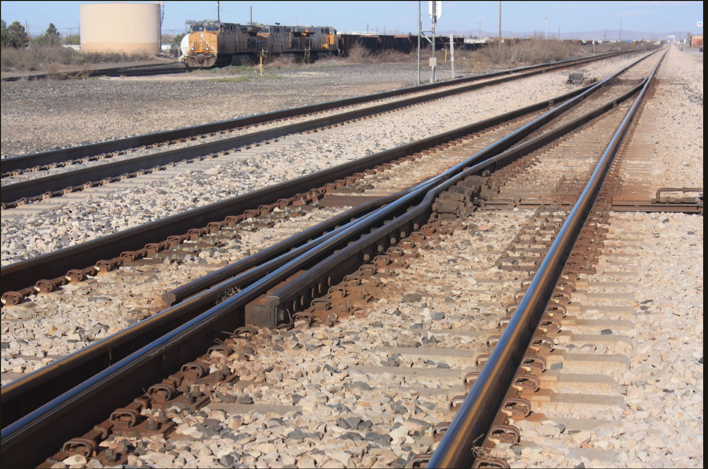
Eastward view of the SP Sunset Route (1881) 1.7 miles west of the previous location. The tracks in the foreground are the double-tracked SP Sunset Route (1881), now owned by Union Pacific, and a crossover track connecting the two tracks. The train on the left is on a siding that connects to the RGM&P (1881) 1.5 miles in the distance.
