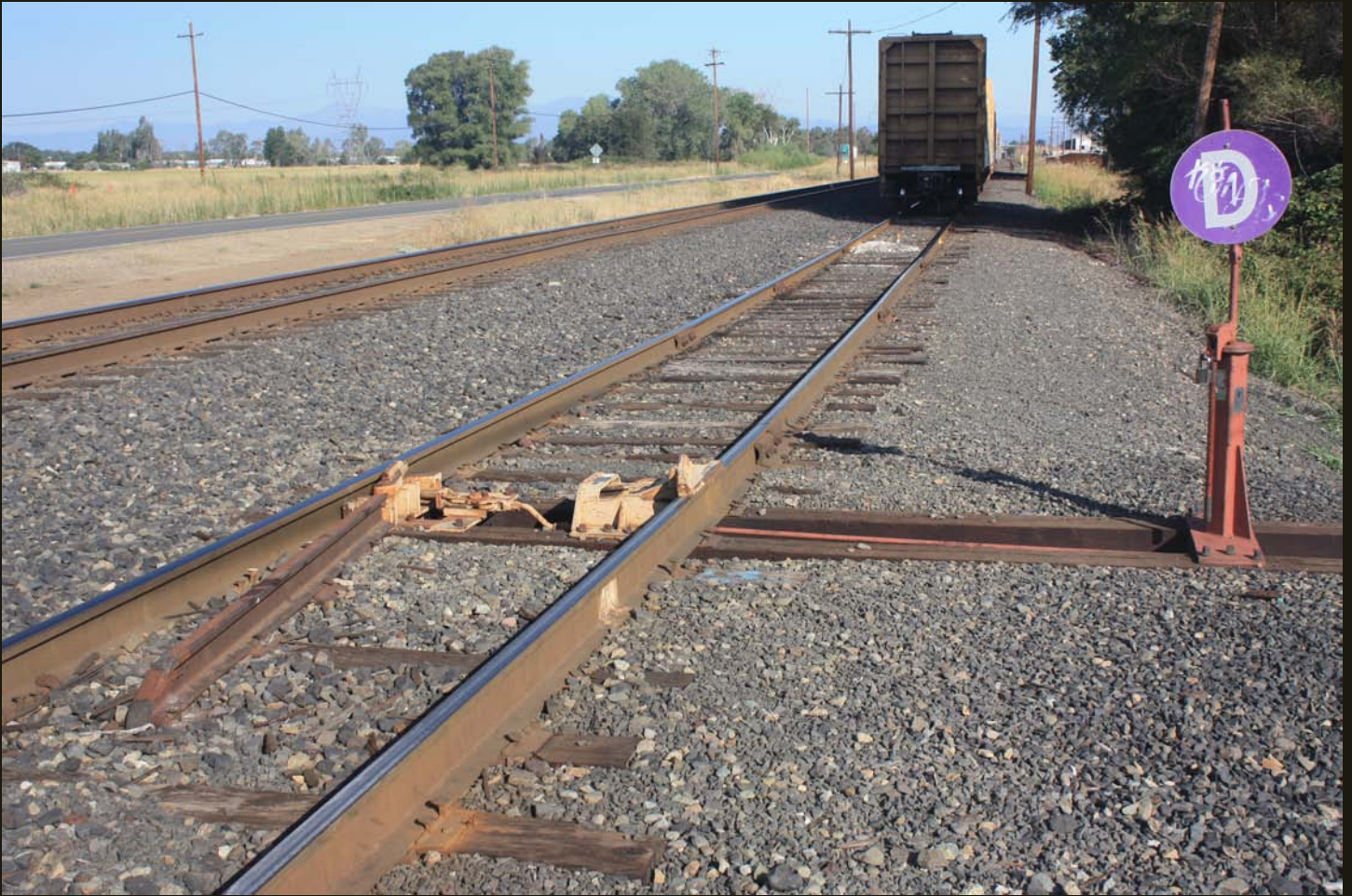
Northwestward view of the same "D" (derail) switch as in the previous photo. The A&BV switch is in the more distant of the two shadows to the right of the cars.
