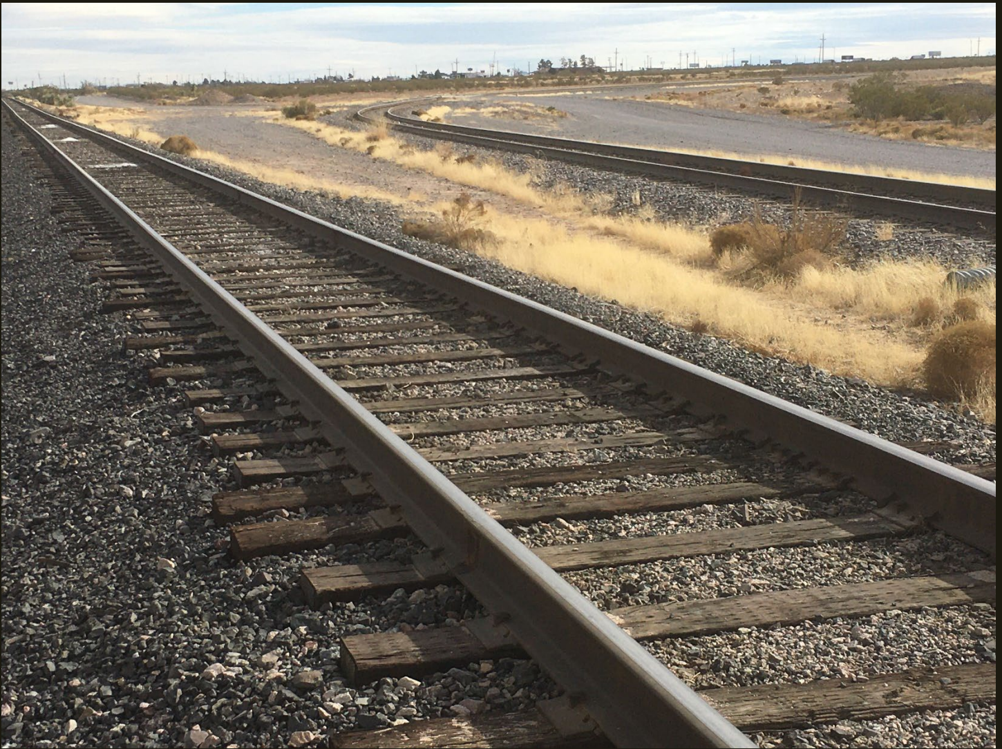
Eastward view of the C&SP (1883n) 1,000 feet west of the previous location. The track to the right is the west branch of the asymmetric wye and the track in the foreground, which we have been calling the C&SP (1883n) mainline, functions as the east branch of the wye.
