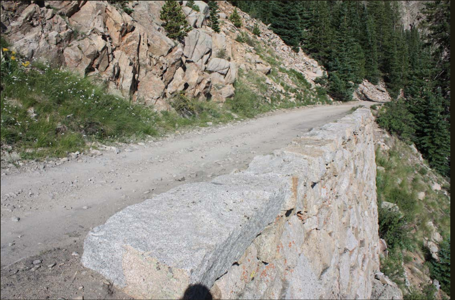
The rock retaining walls were built to last.
