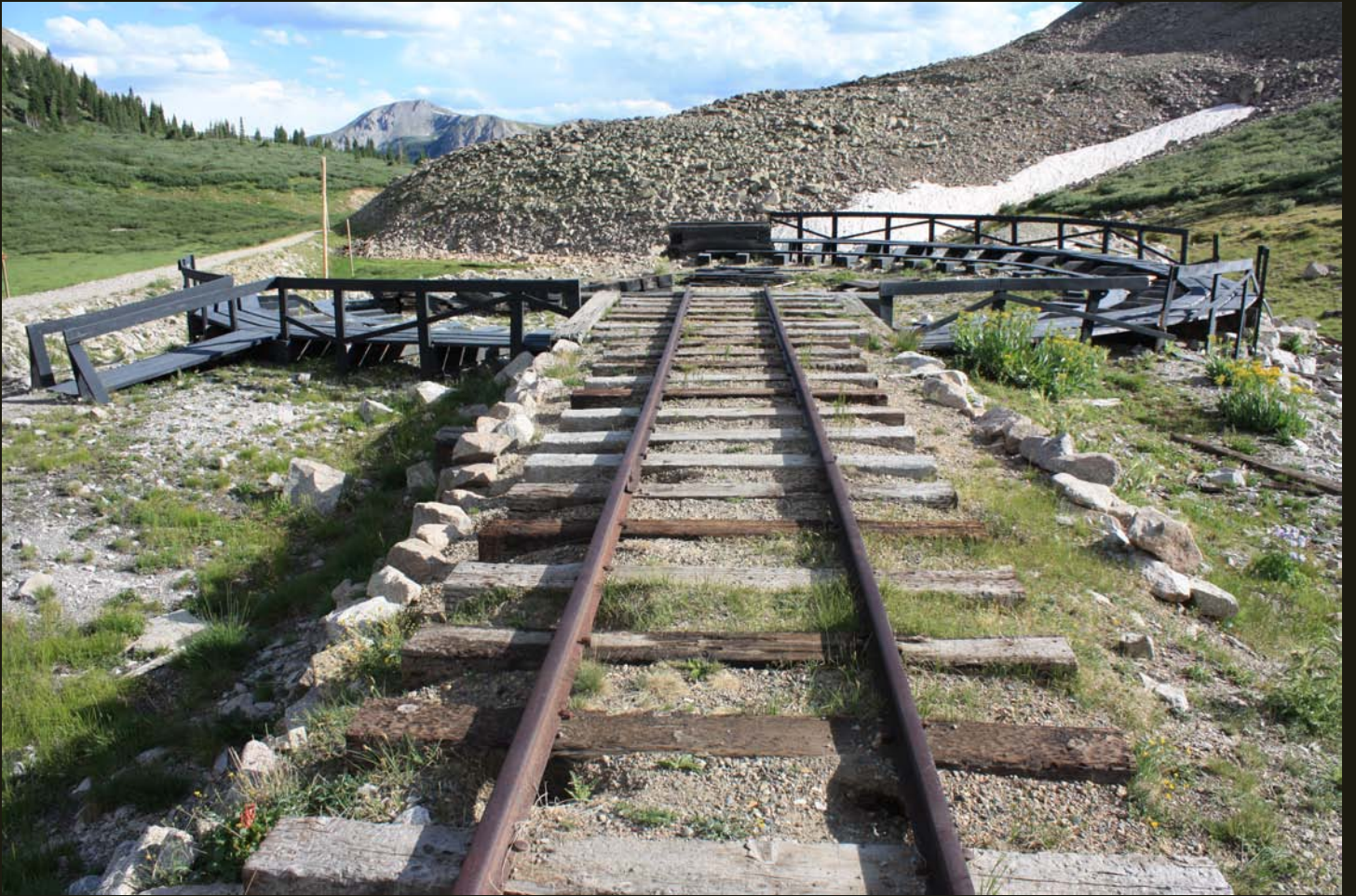
The Alpine Tunnel facility include a turntable to turn helper engines. The turntable is being restored.
