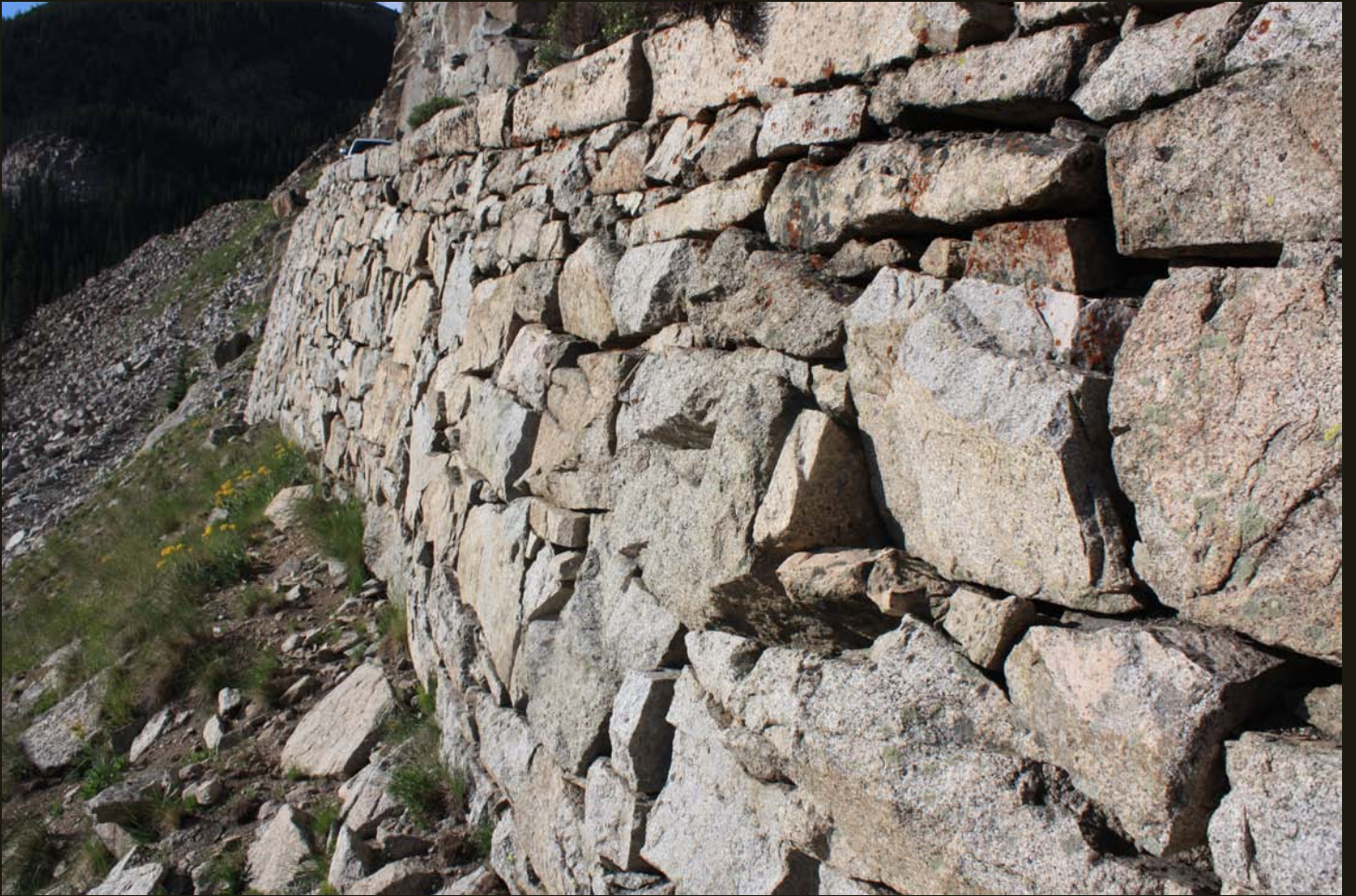
Detail of the retaining wall across the Palisade.
