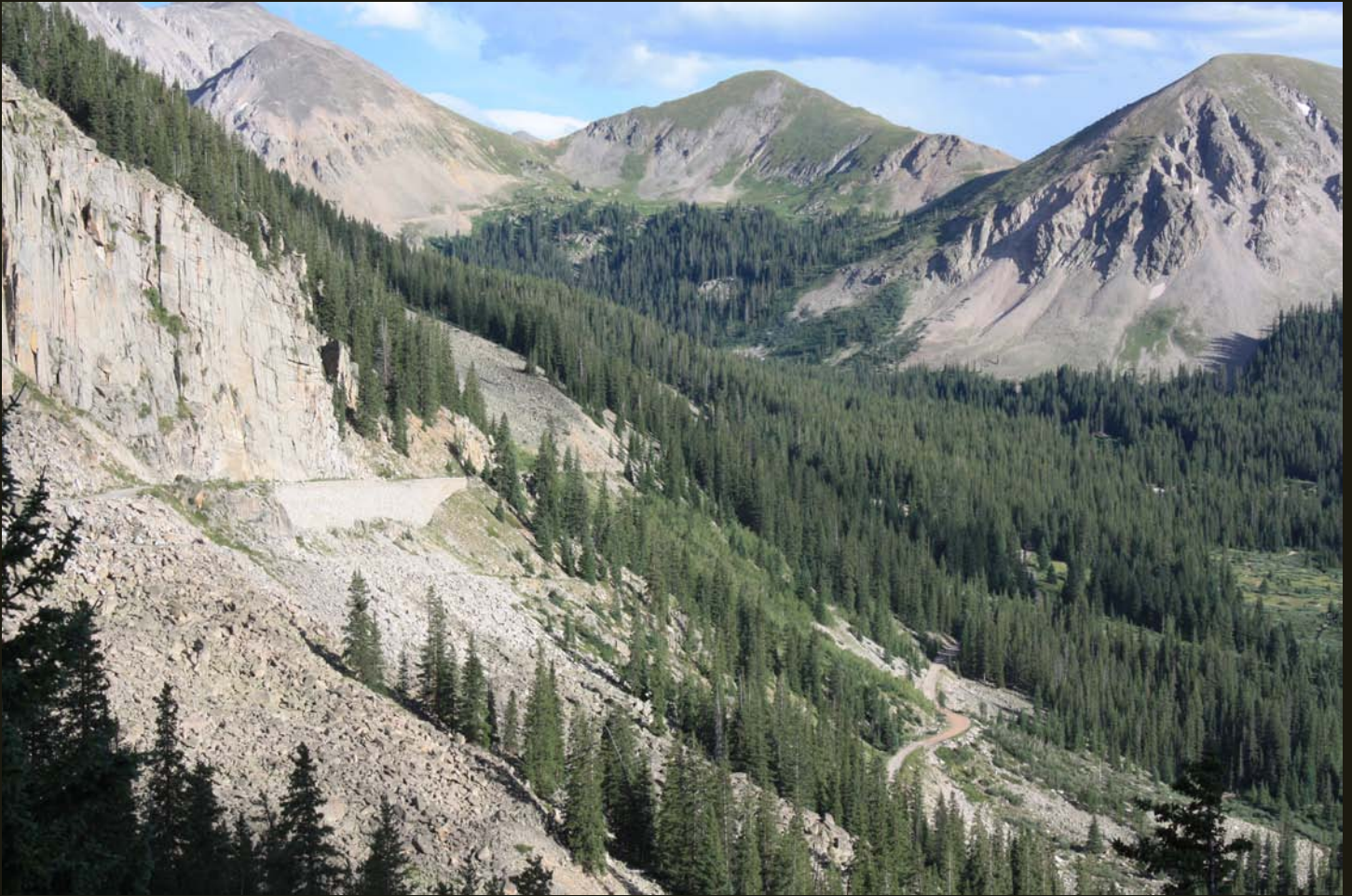
A rock retaining wall carries the DSP&P grade across the Palisade, a near-vertical granite escarpment, and a switchback out of sight in the distance, carries the grade lower down the slope. The switchback curve is the subject of the previous photograph.
