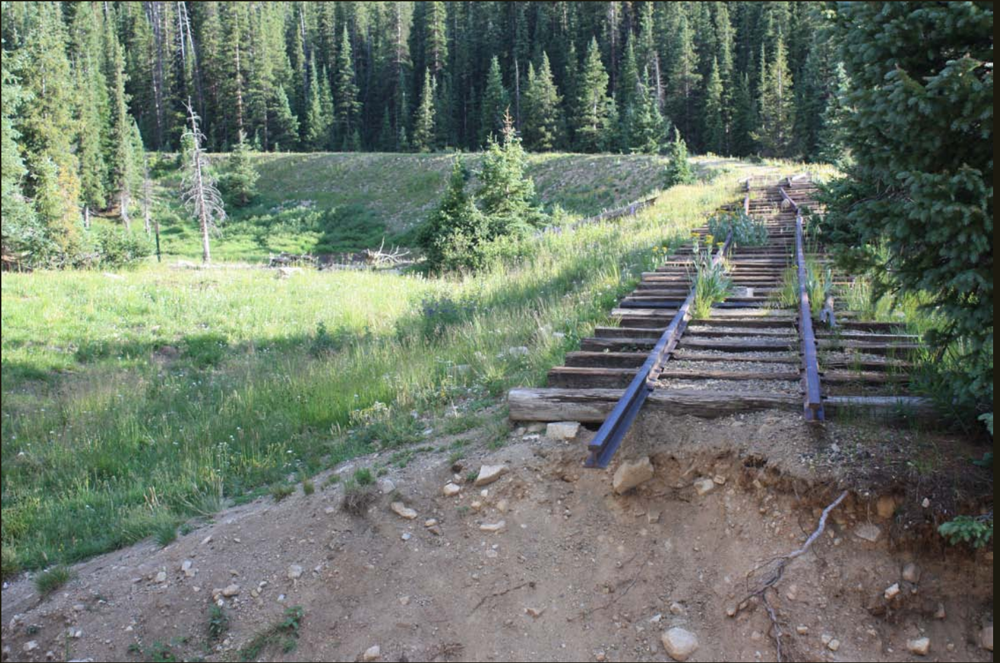
Fill and some track are present at a curve for a switchback needed to gain elevation toward the Alpine Tunnel. This is the only place the road leaves the railroad grade.
