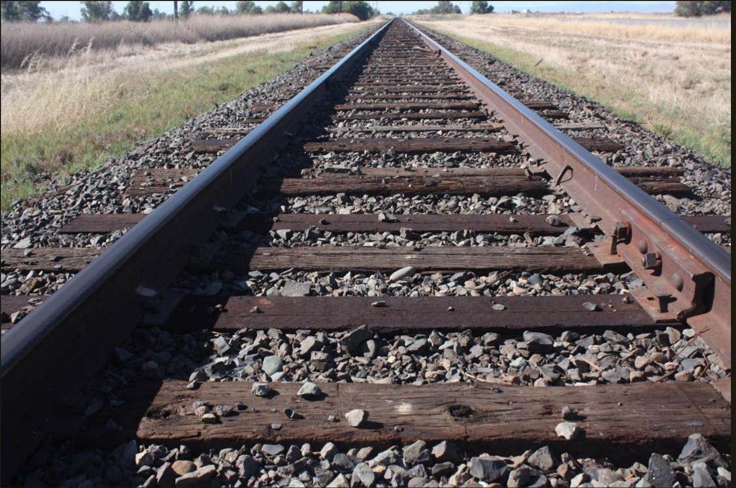
Southward view of the Northern Railway (now California Northern) at the same location as previous. Note the old bolted track; this was replaced with welded track father south.
