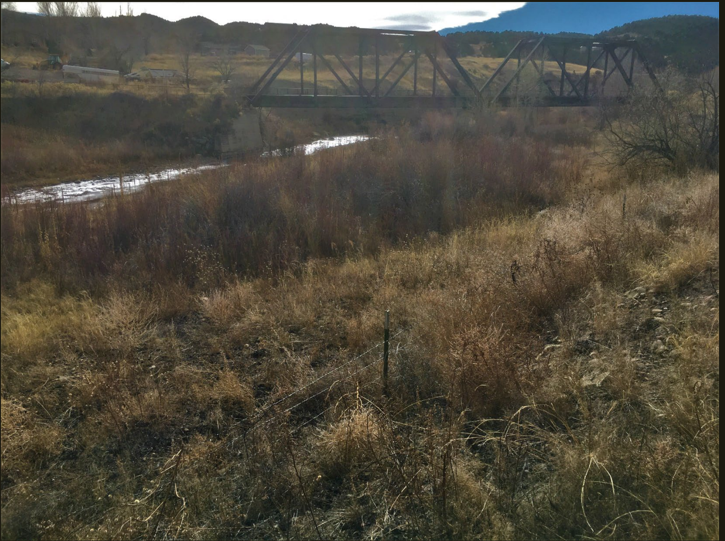
Southwestward view the same bridge over the Purgatoire River. This bridge is the most significant remaining feature of the C&W (1903).
