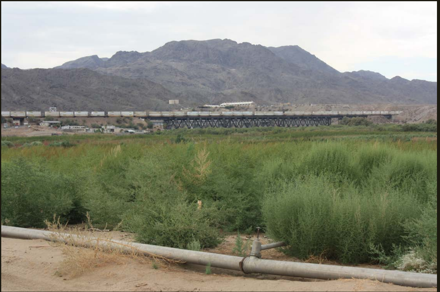
Southwestward view of the 1945 AT&SF bridge across the Colorado River, as seen from a tumbleweed-covered field in Arizona on the Colorado River floodplain; the Chemehuevi Mountains are on the California side. When this bridge replaced the 1890 Red Rock Cantilever Bridge in 1945, U.S. Highway 66 was rerouted onto the Red Rock Cantilever Bridge; the railroad-turned-automobile Red Rock Bridge was dismantled in 1978 and I could find no trace of it.
