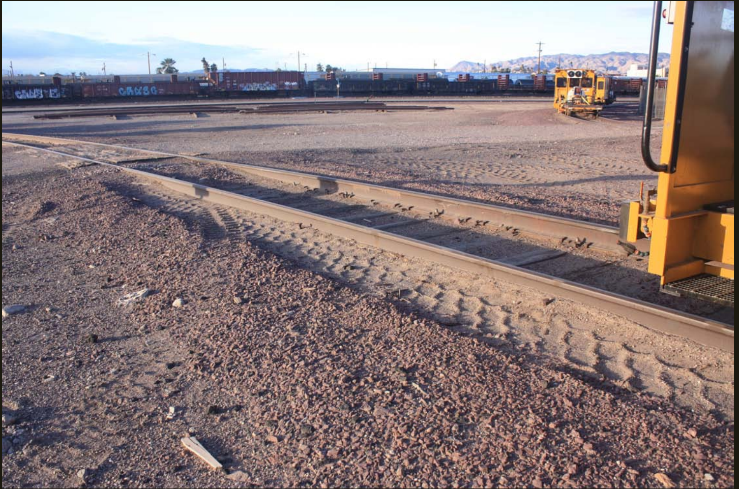
Northwestward view east of the Needles sidings (previous photo). Note the wye with the maintenance vehicles. This wye is at or very near the location of the original 1883 A&P alignment across the Colorado River.
