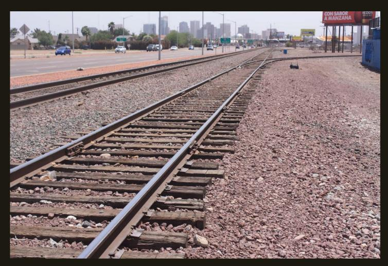
Southeastward view of the SFP&P (1895), same location as previous. The track in the foreground is a siding with industrial spurs; note the bolted rails compared to the welded track of the mainline. Barely visible in the distance, the track makes a 45° turn to the right to head due south. That is the point at which, in 1895, the SFP&P reached the outskirts of Phoenix, with its north-south east-west streets that needed to be followed into town. The downtown Phoenix skyline is in the distance.
