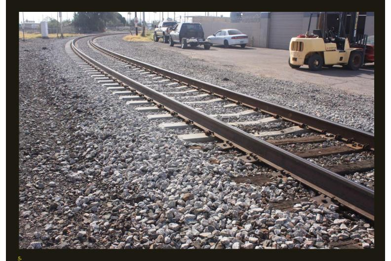
Southeastward view of the P&E (1904) where it makes a  $90^{\circ}$  turn to the right. The curve was recently upgraded, with new ballast and concrete ties.
