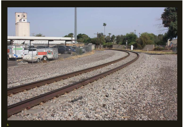
Northwestward view of the west branch of the P&E (1904) wye, showing the same grain elevator and upgraded ties and ballast as before.
