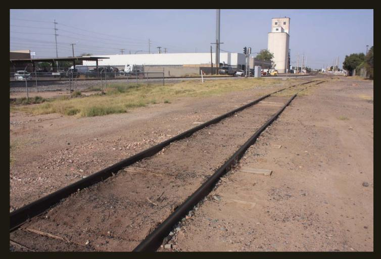
Westward view of the P&E (1904); the southward curve with new ballast is in the distance and an old straight track is in the foreground. The curved track was once the west branch of a wye, with the old track in the foreground as the "mainline." The east branch of the wye, present on the 1914-1915 topo map, has been removed.
