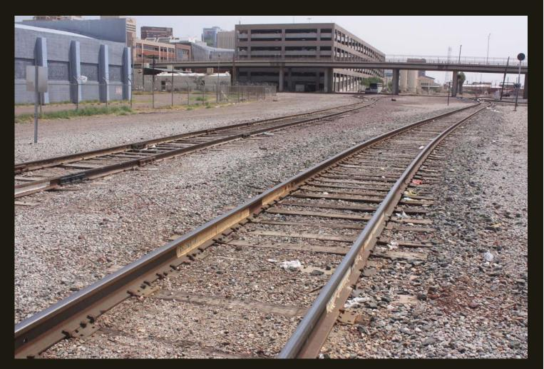
Eastward view at the same location as the previous photo. The bolted track on the left (north) is the SFP&P (1895)/AT&SF and the welded track on the right is the AE (1910)/SP. The overpass is 7th Avenue and the Phoenix Union Station is in the distance beyond the overpass.
